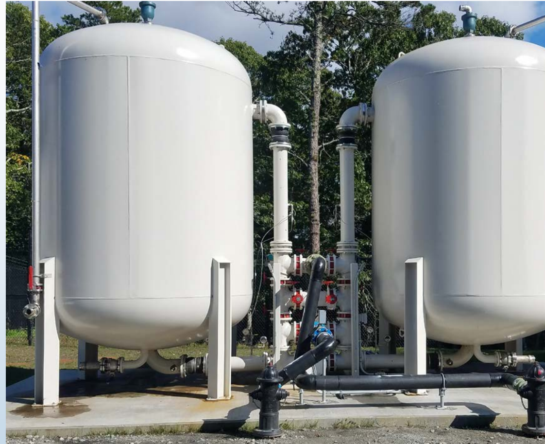
PFAS Removal Pressure Vessel Installation (Hyannis, Massachusetts)
