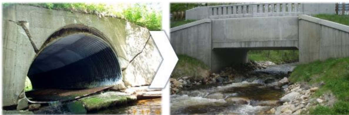
Figure 2.7 Example of Culvert Replacement
