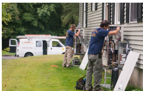
PICTURE 5B-2. INSTALLATION OF RESIDENTIAL HEAT PUMPS
