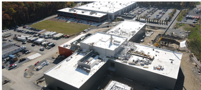
CFS' commercial fusion energy campus in Devens
