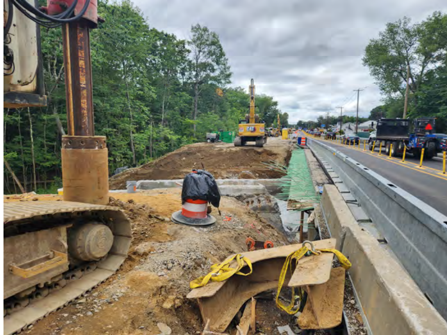
Pile Driving and Abutment Demolition Little River Bridge – Stage 2
