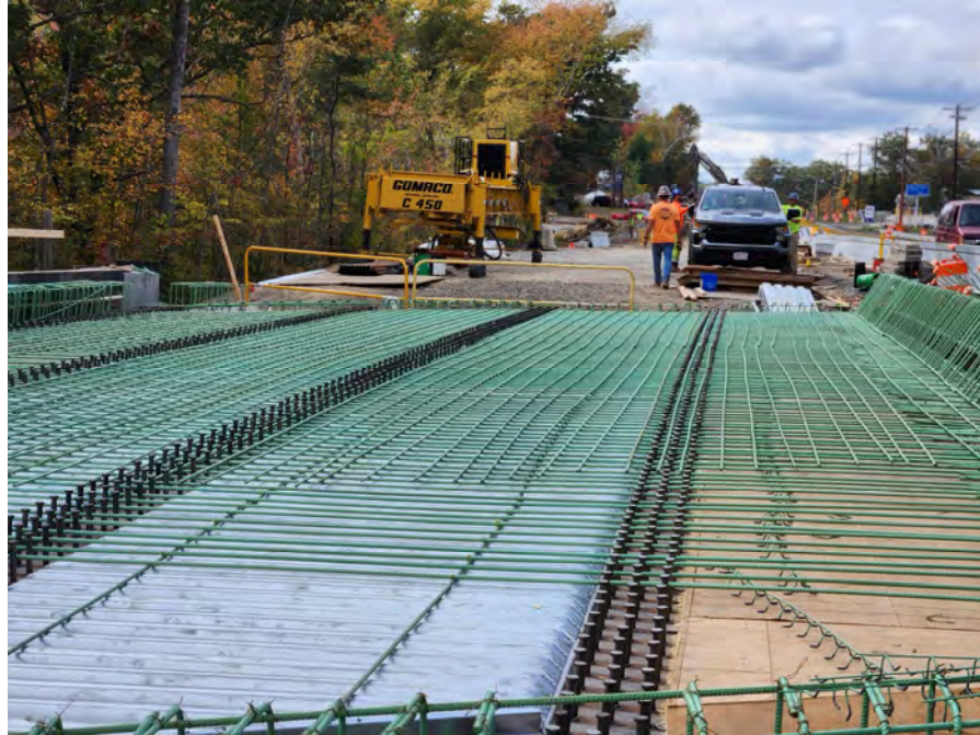
Little River Bridge Deck Reinforcement and Formwork – Stage 2
