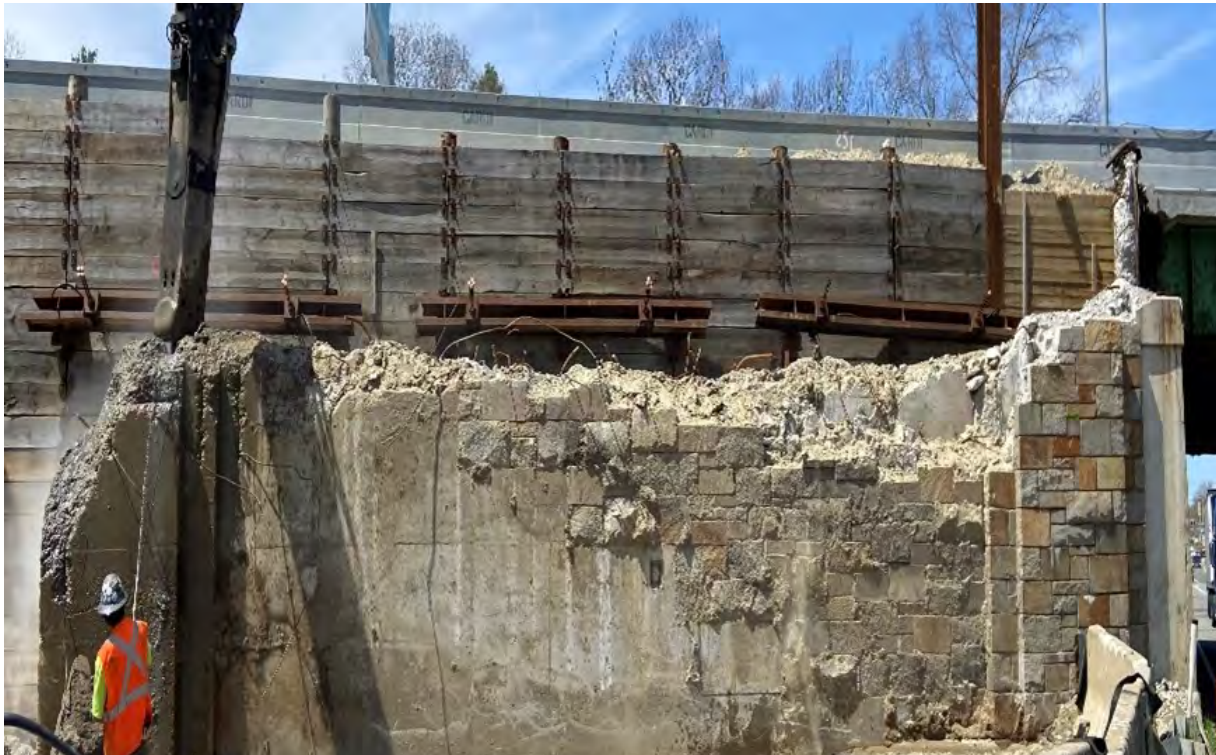
Abutment Demolition at Bridge T-01-046
