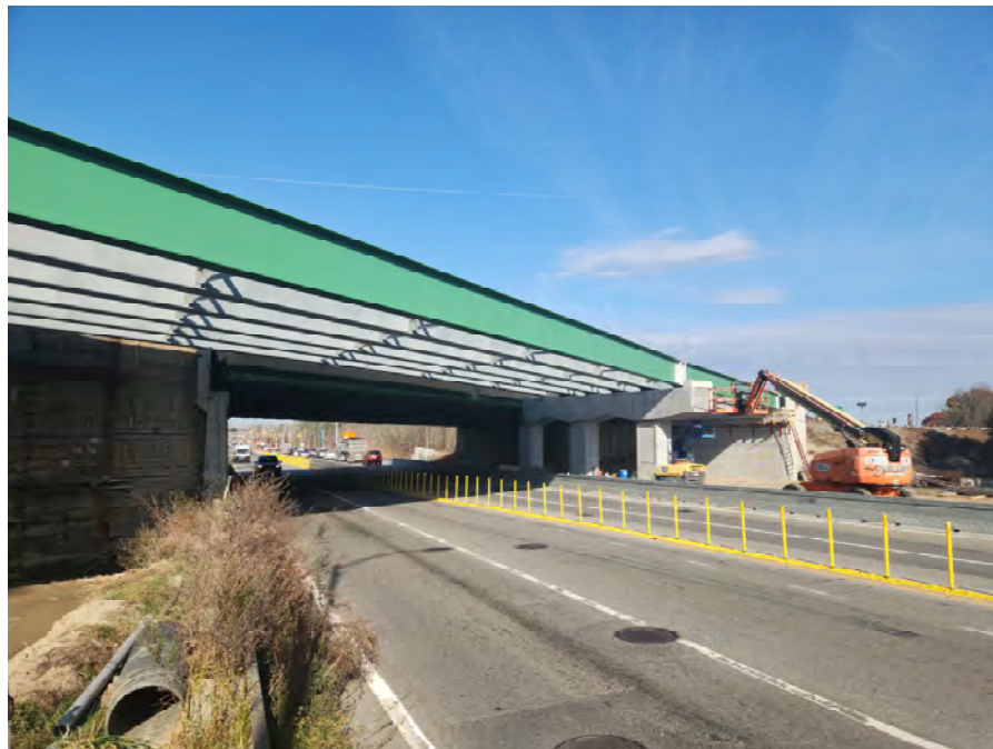
Girders Placed Across Route 140 at Bridge T-01-046
