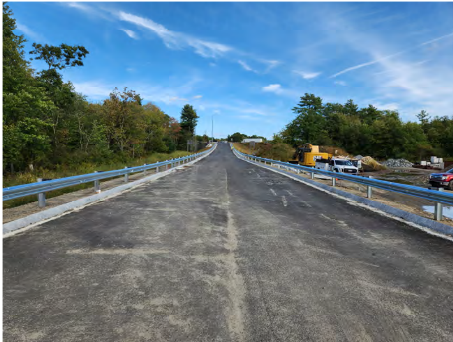
Ramp F Pavement, Granite Edging and Guard Rail
