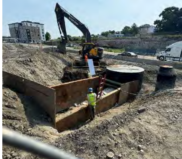
Drainage MH 09-11 upstream of new City Pier outfall June 2024
