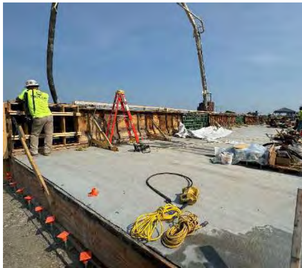
March casting CF-PL3 bridge barrier on F-02-087 June 2024
