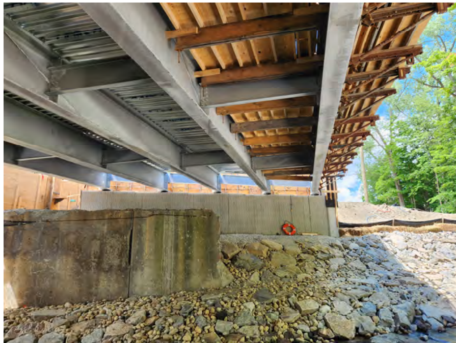
Little River Bridge Girders – Stage 1
