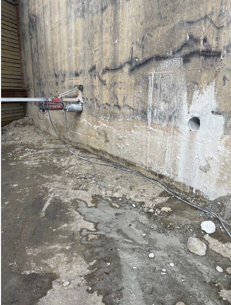
Removal of Asbestos Weepholes at Bridge T-01-045
