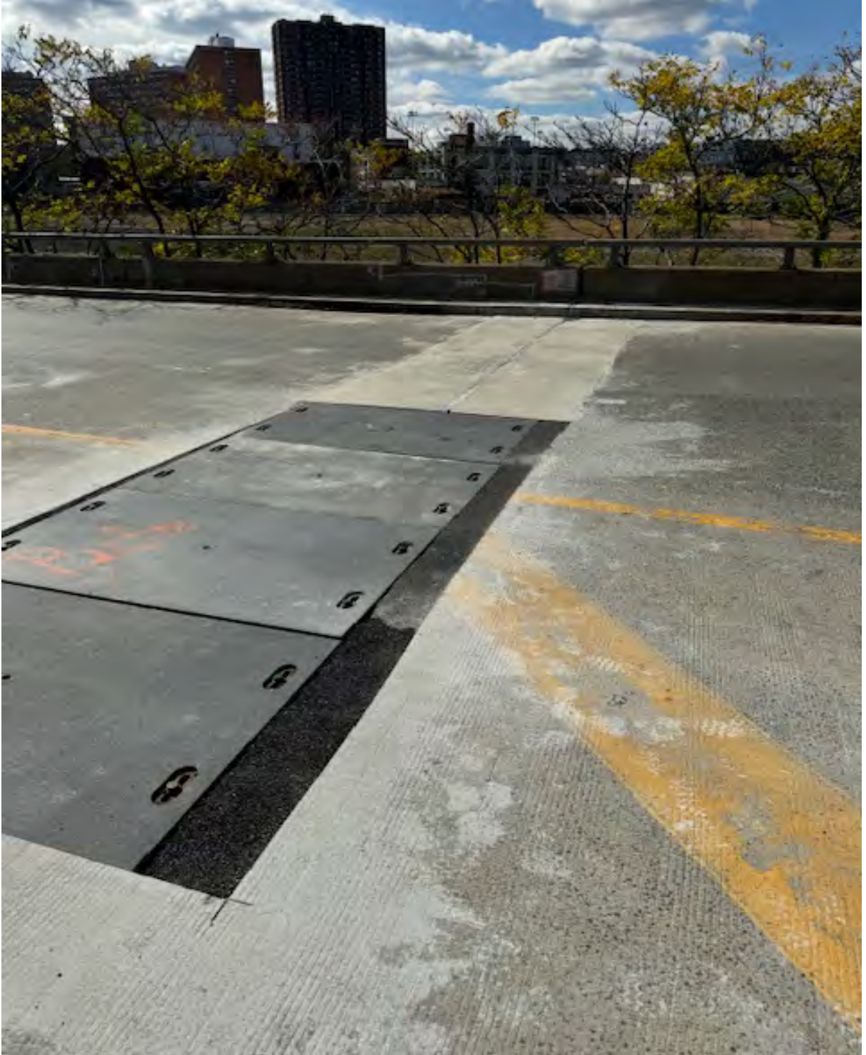
Roadway joint being repaired on Ramp D (onramp to I-90 Eastbound)
