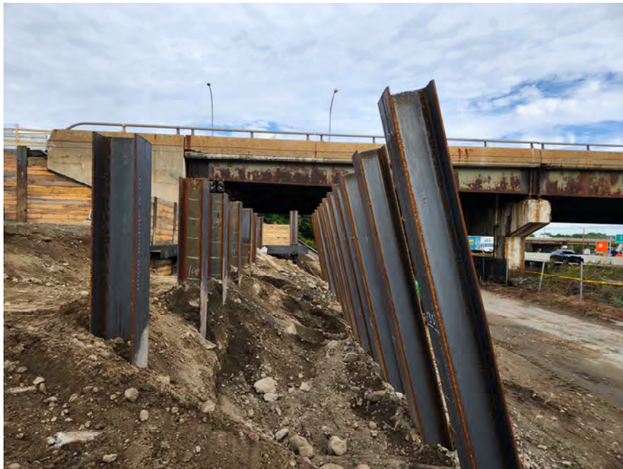
West Abutment Pile Layout
