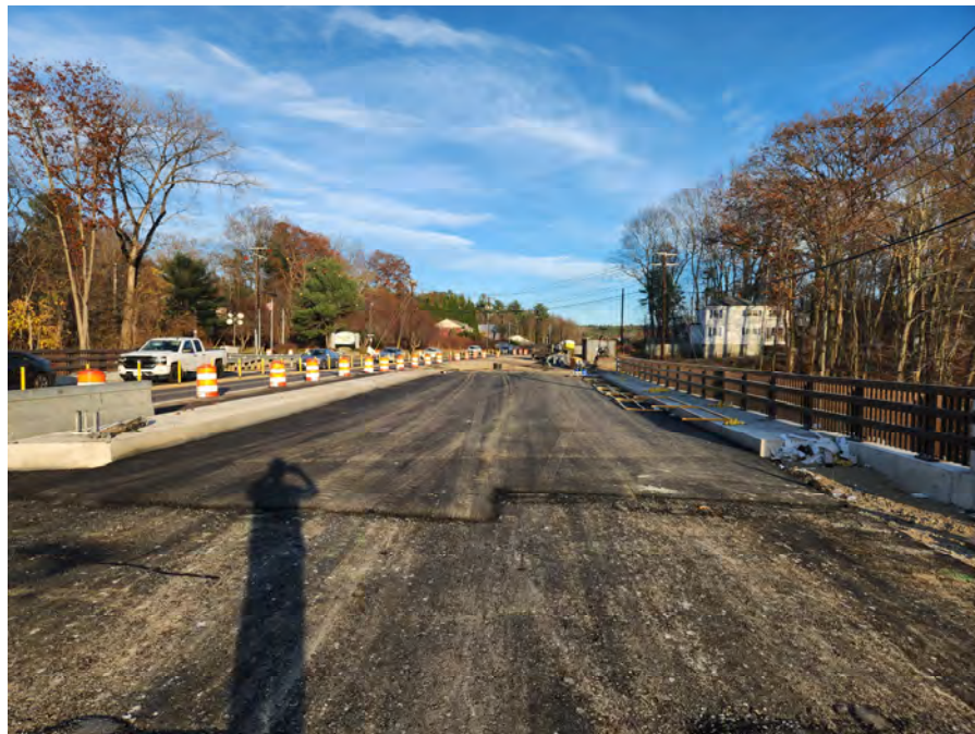
French River Bridge Deck Paved and Railing Installed – Stage 2
