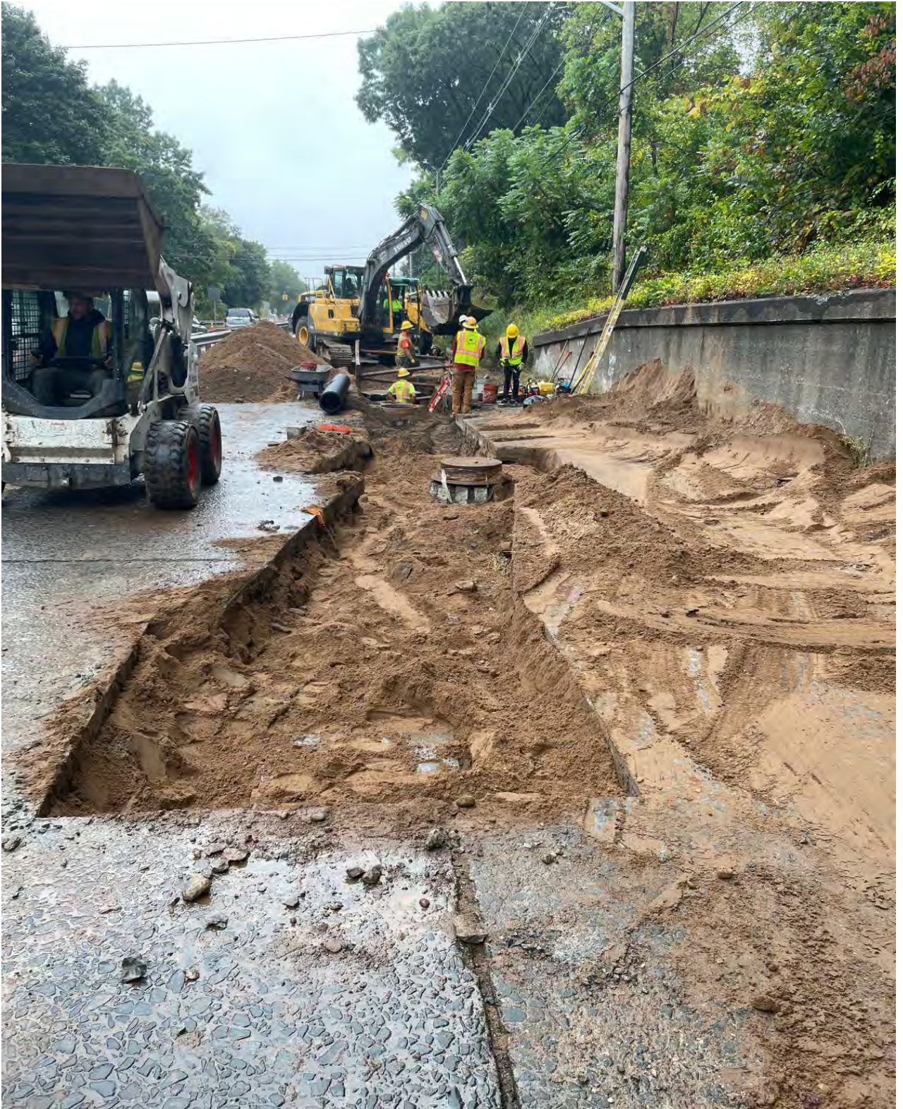
New Drainage Placement
