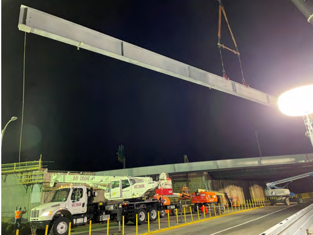
Installation of Girders at Bridge T-01-046
