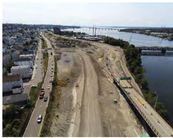
Looking south from VMB off-ramp, Davol St. NB under construction September 2024
