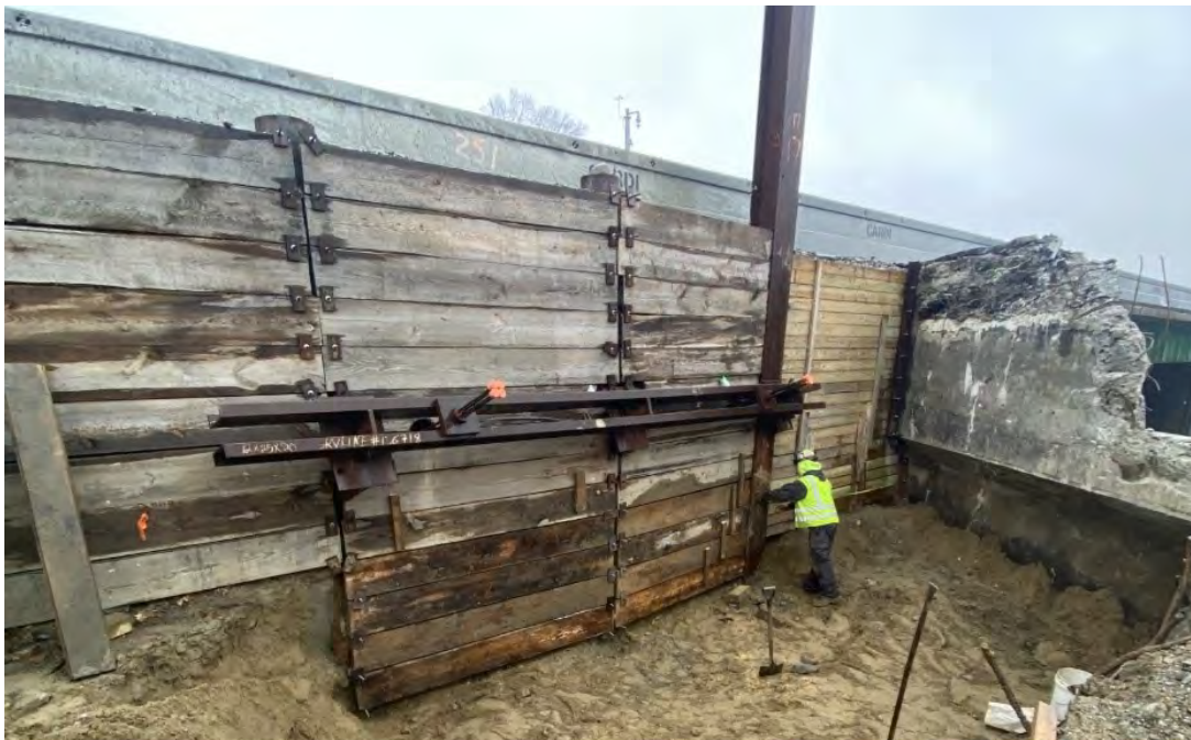
Upper Level SOE at Bridge T-01-046
