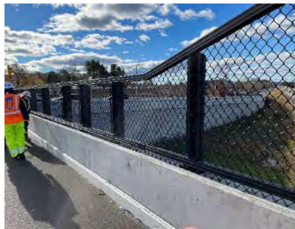
Snow fence at Wall #14 with new off-ramp in background November 2024
