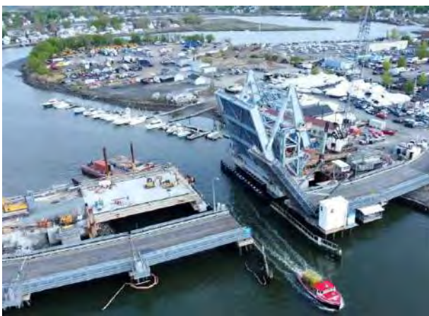
Bridge opening May 2024
