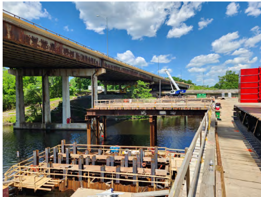
Pier 2 Cofferdam and Piles
