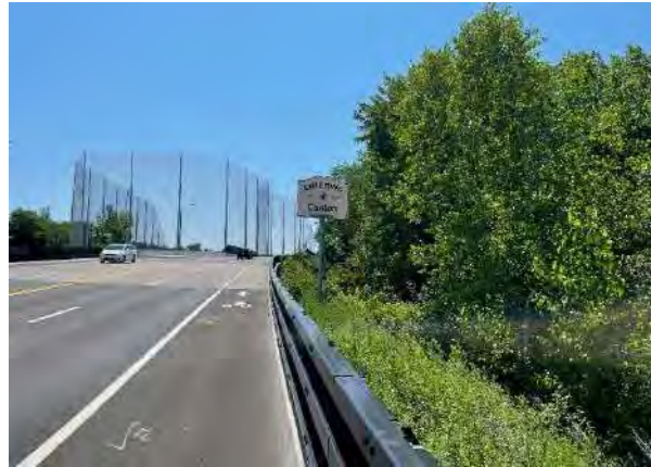
Dedham St. looking east over the Neponset River Bridge June 2024
