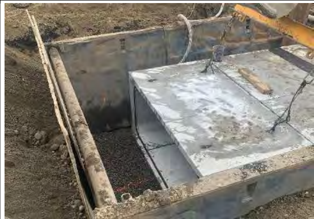
12' x 5' drainage culvert between City Pier and Davol St. NB January 2024
