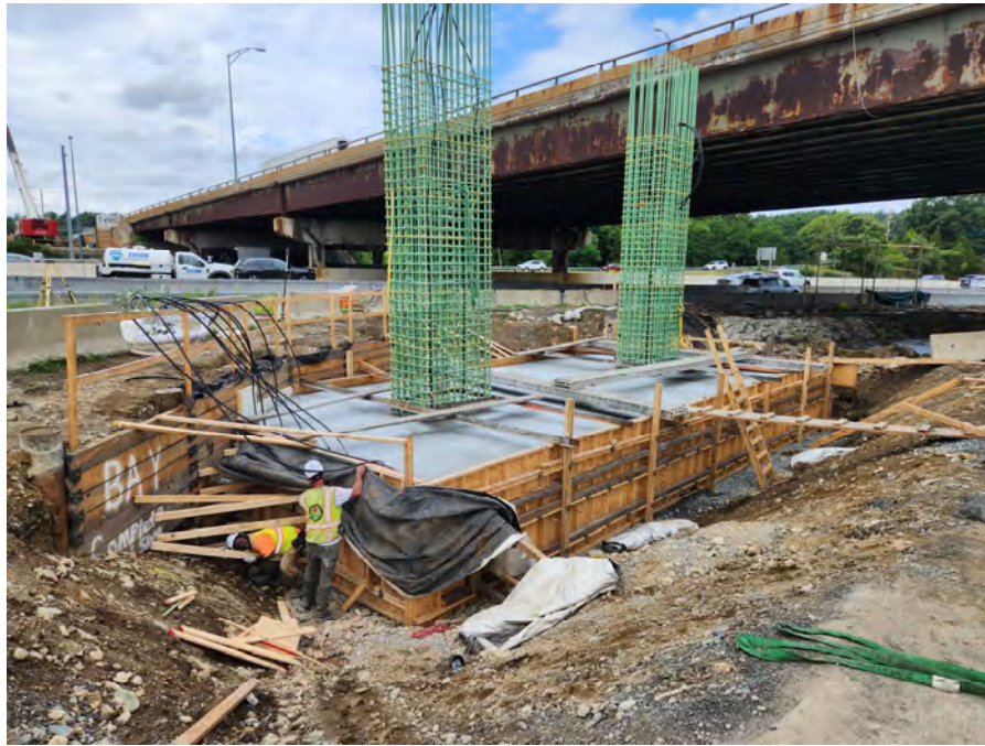
Pier 1 Footing and Column Reinforcement
