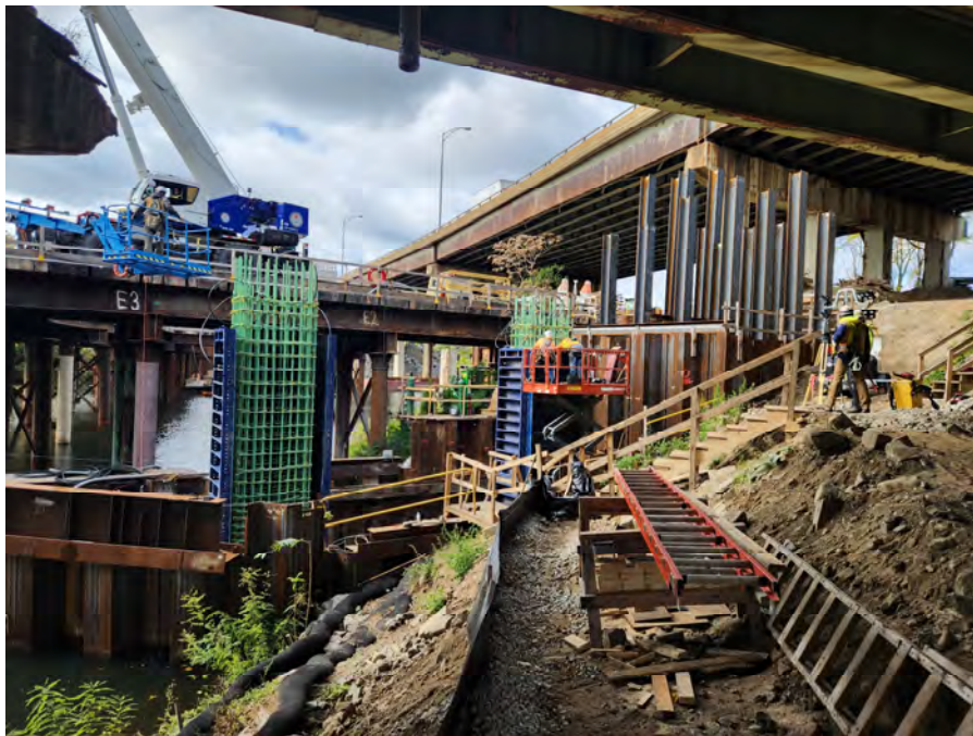
Pier 3 Column Reinforcement and Formwork
