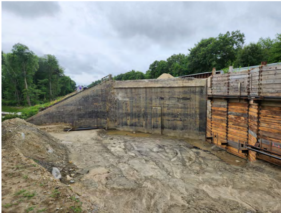
Level 2 SOE Installed at Bridge T-01-045
