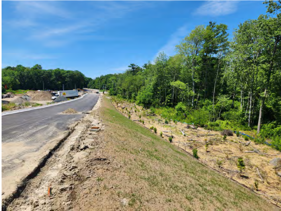
Ramp F Base Course Pavement and Wetland Mitigation
