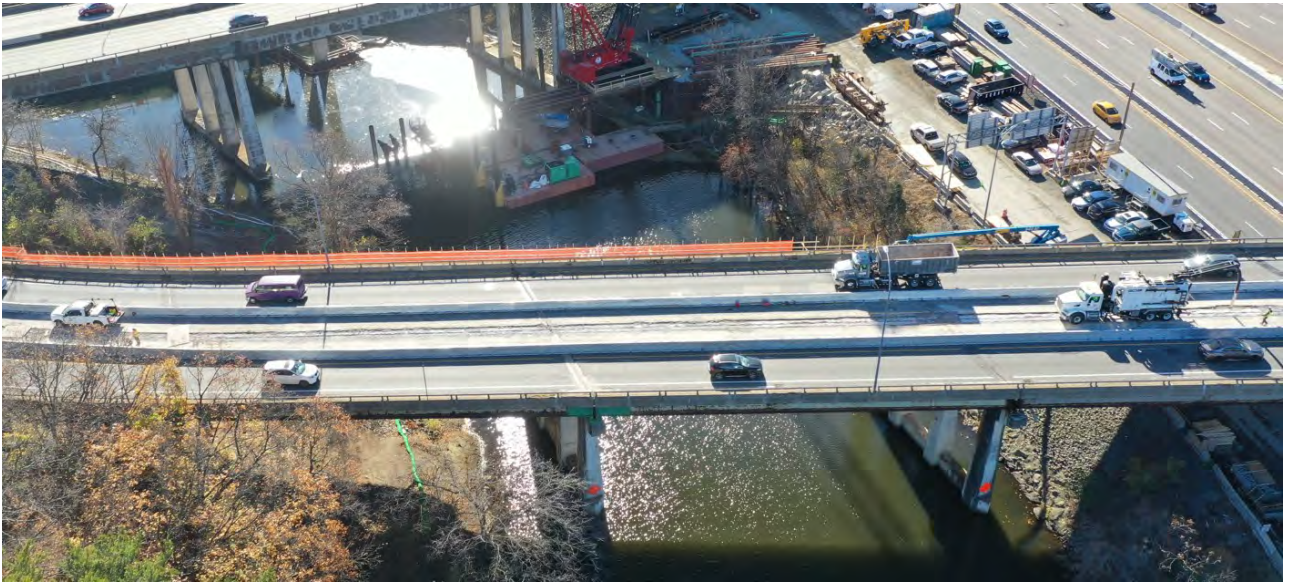
Bridge N-12-064 = W-29-034 Raised Median Removal
