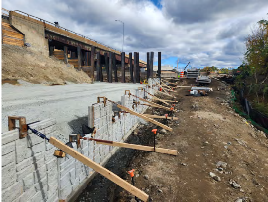
Wall 17 at West Abutment
