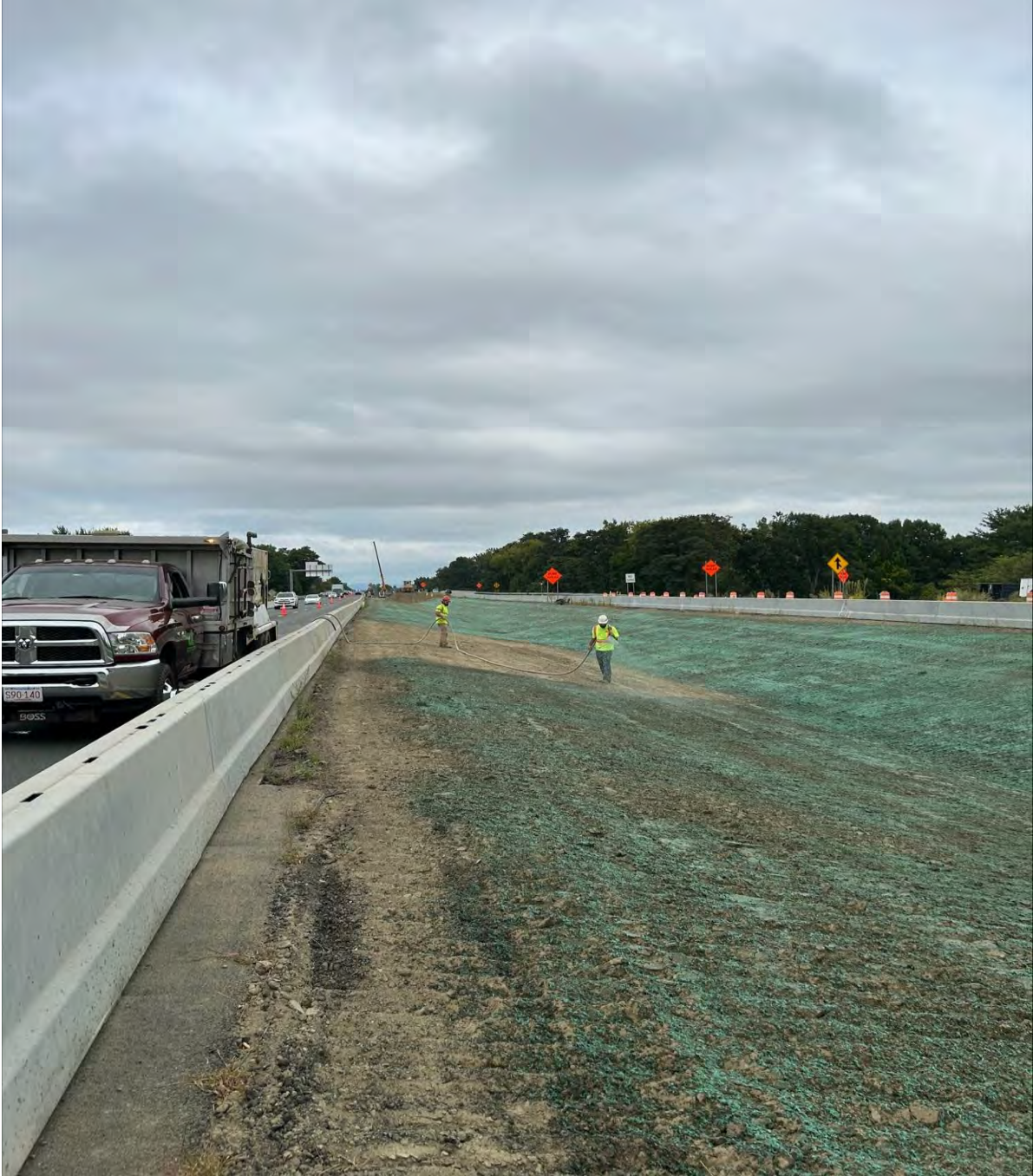
Hydroseeding Restored Median Area
