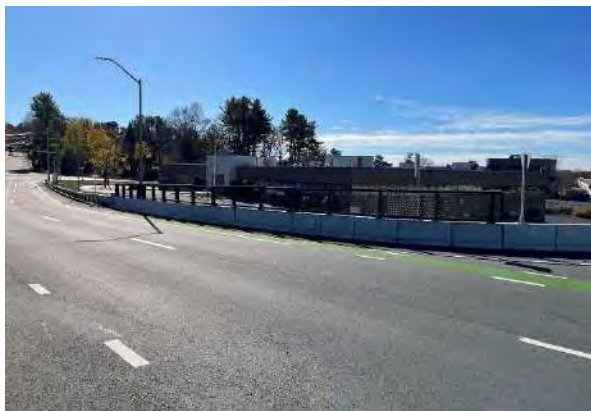
Snow fence complete at Wall #13, looking east November 2024
