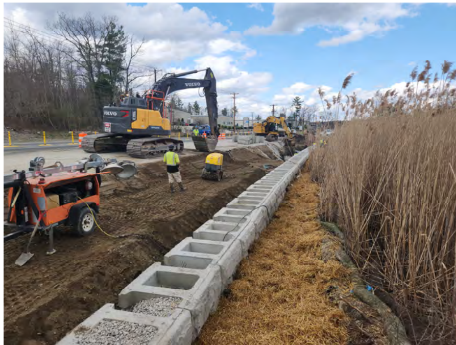
Wall H Construction
