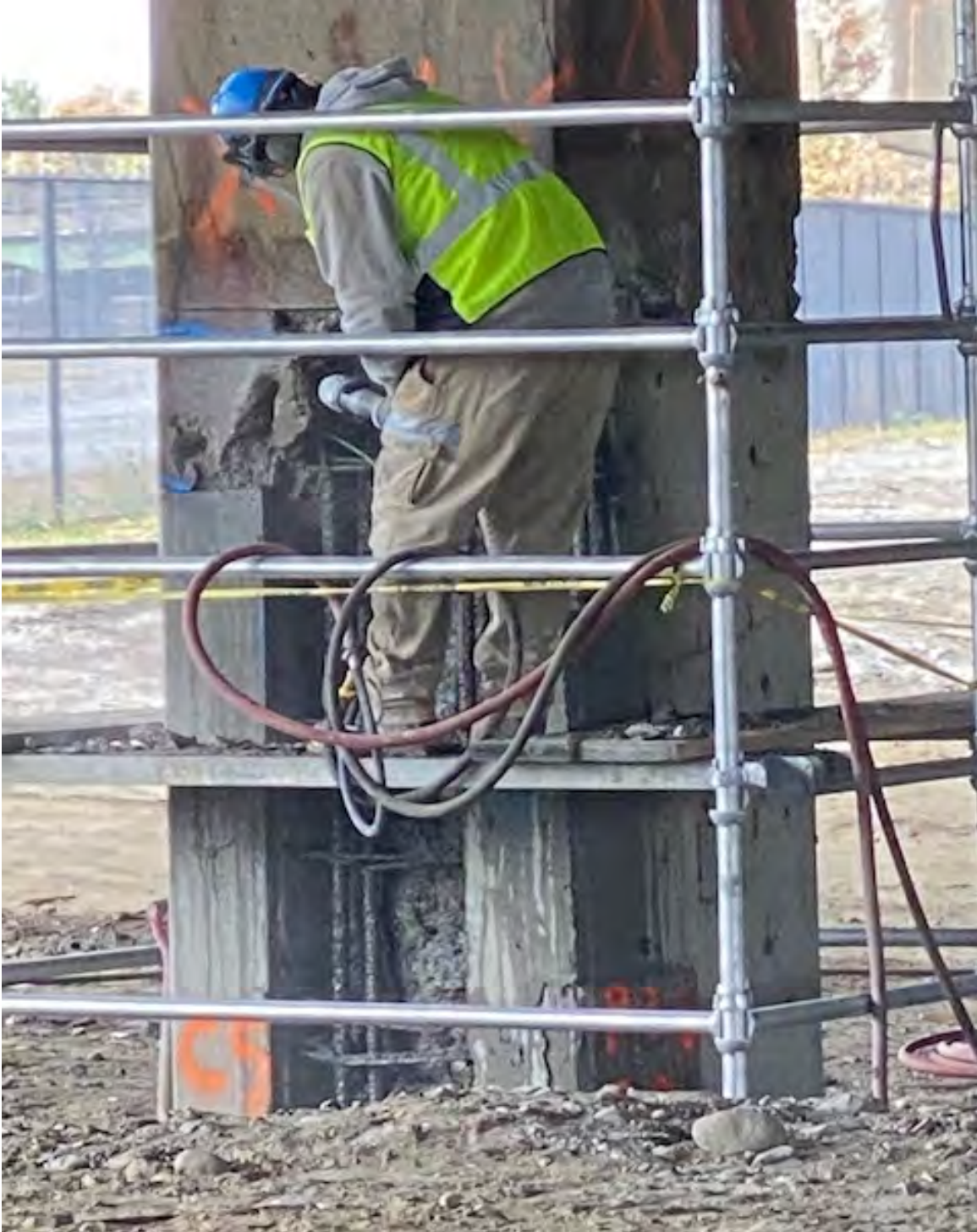
Demolition of unsound concrete
