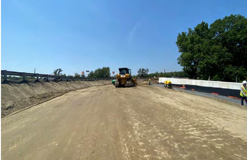
Ramp E Subgrade adjacent to Wall 4
