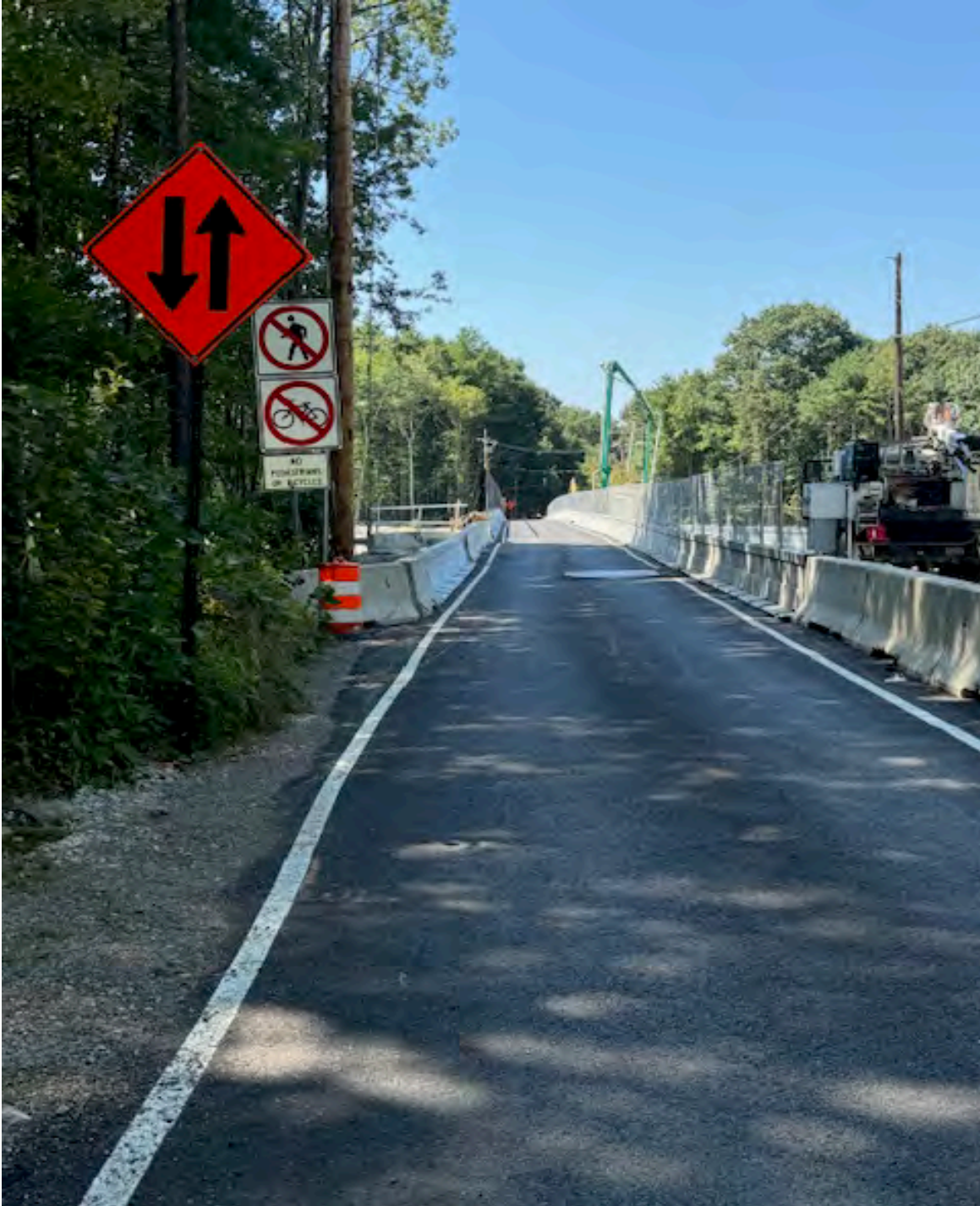
South half of Fruit Street bridge now open to traffic
