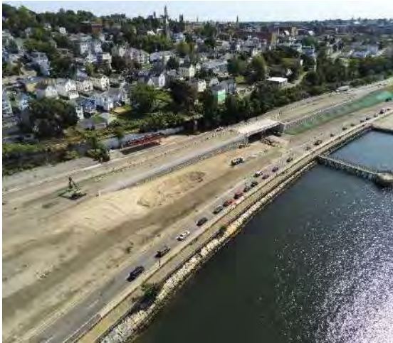
Overview of F-02-087 and modular approach walls September 2024
