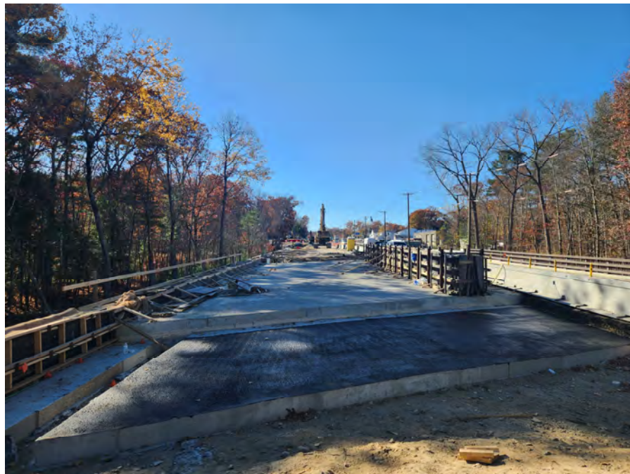
Little River Bridge Deck and Median Barrier Formwork – Stage 2
