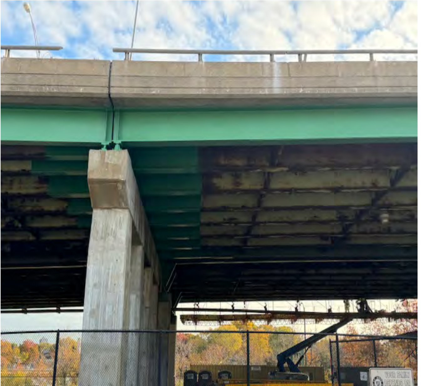
Typical conditions post repair work
