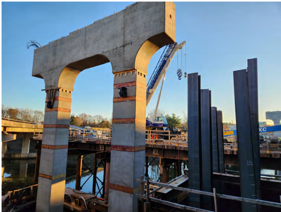
Pier 3 with Formwork Removed
