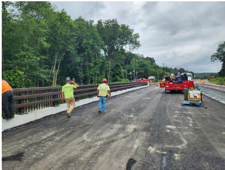
French River Bridge Deck Paved and Railings Installed – Stage 1
