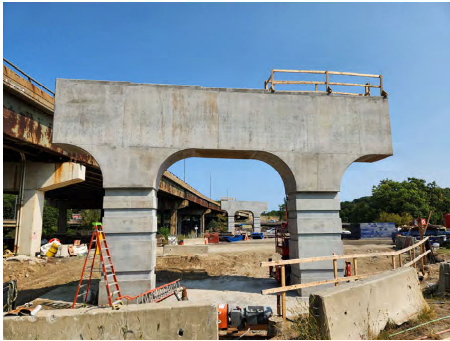
Piers 1 and 2 with Formwork Removed
