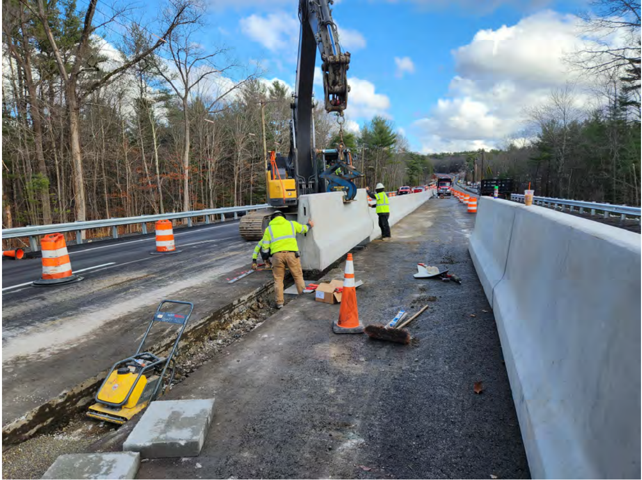
Median Barrier Installation
