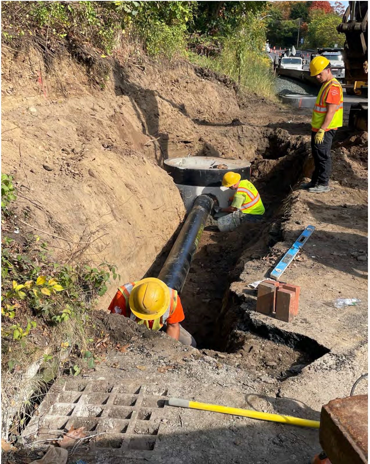
New Drainage Placement
