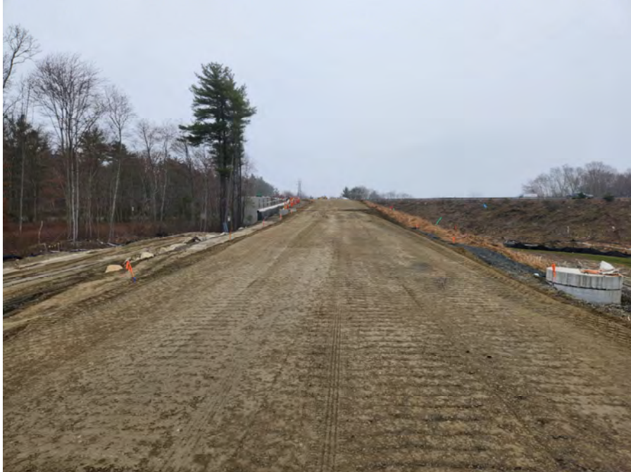
Ramp F Subgrade Preparation
