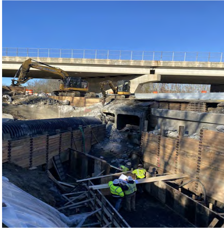
Temporary SOE and Formwork for Abutment Footing at T-01-054 Culvert Extension
