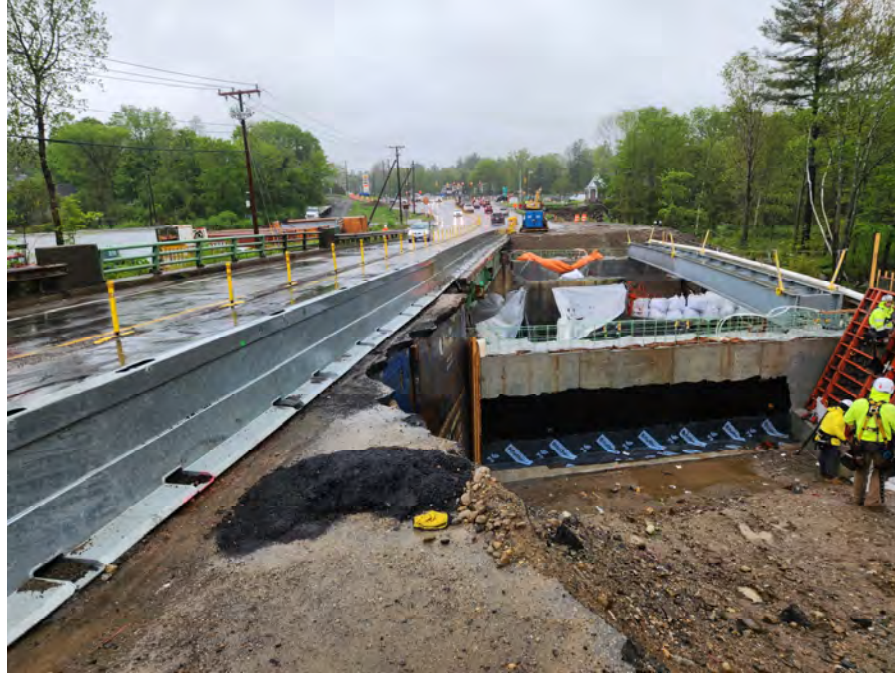
French River Bridge Abutment Construction Stage 1
