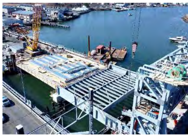
Span 1 SIPs, moveable span floor beams and stringers March 2024
