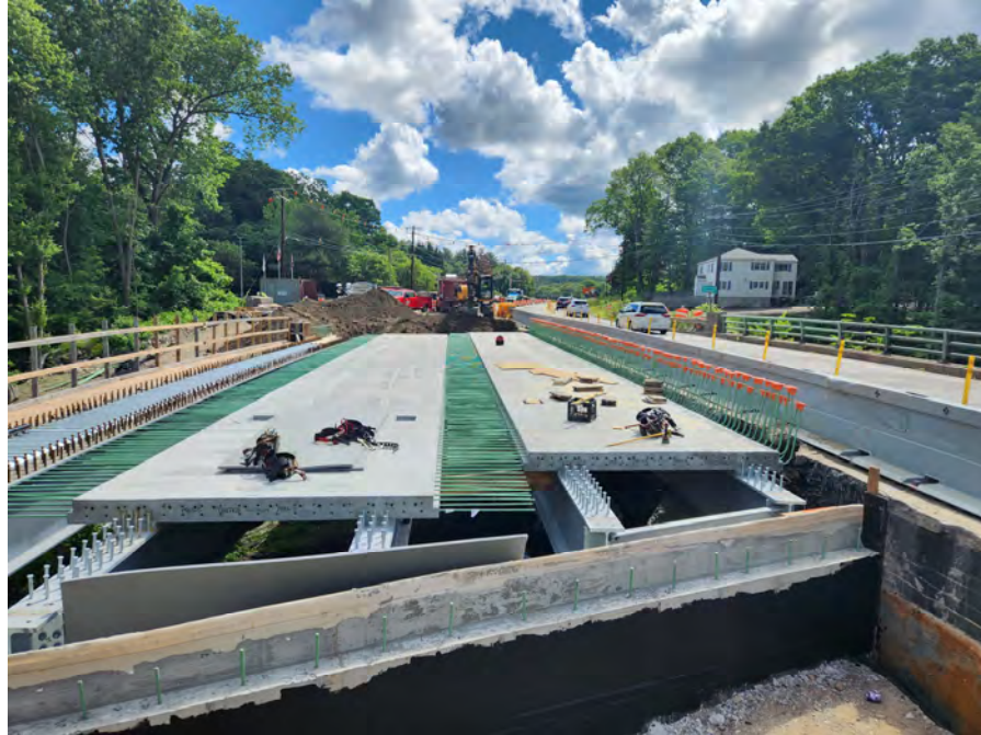
Precast Bridge Units Installed French River Bridge Stage 1
