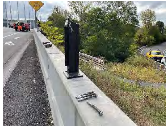
Snow fence post October 2024
