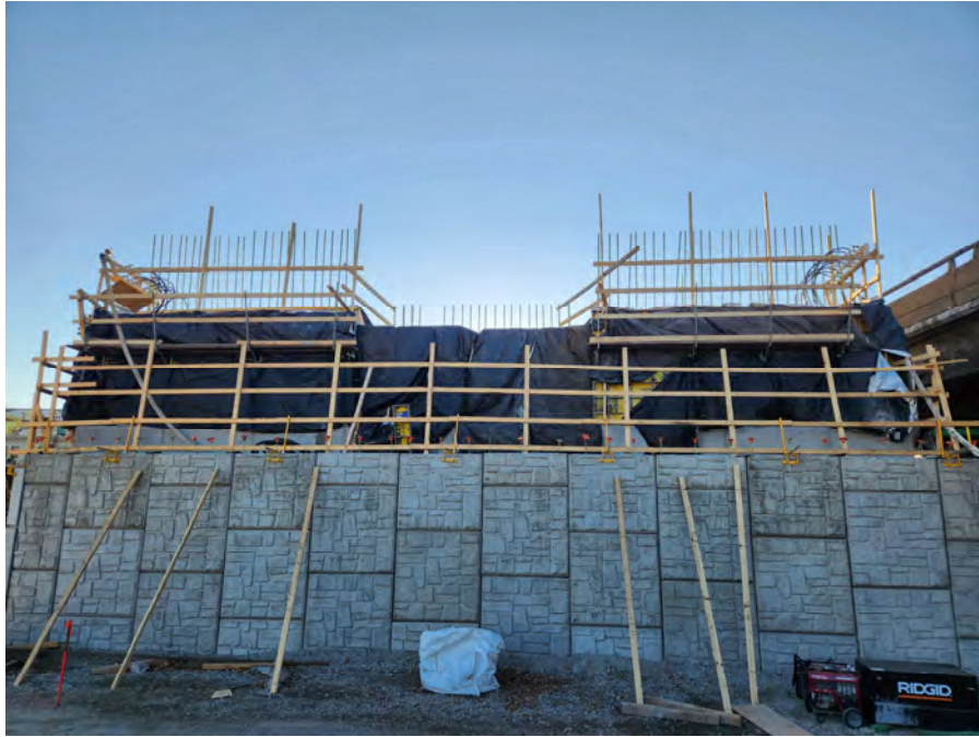
West Abutment Stem and MSE Wall
