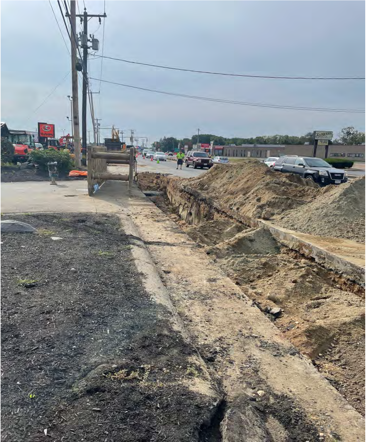
New Waterline Placed Under Existing Concrete Pavement
