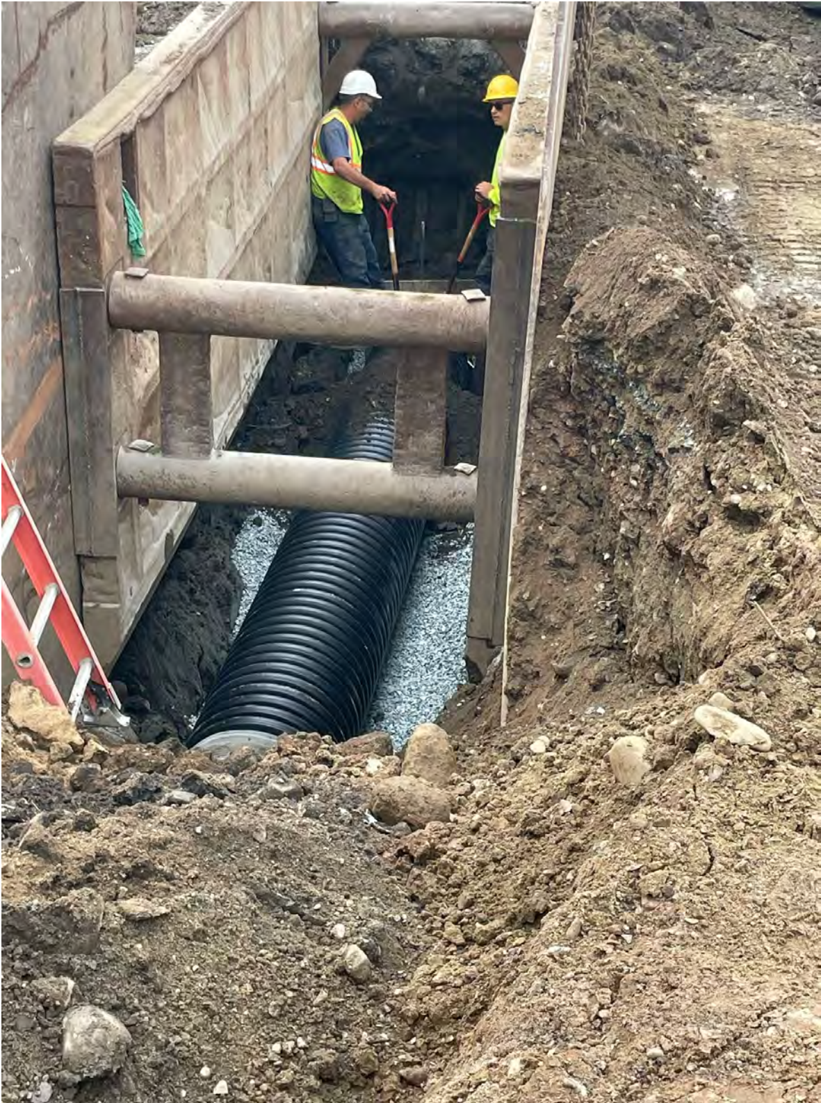
New Drainage Placement
