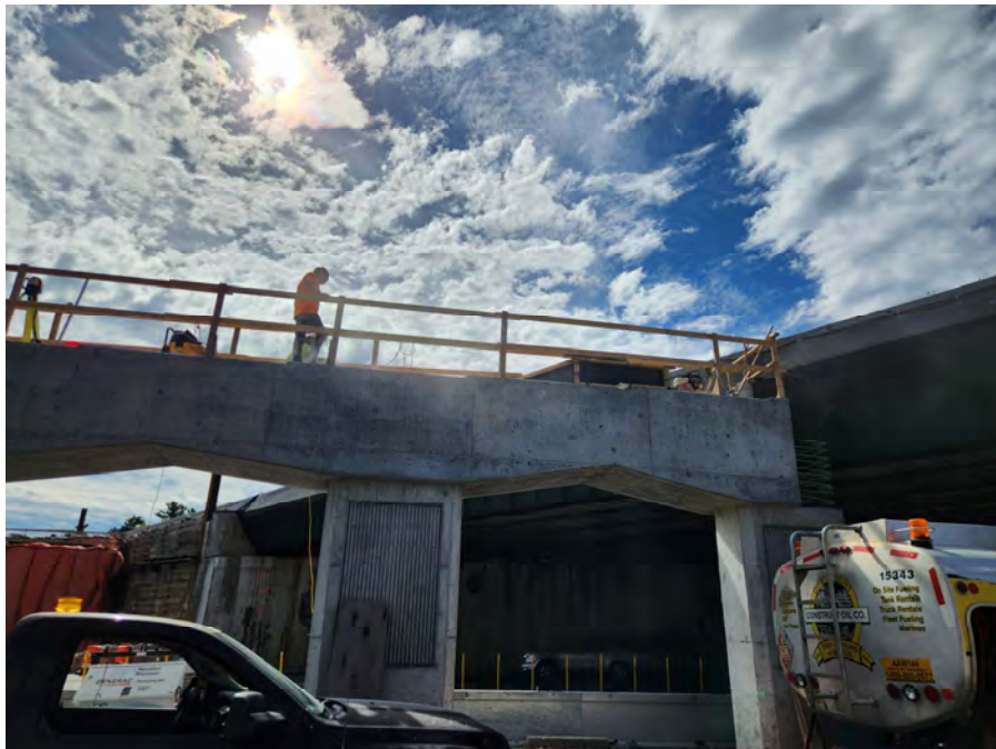
Center Pier at T-01-046 Beam Seat Preparation
