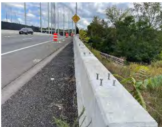
Attachment bolts in place October 2024
