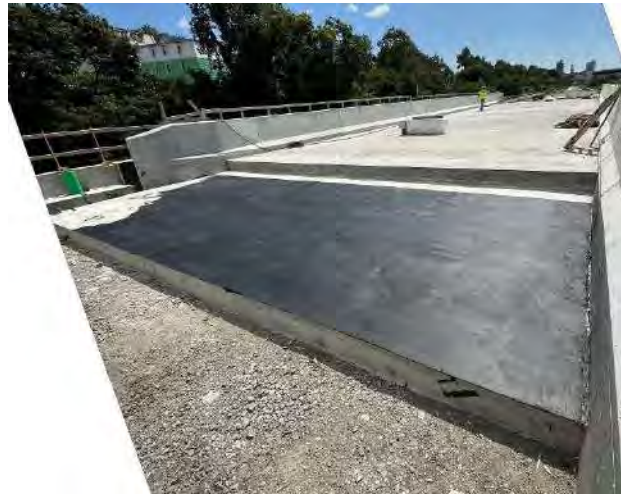
F-02-087 north approach slab September 2024
