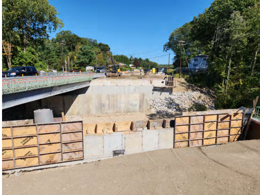
French River Bridge Backwall Formwork – Stage 2
