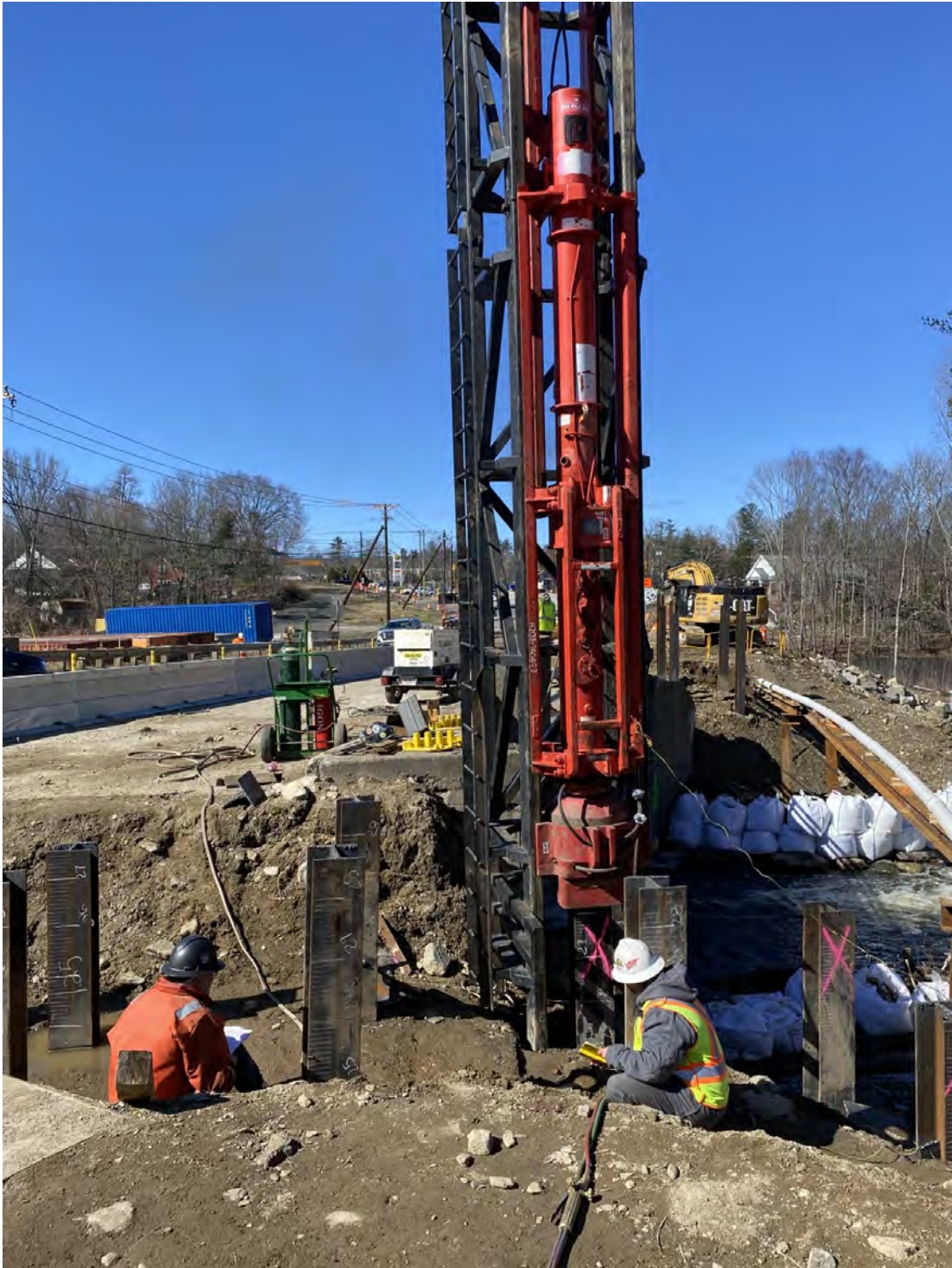
Pile Driving Operations at French River Bridge Stage 1
