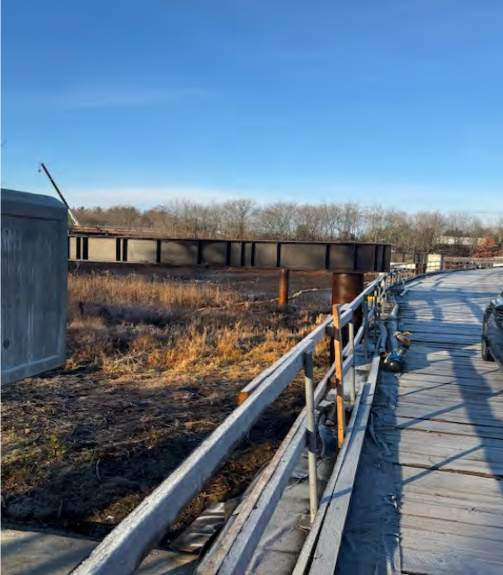
Temporary steel falsework to support tub girder erection on WN
