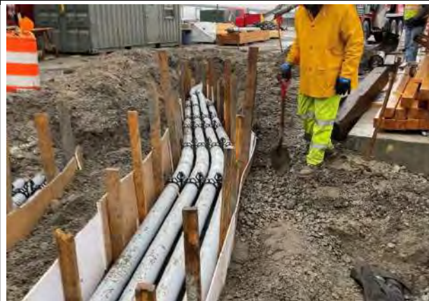
NGRID conduit under F-02-087 April 2024
