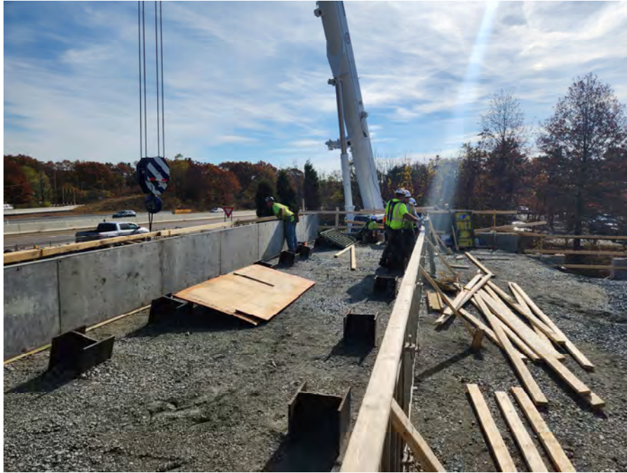
West Abutment Cap Formwork
