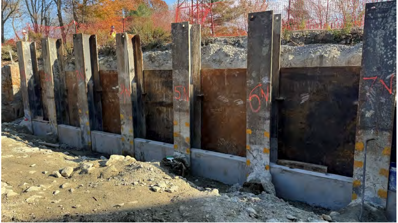
Installation of Permanent SOE at Bridge T-01-047
