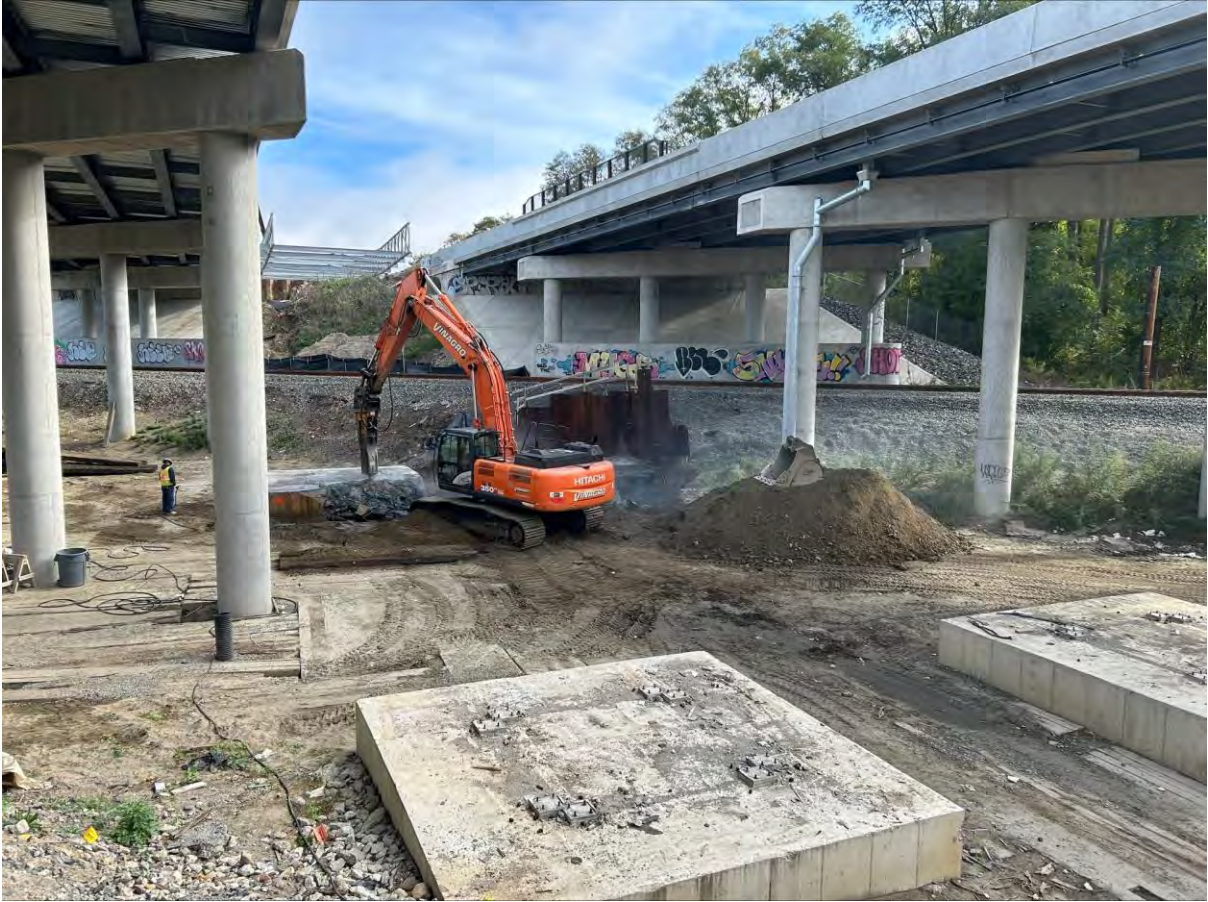
Demolition of Footings for Temporary Access Bridge
