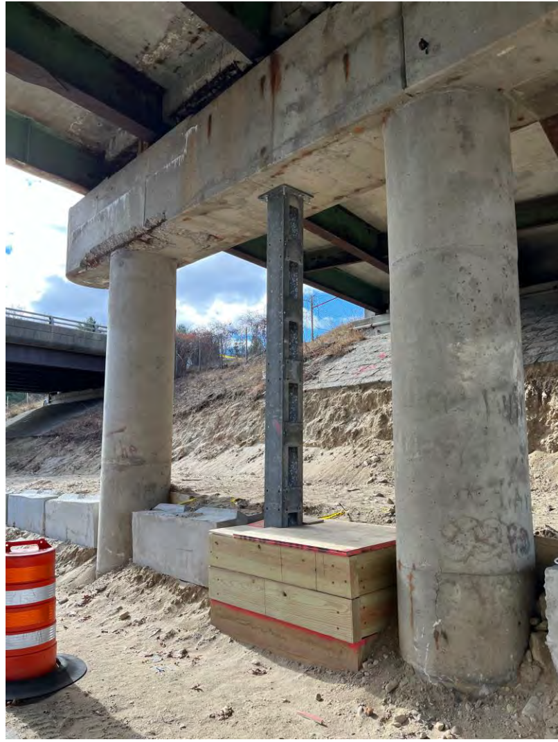
Shoring Tower Along Route 28 for I-495
