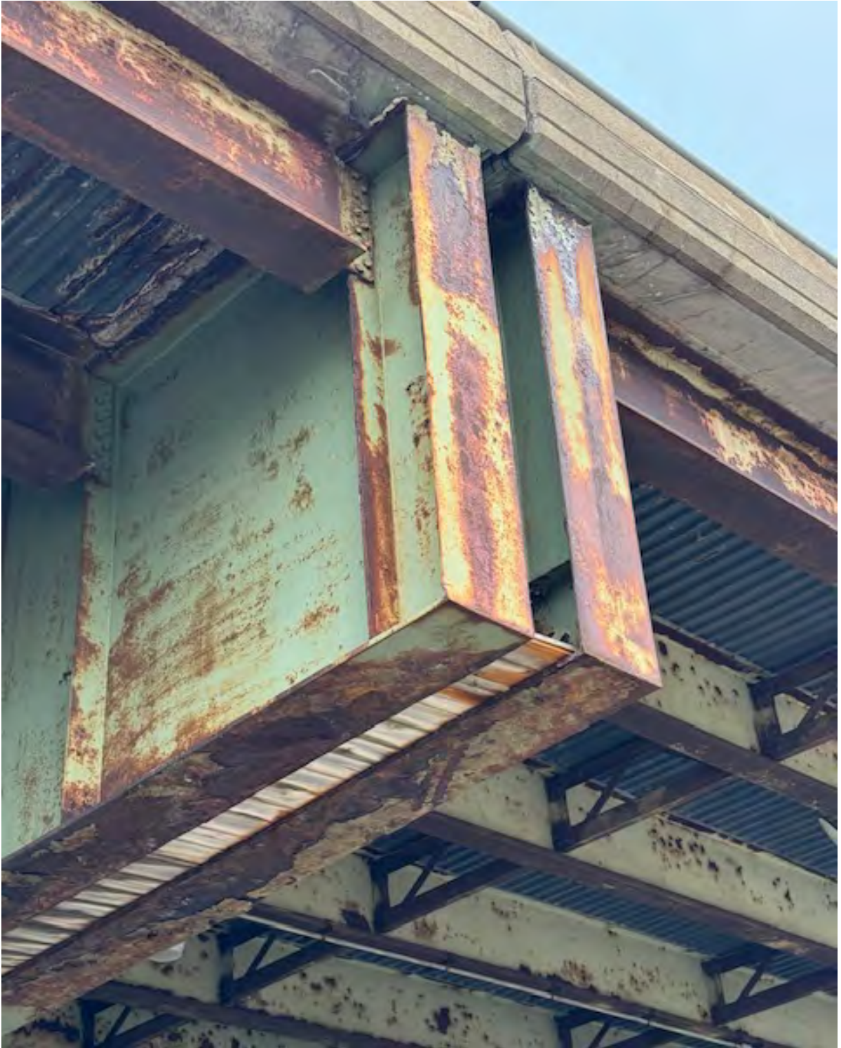
Typical condition of twin structural steel girders at pier (2023)
