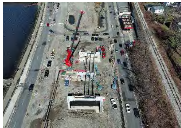
F-02-087 beam erection March 2024
