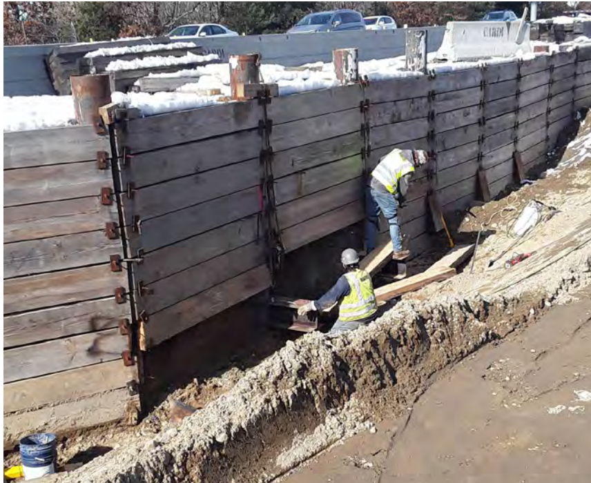
Upper Level Support of Excavation (SOE) at Bridge T-01-045
