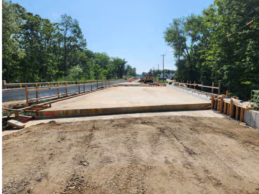
Little River Bridge Deck – Stage 1
