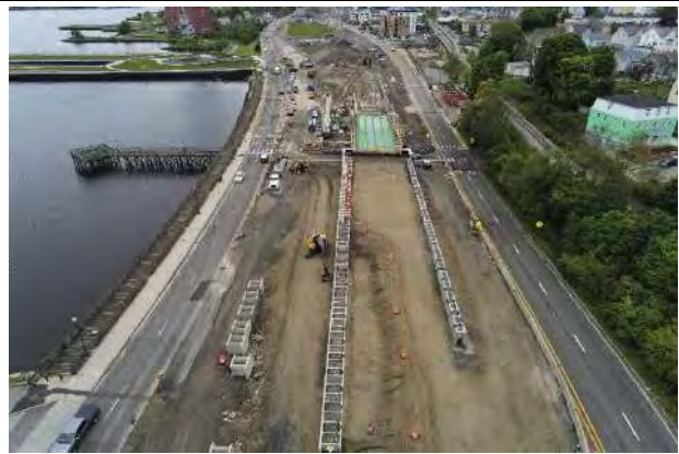
F-02-087 looking north May 2024
