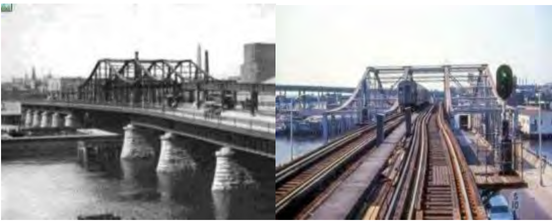
Historic North Washington Street Bridge
