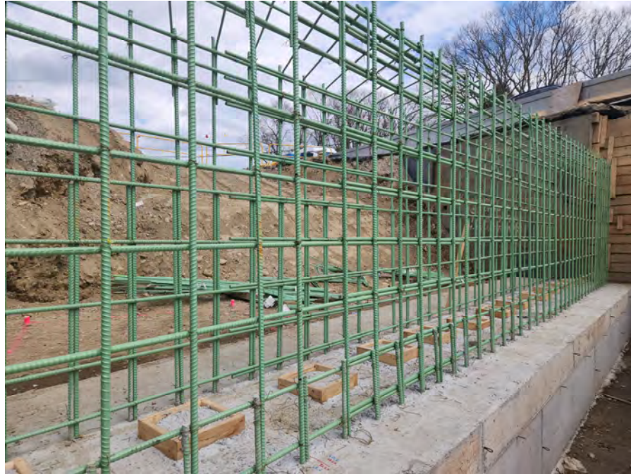
French River Bridge Abutment Stem – Stage 1
