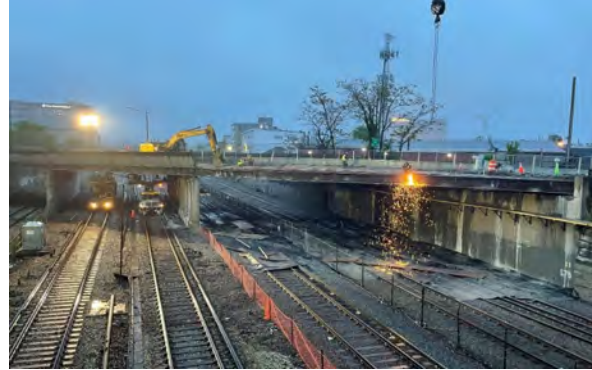
May 2024 – Mystic Avenue Demolition
