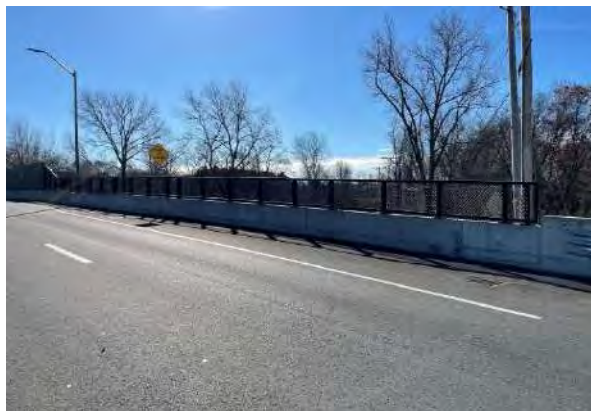
Snow fence complete at RR Bridge SW wingwall November 2024
