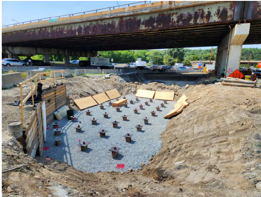
Pier 1 Micro Pile Layout
