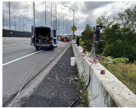
Coring for snow fence attachment bolts October 2024
