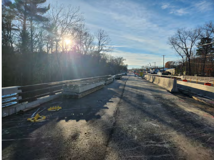
Little River Bridge Deck Paved and Railing Installed – Stage 2
