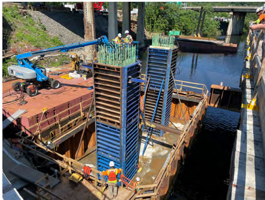
Pier 2 Column Formwork
