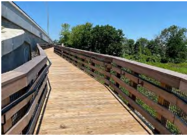
Completed handrail at pedestrian bridge C-02-050 June 2024
