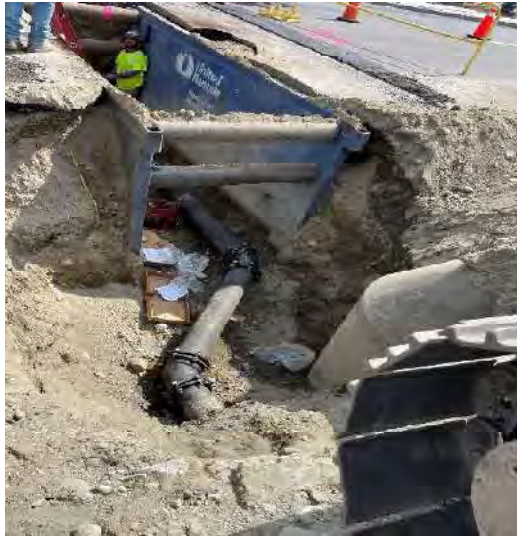
Installation of 8" lateral water main September 2024
