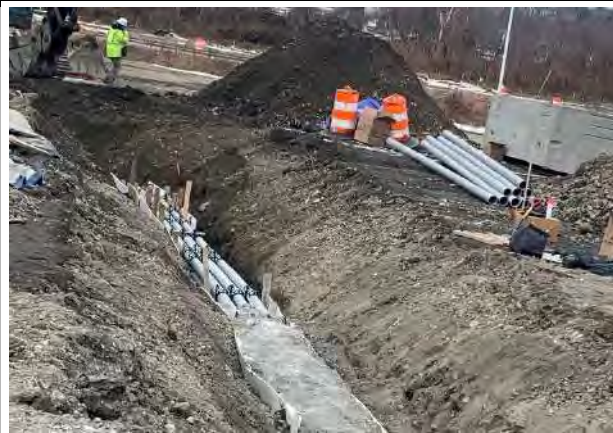
Conduit for NGRID, Brightman Street extension January 2024
