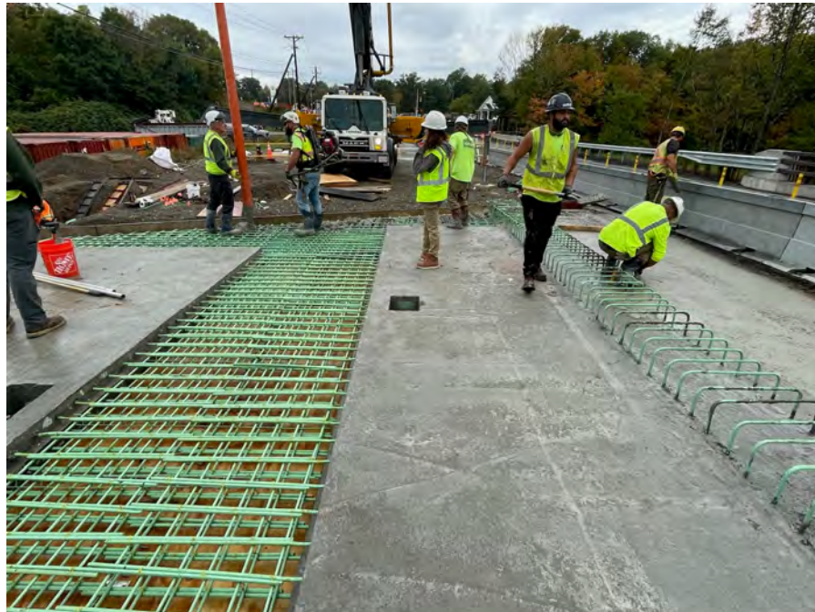
French River Bridge Deck Closure Pour – Stage 2
