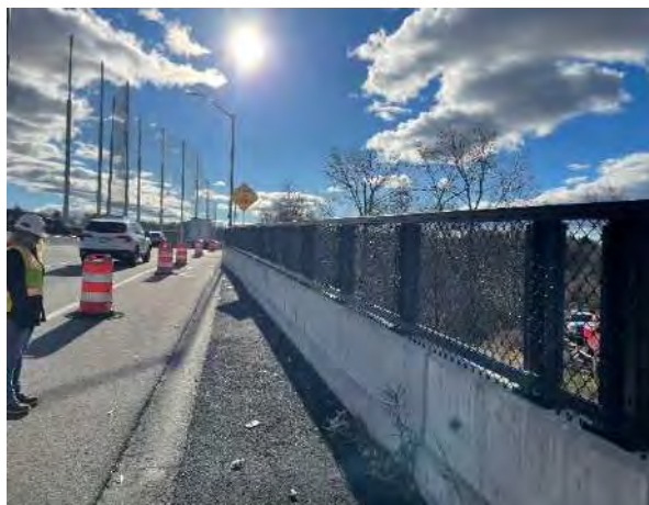
Snow fence at NW wingwall of RR Bridge November 2024
