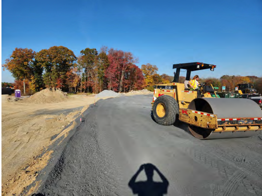
Ramp C Subbase Construction
