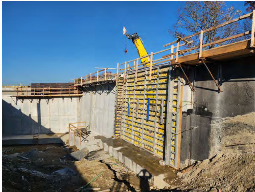
Wall 3 Closure at Bridge T-01-046 Wingwall
