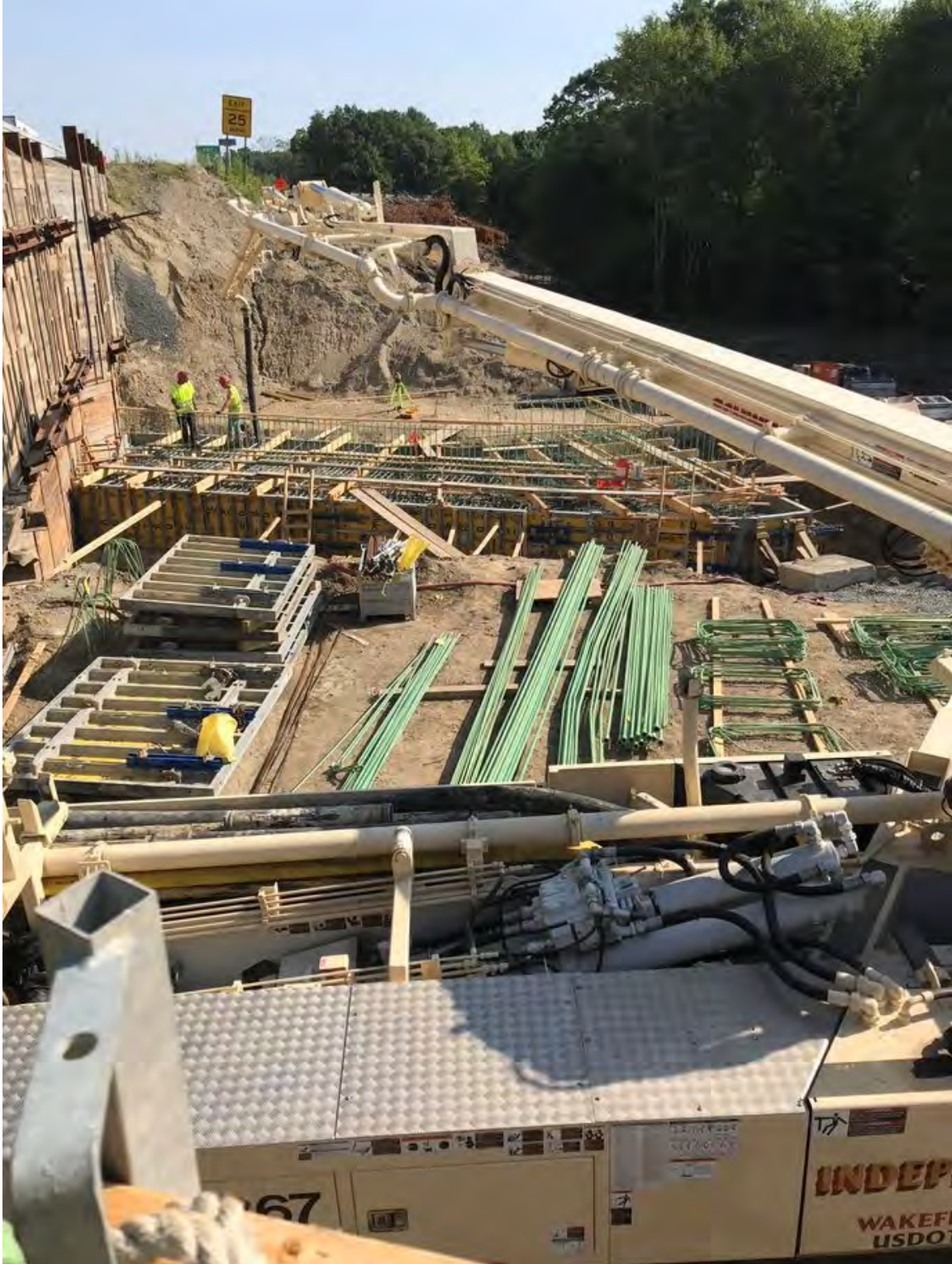
Concrete Placement at Bridge T-01-046 Abutment Footing
