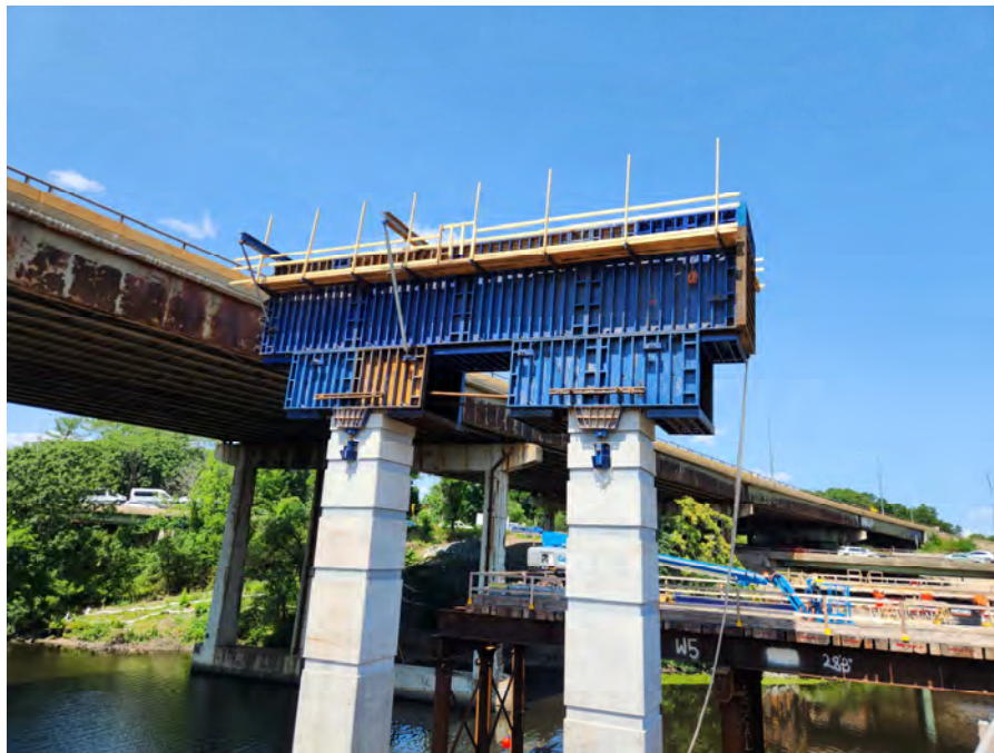
Pier 2 Cap Formwork
