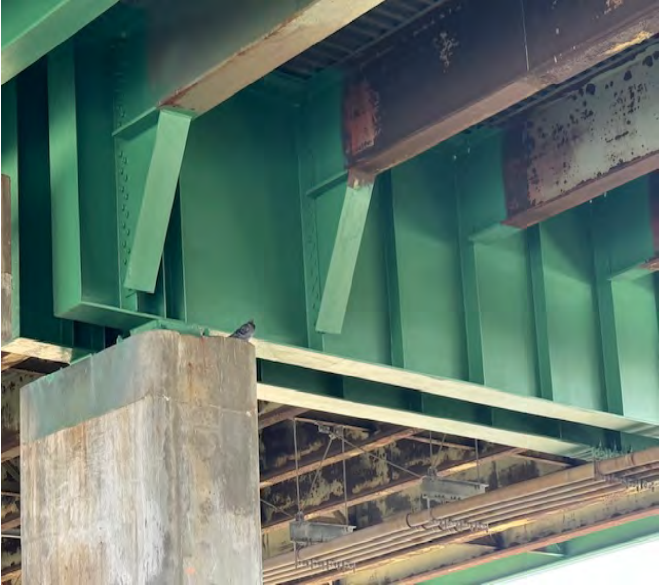
Steel girders at pier post repairs
