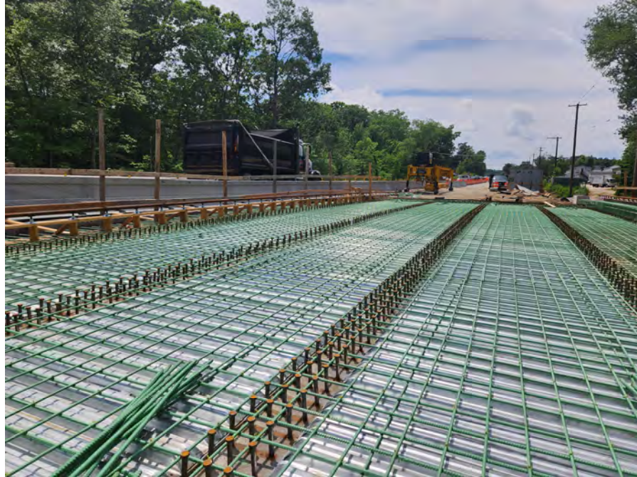
Little River Bridge Deck Formwork and Steel Reinforcement – Stage 1
