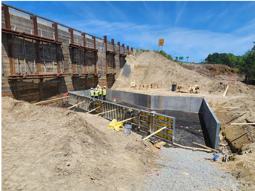
Footing Formwork at Bridge T-01-046
