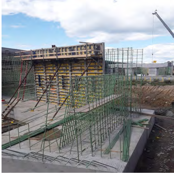
Abutment Stem Formwork and Reinforcement at Bridge T-01-046
