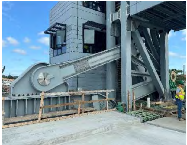
West operating strut and segmental gear August 2024
