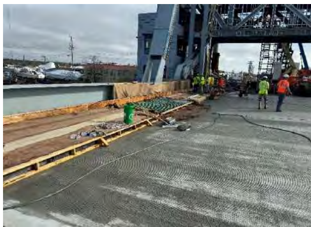
Moveable span sidewalk pours May 2024
