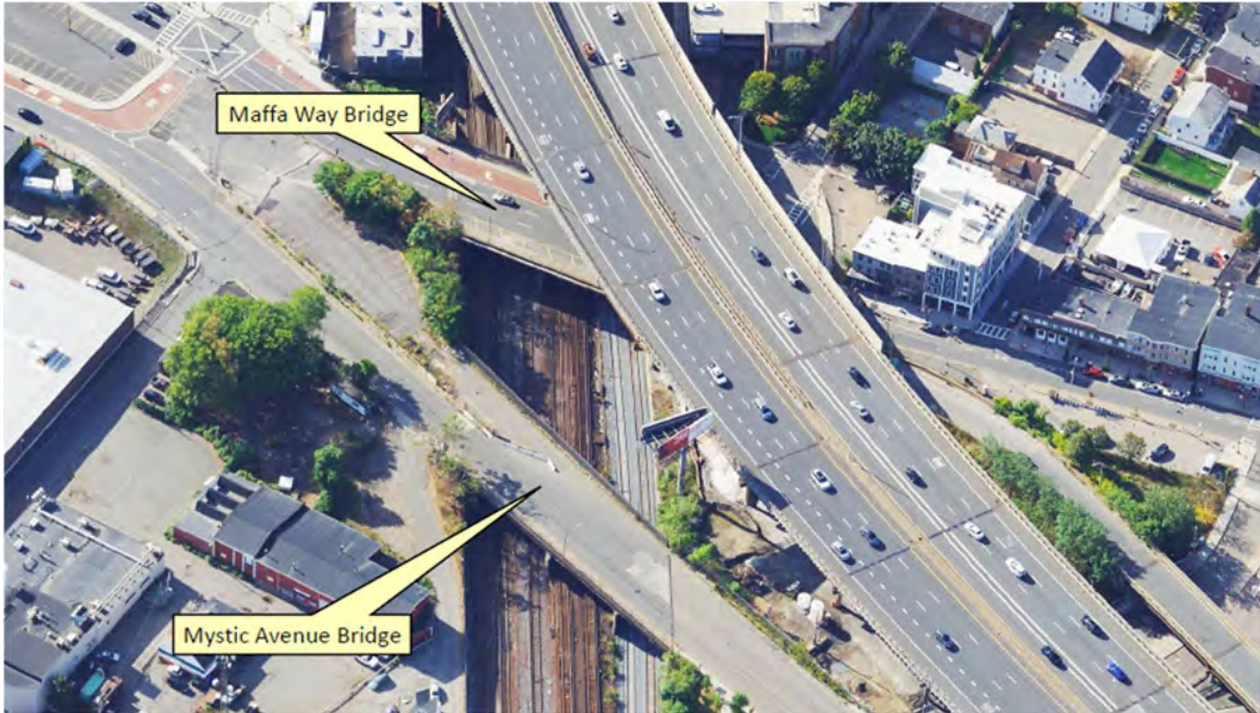
Aerial View of Project Location
