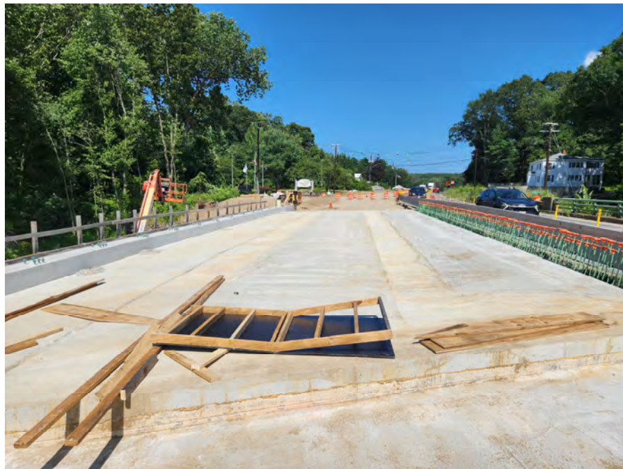
French River Bridge Stage 1 Deck with Closure Pours
