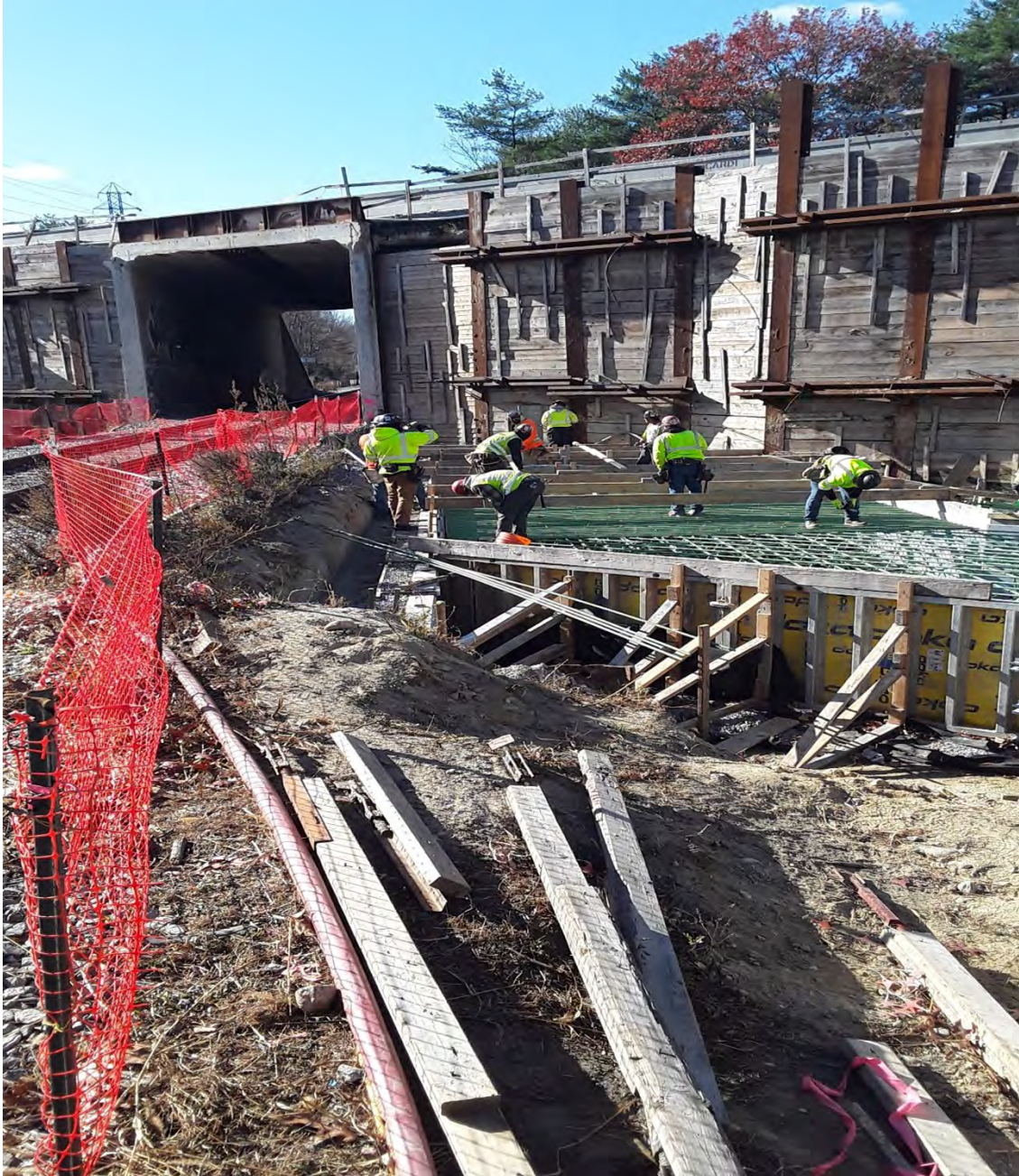
Formwork and Reinforcement for Abutment Footing at T-01-047
