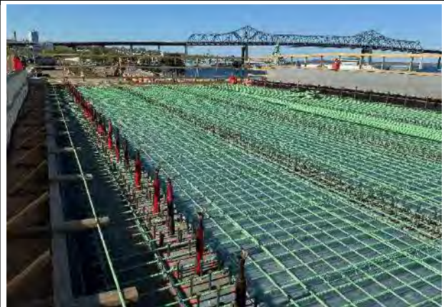
F-02-087 reinforcing steel in progress May 2024
