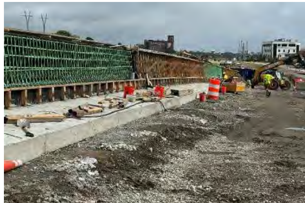
Wall D-03, NW approach CL-PL3 on moment slab August 2024
