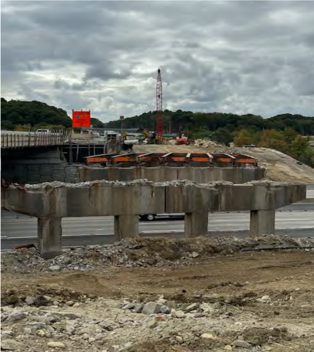
495 South over I-90 during demolition in September 2024
