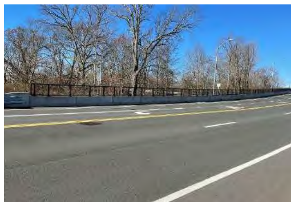
Snow fence complete at Wall #10 November 2024
