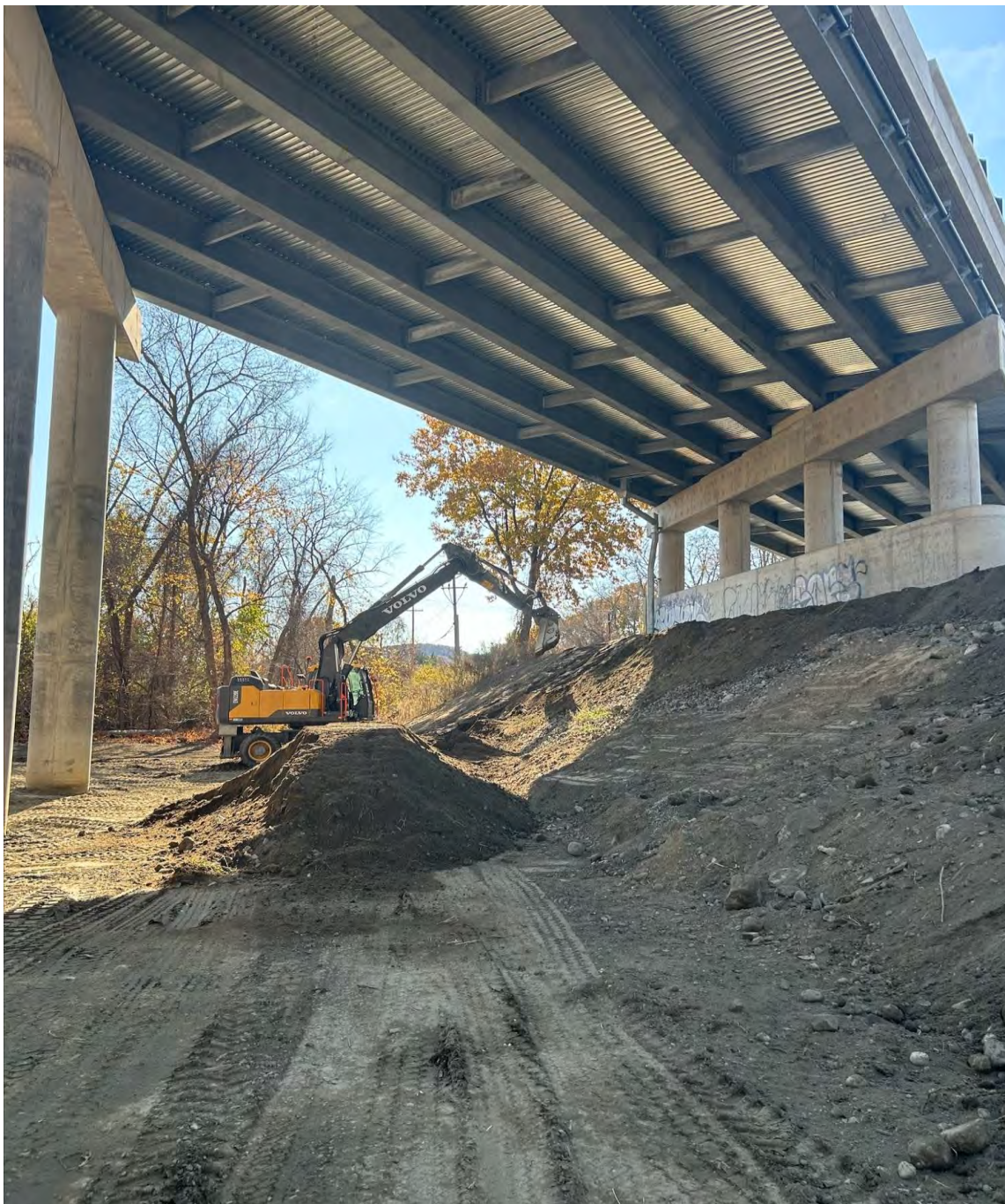
Shaping Slopes Under Bridge No. 59
