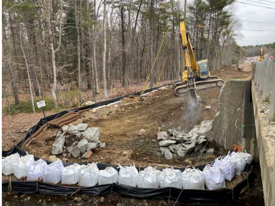
Wingwall Demolition Little River Bridge Stage I
