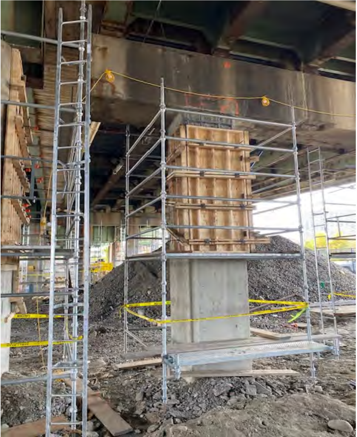
Column repair with lower repaired and upper formed
