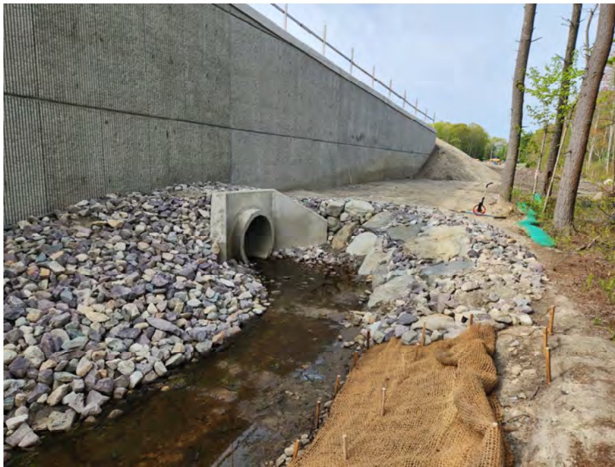
Streambed Relocation Behind Wall 5
