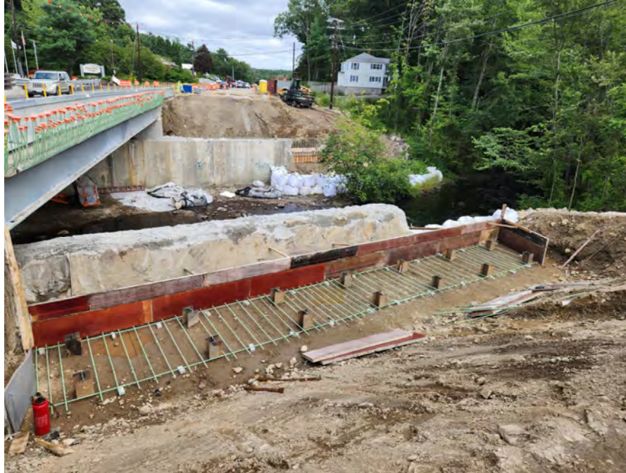
Abutment Footing Formwork French River Bridge Stage 2
