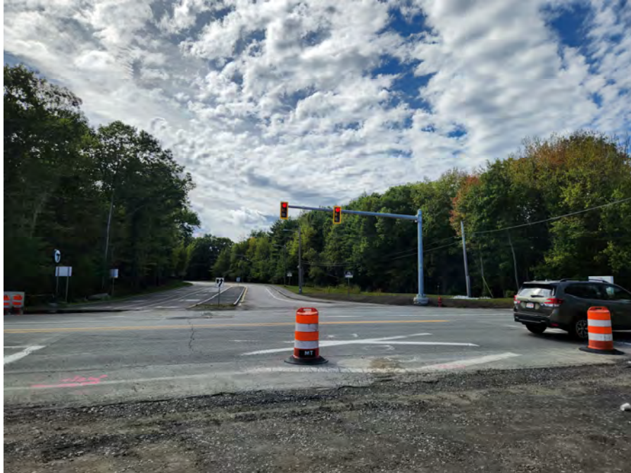
Traffic Signal Installed at Ramp F/Industrial Drive/Route 140 Intersection
