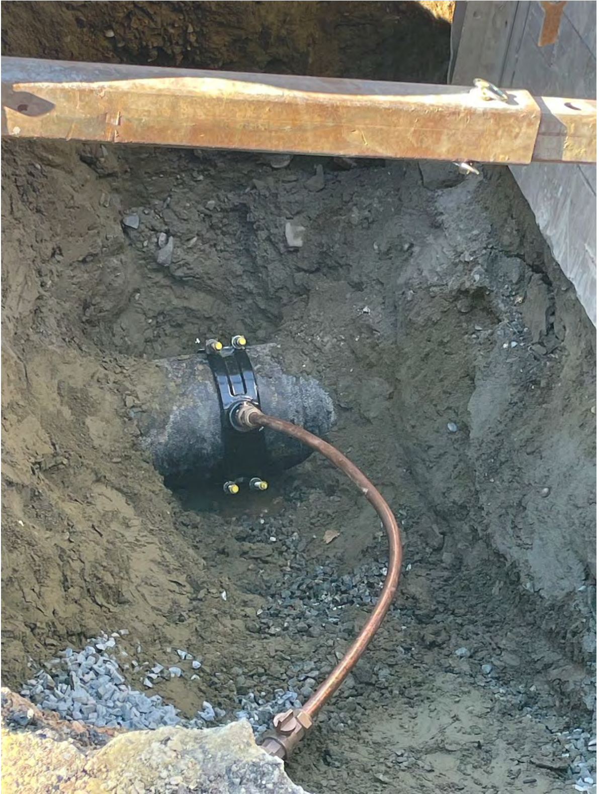
New Service Connection
