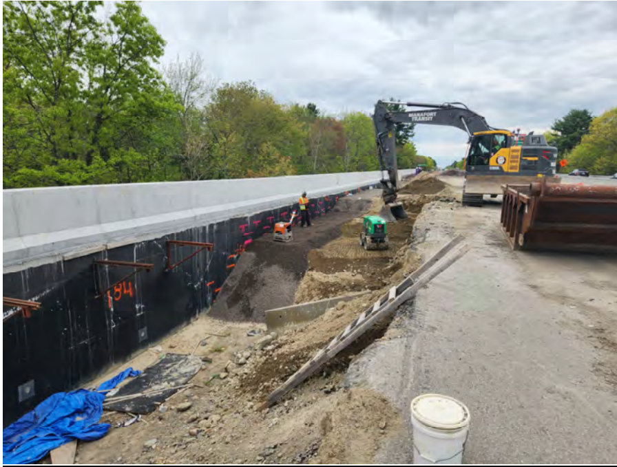
Placement of Lightweight Fill at Wall 2
