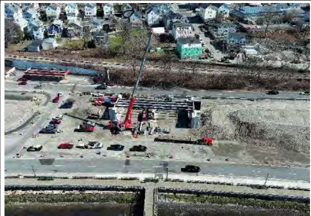
F-02-087 beam erection March 2024
