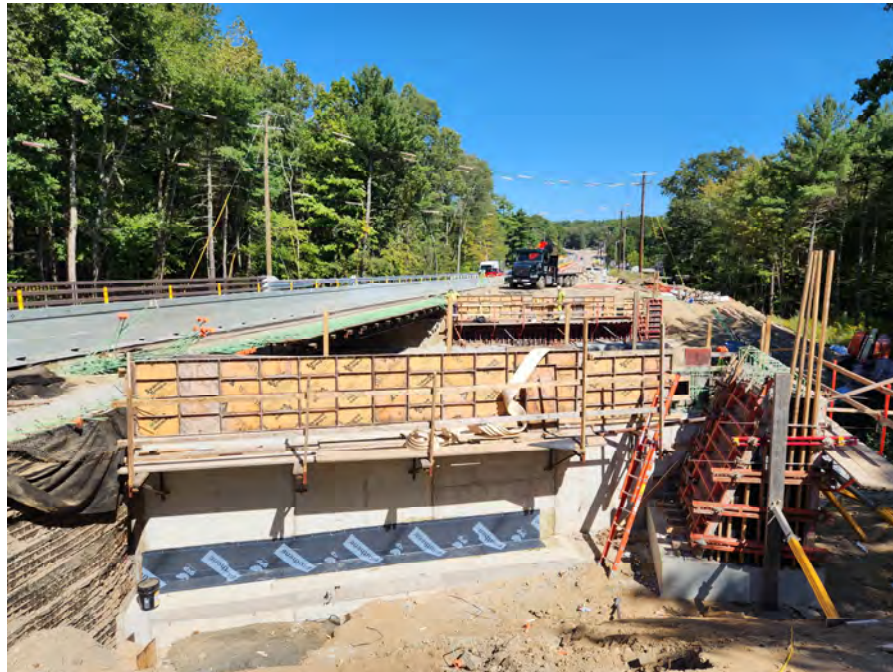
Little River Bridge Abutment and Wingwall Formwork - Stage 2
