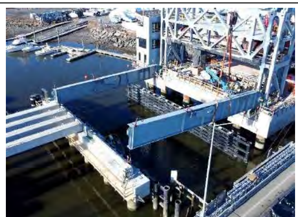
Installation of bascule girders February 2024
