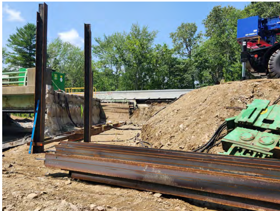
French River Bridge Abutment Demolition and Pile Driving – Stage 2
