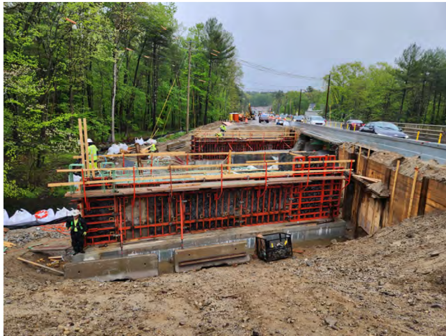
Abutment Formwork Little River Bridge - Stage 1
