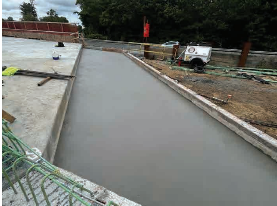
Bridge T-01-047 Approach Slab Concrete Placement
