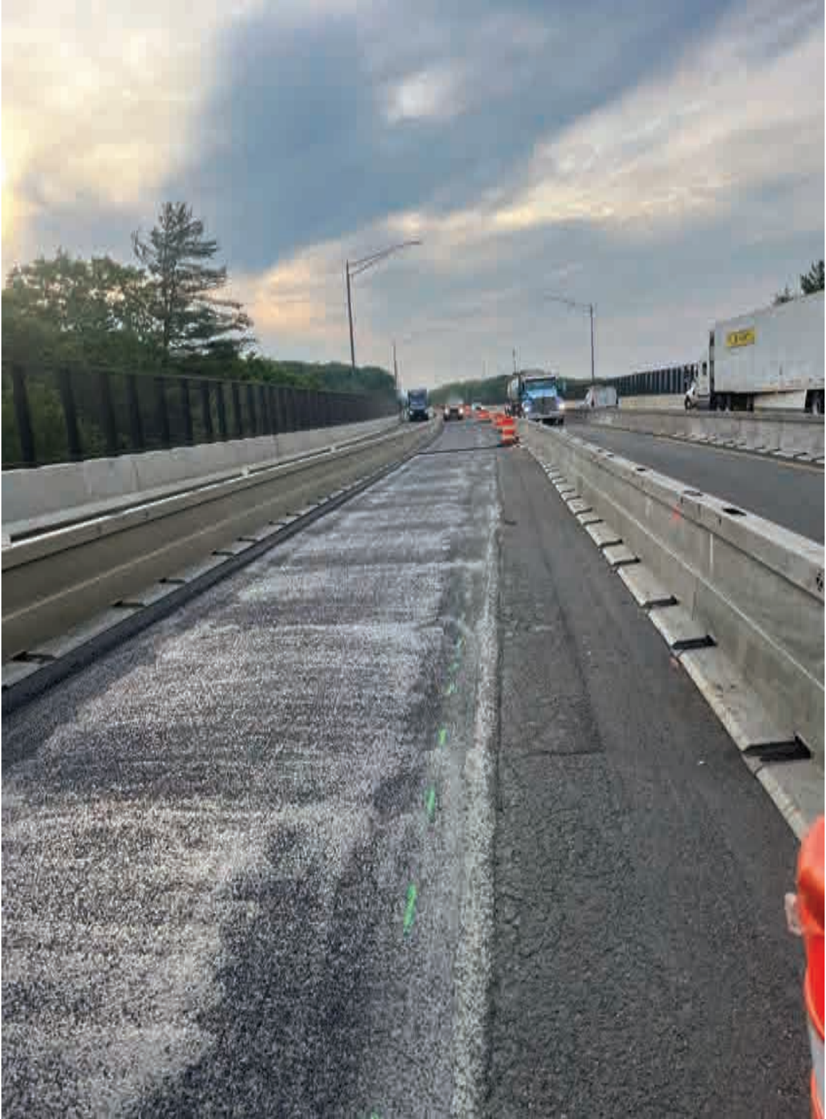
Final Polymer Modified Tack Coat and Membrane Stage V
