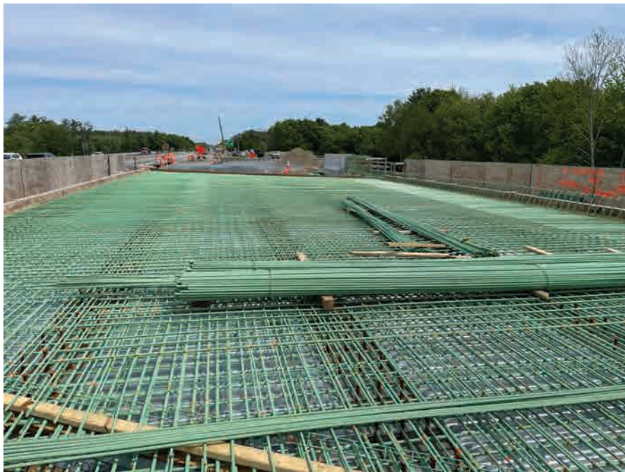
Bridge T-01-046 Deck Reinforcement
