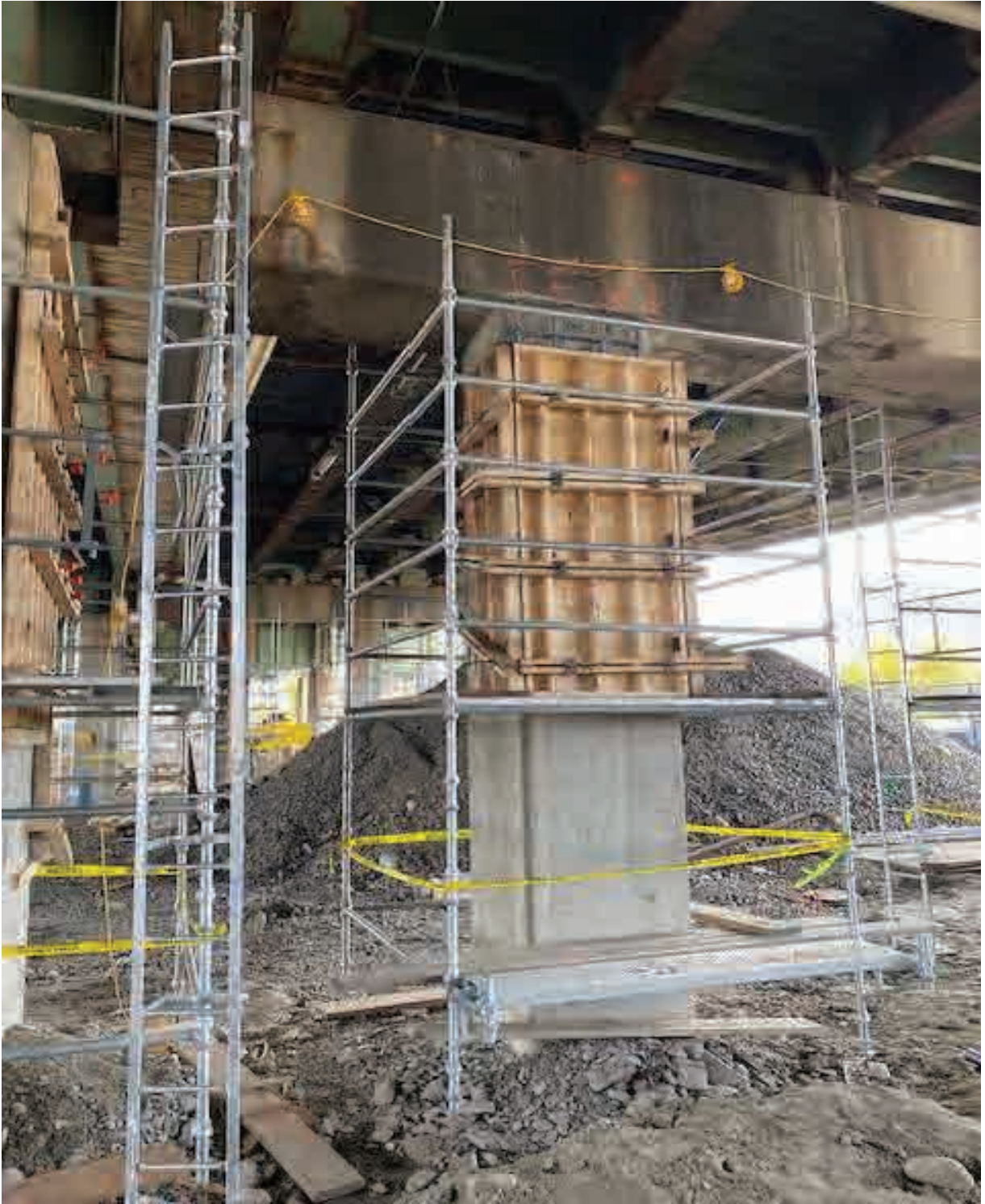
2024 column repair with lower repaired and upper formed
