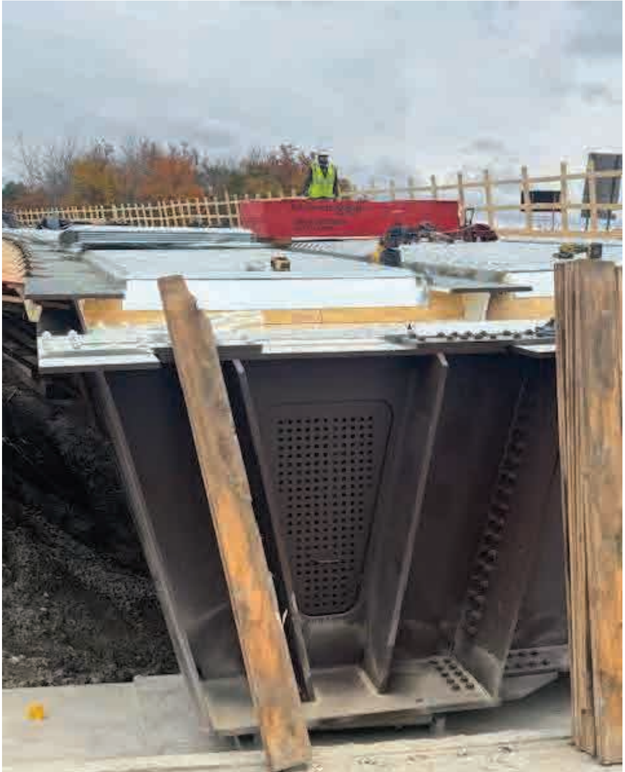
North end of Ramp WN showing end of trapezoidal box beam
