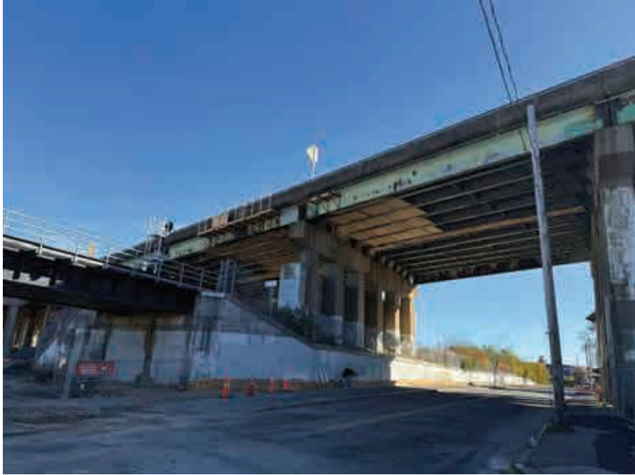
Shielding Installed Over Critical Sidewalks, Roadway, and Railroad Areas – October 2025
