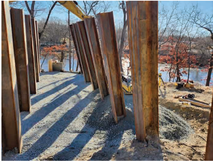
East Abutment Piles (Bridge N-12-066)
