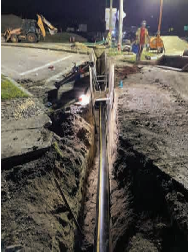
Gas Line Installation in Rt. 9 EB by Eversource
