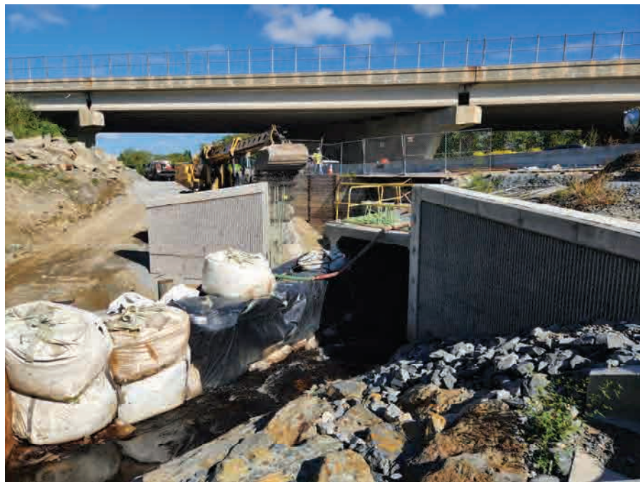
Bridge T-01-054 with Flow Diverted into East Barrel
