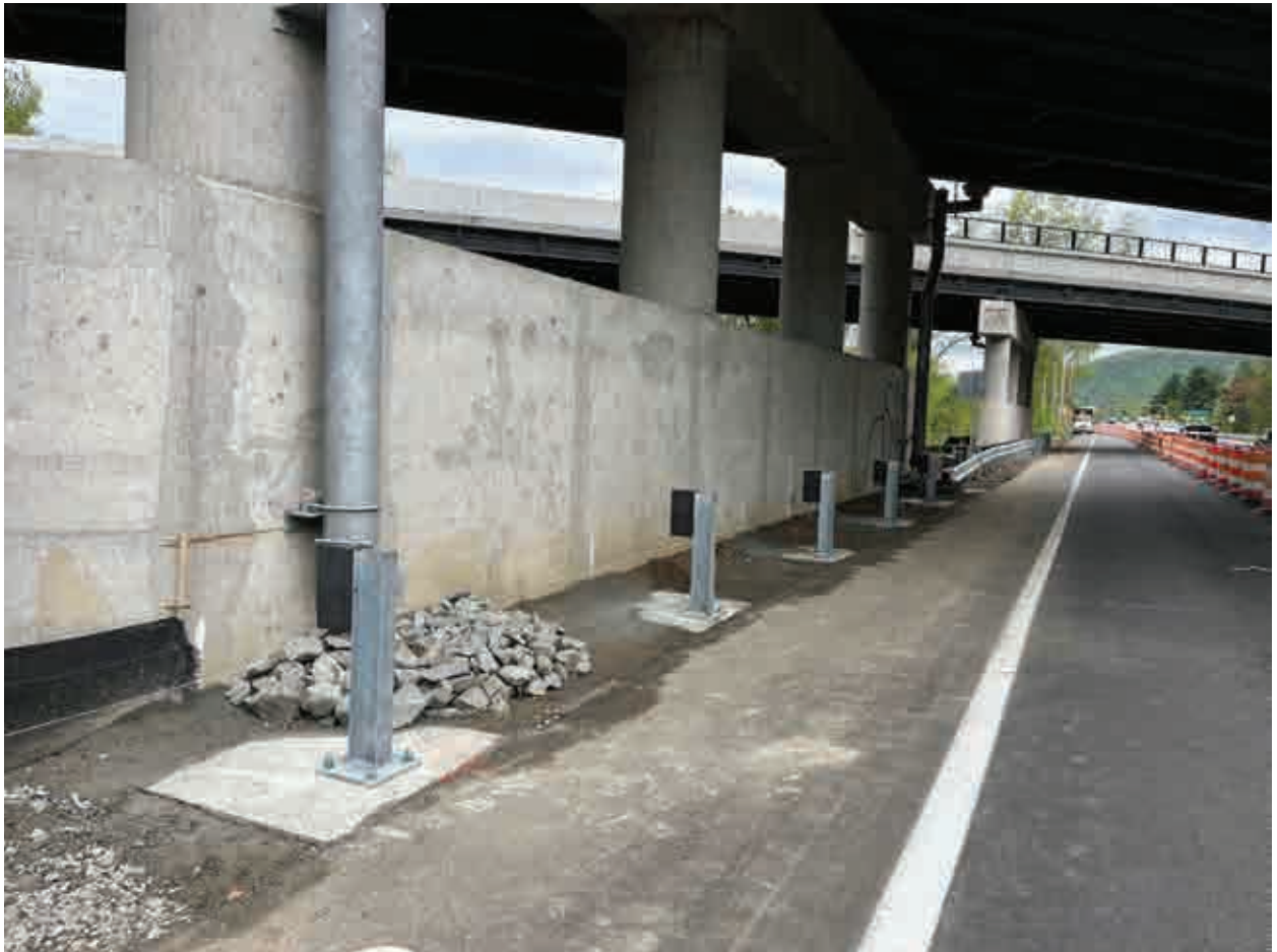
Specialty Guard Rail Foundations and Posts at Pier 2 (Route 5 NB)
