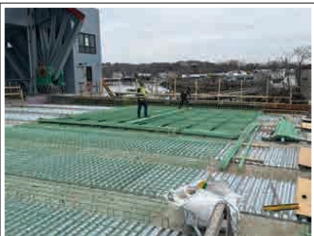
Span 3 reinforcing and SIP pans January 2025
