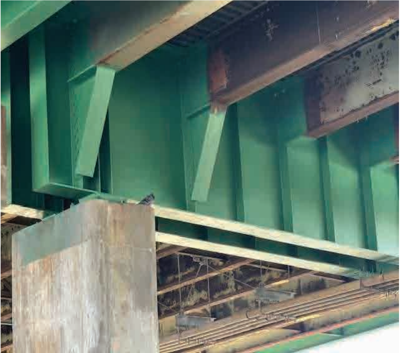
Steel girders at pier post repairs
