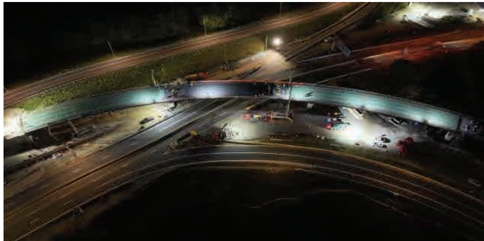
Ramp WS deck placement beginning at night
