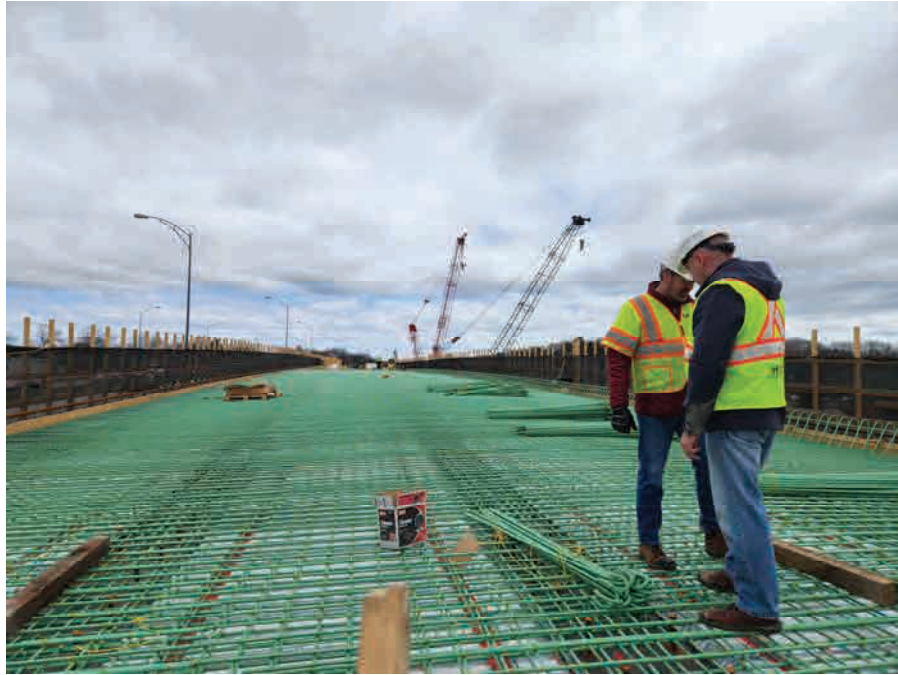
Formwork and Deck Reinforcement (Bridge N-12-066)
