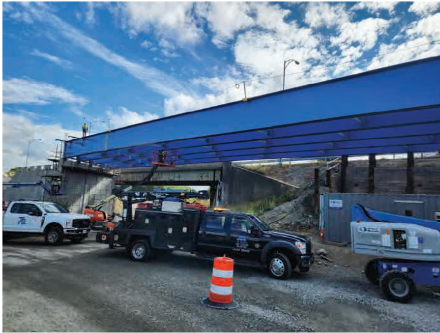
Girders Installed at Bridge W-29-057
