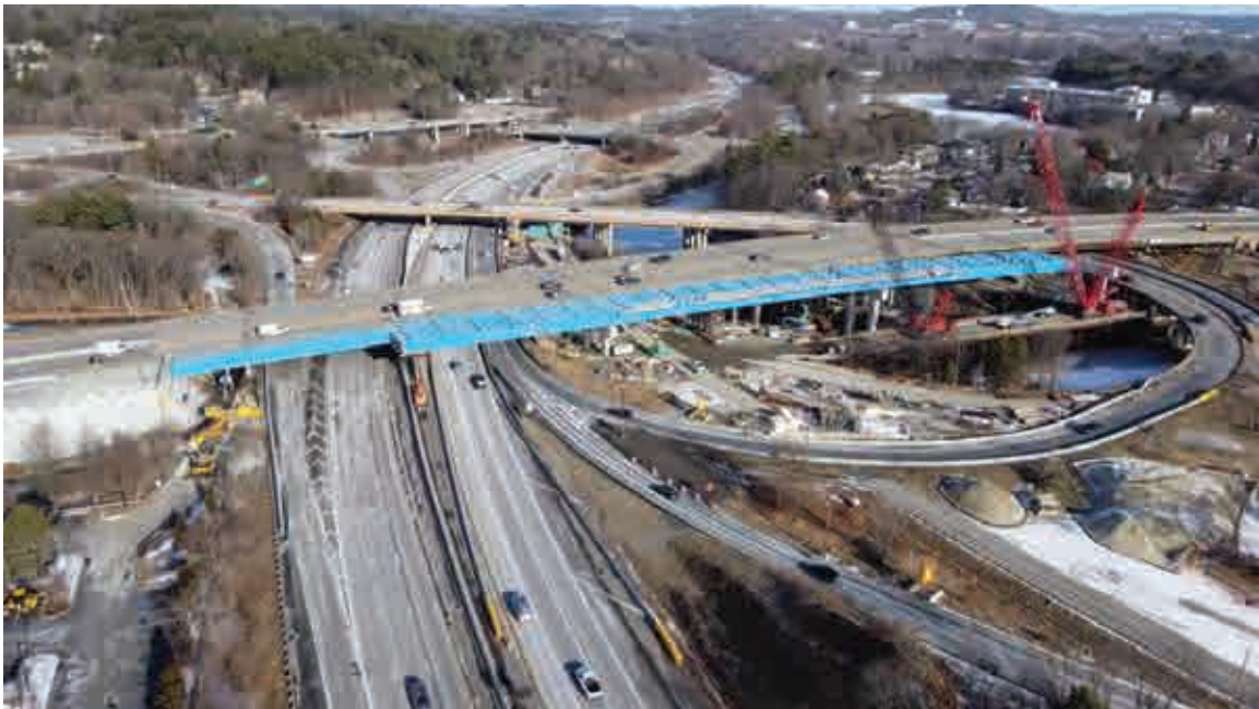
Girder Installation across I-95 (Bridge N-12-066)
