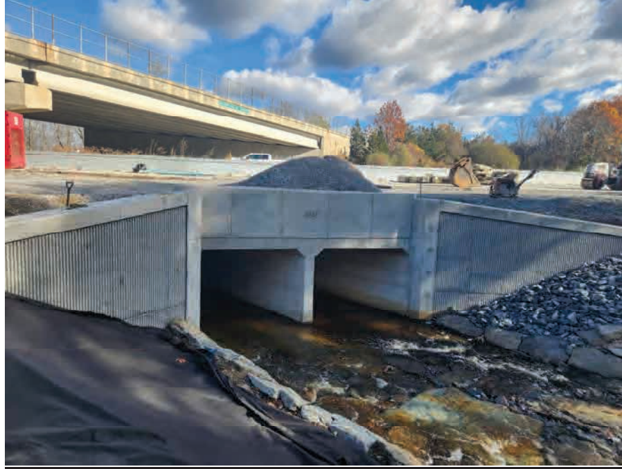
Bridge T-01-054 Extension Completed and Flows through Barrels
