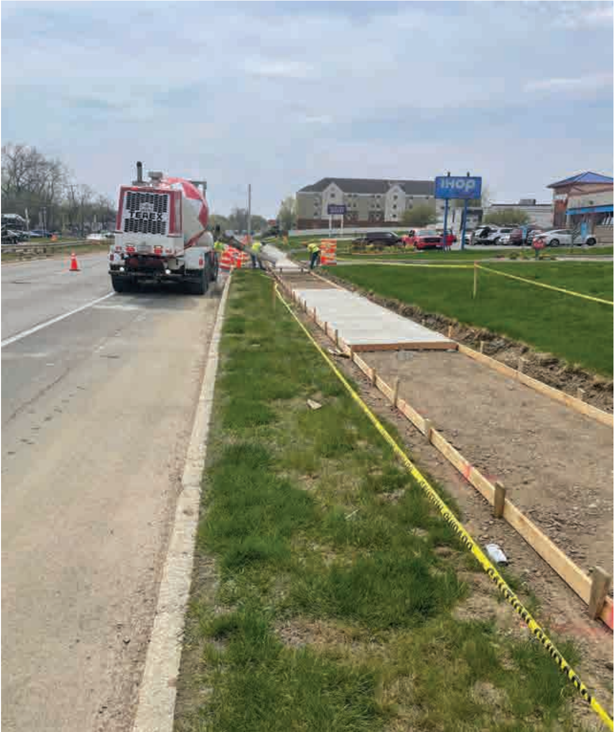
Placing Cement Concrete Sidewalk at Southern End of Project
