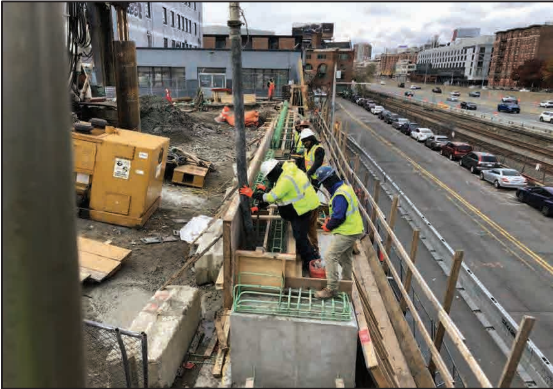
Charlesgate West Bridge South Abutment Backwall Concrete Placement November 12, 2025
