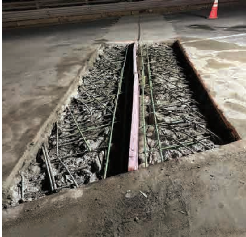
Emergency Deck Repairs
