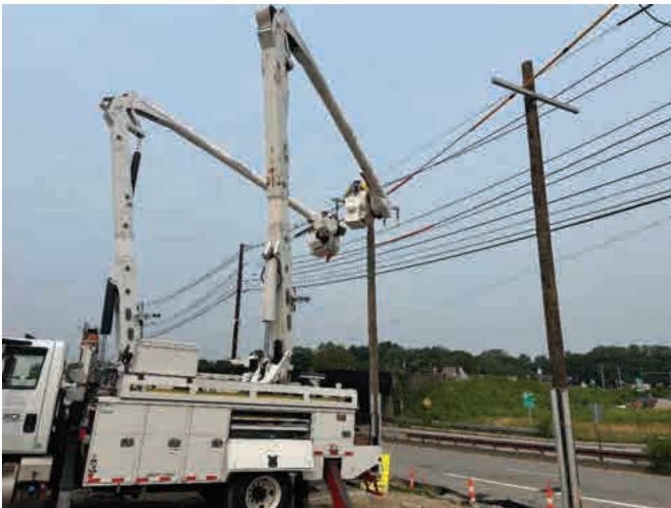
Wiring at New Utility Poles
