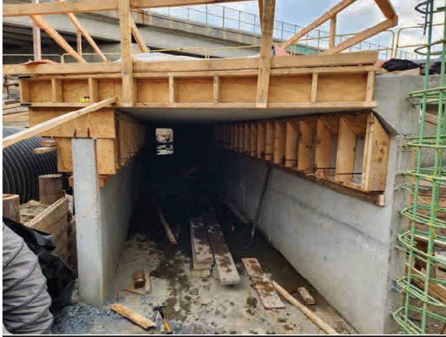
Bridge T-01-054 Roof Formwork
