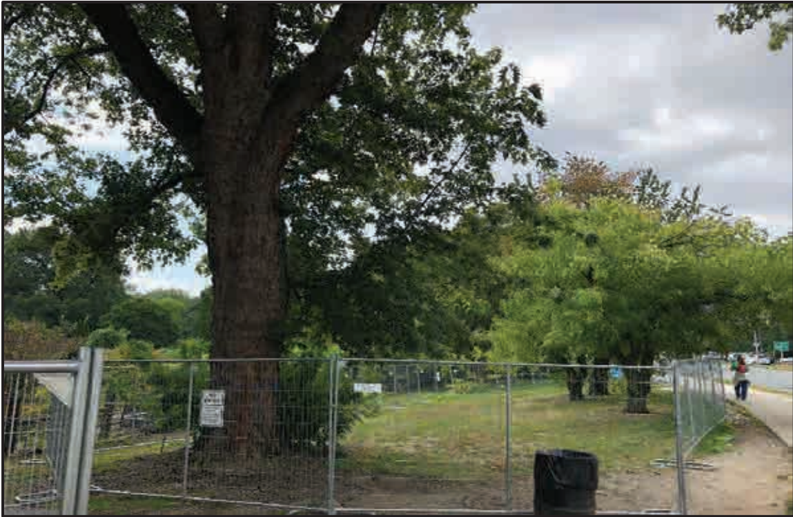
Tree Protection Fencing – September 15, 2025
