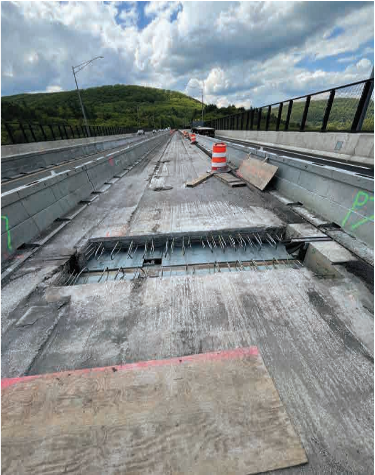
Full Depth Excavation at Expansion Joint – Stage 5 Construction
