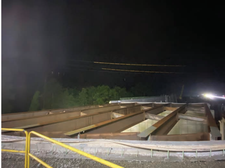
Beam Erection at Bridge T-01-047
