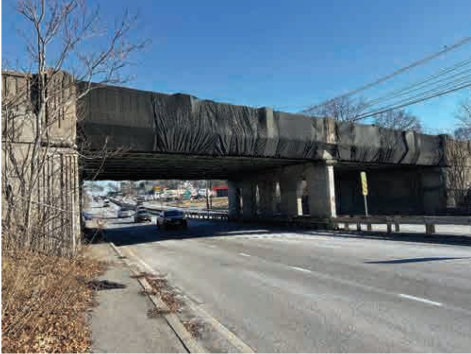
Protective Netting Installed on Existing Rt. 27 Bridge
