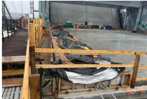
Span 3 east side sidewalk cure from Lynn abutment April 2025
