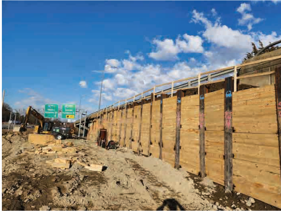
Support of Excavation along Ramp G
