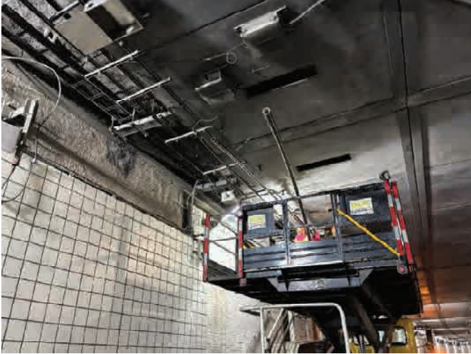
Figure 3 Showing Contractor installing lighting conduits
