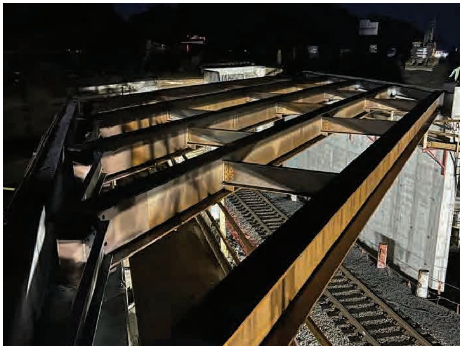
Bridge T-01-045 Beam Erection
