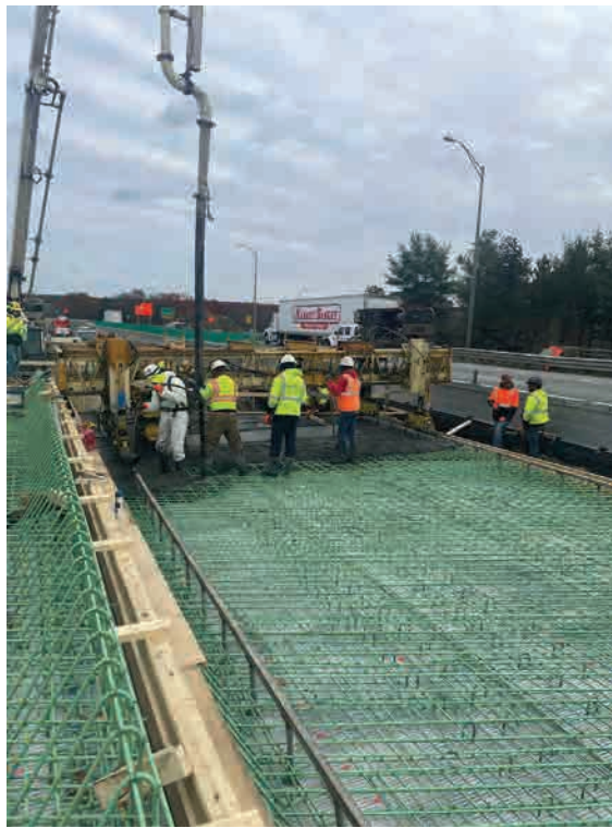
Placing Concrete for Bridge Deck
