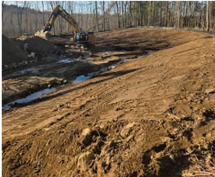
Building Subgrade at Wetland Replication Area
