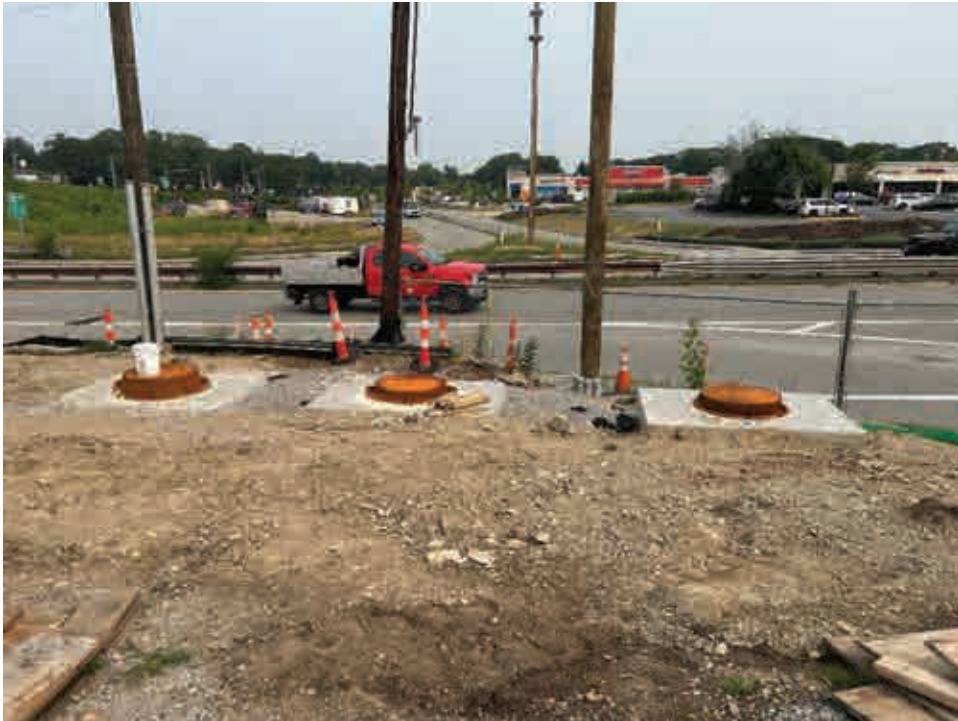
Duct Bank Manholes Installed at South Abutment
