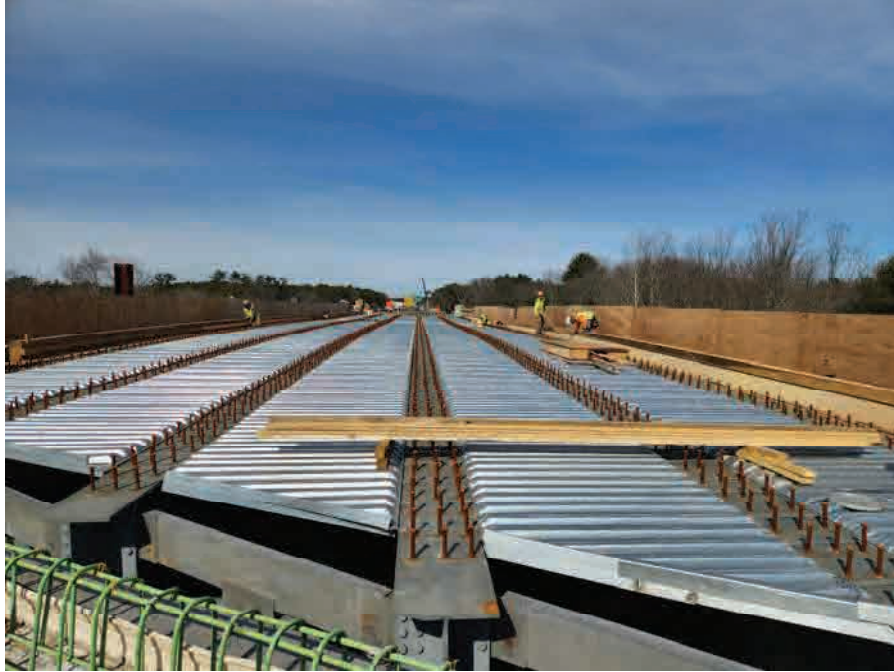
Bridge T-01-046 Deck Formwork
