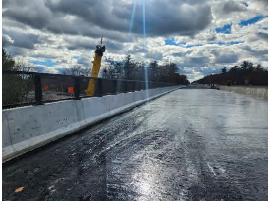
Bridge T-01-046 Membrane Waterproofing and Snow Fence
