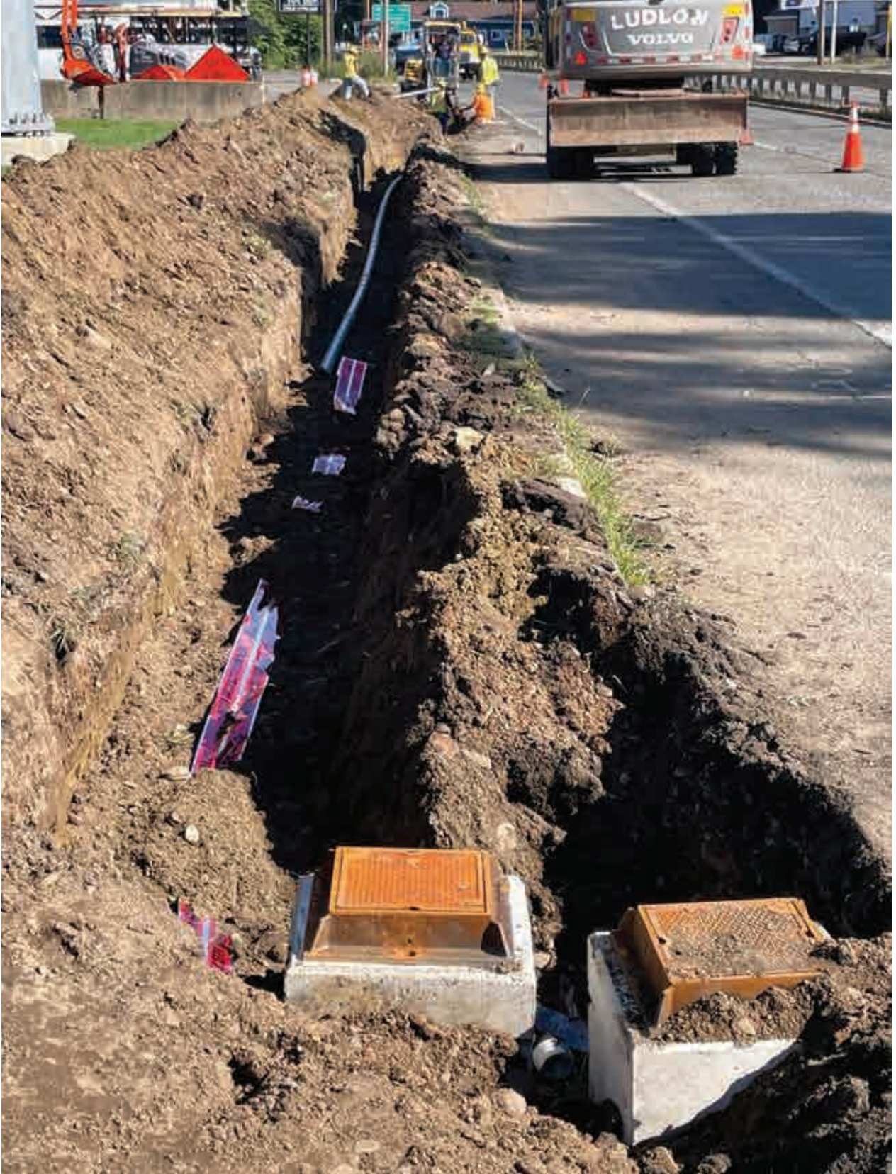
Conduit Installation for Traffic Signal
