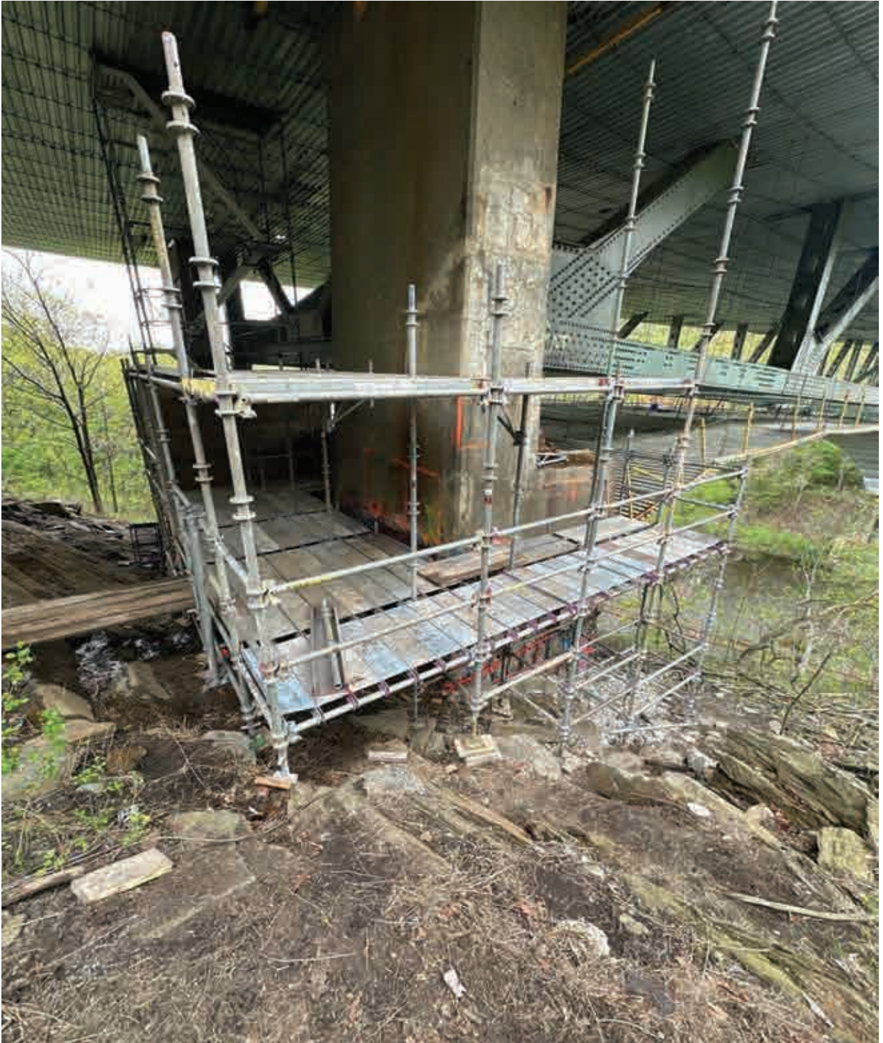
Staging for Pier 7 Spalled Concrete Substructure Repair
