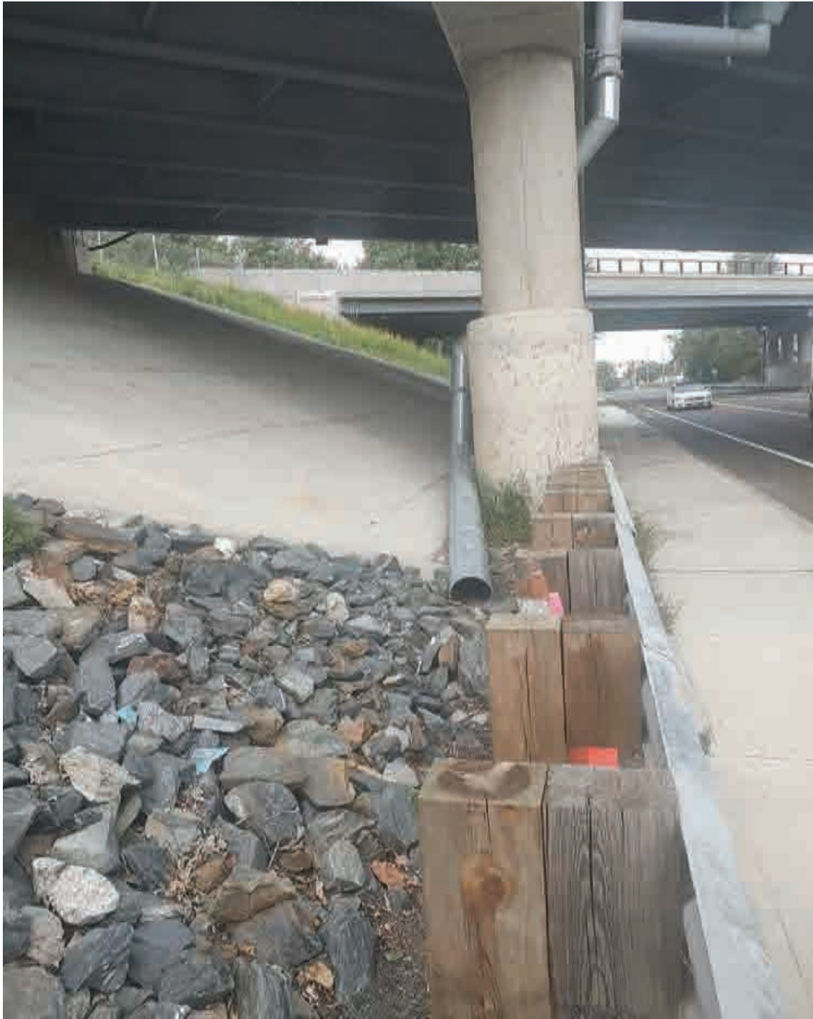
Re-worked Downspout at Pier 1 Emptying Behind Sidewalk and Guard Rail
