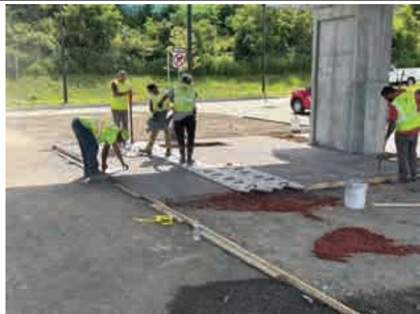
Stamped concrete sidewalk under F-02-087 August 2025
