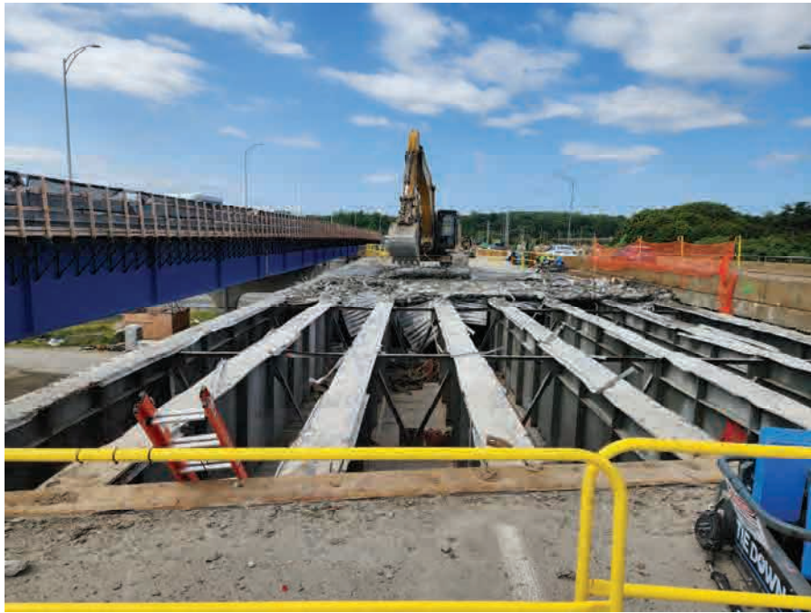
Demolition of Existing Eastbound Bridge N-12-066 Superstructure
