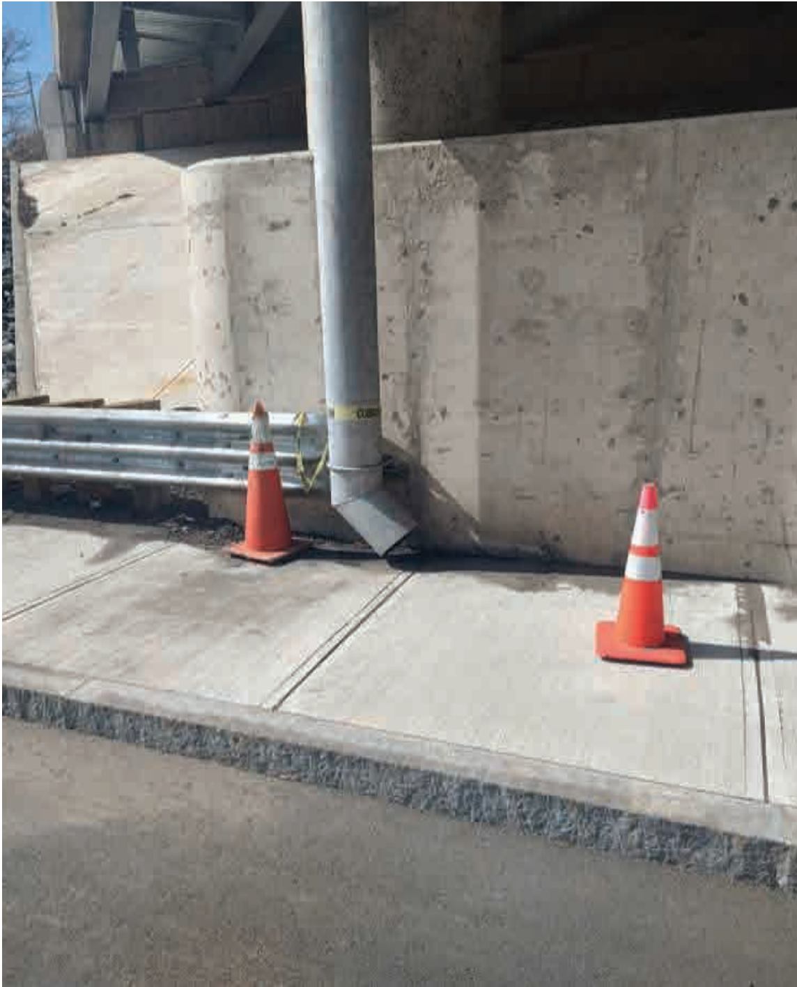
Prior Condition-Downspout at Pier 1 Emptying Onto Sidewalk
