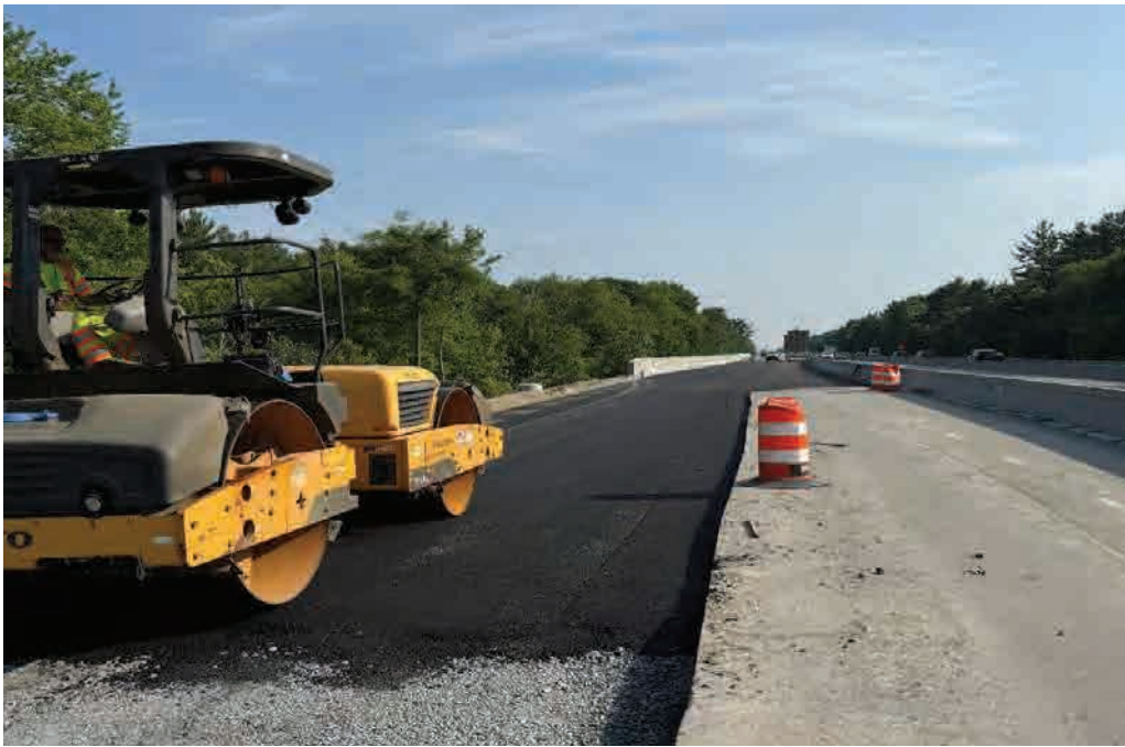
Paving Roadway Widening on Route 24 North
