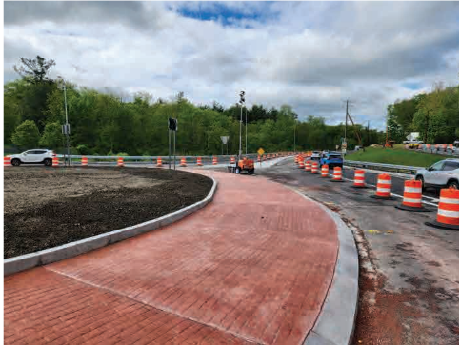
Roundabout Truck Apron Construction
