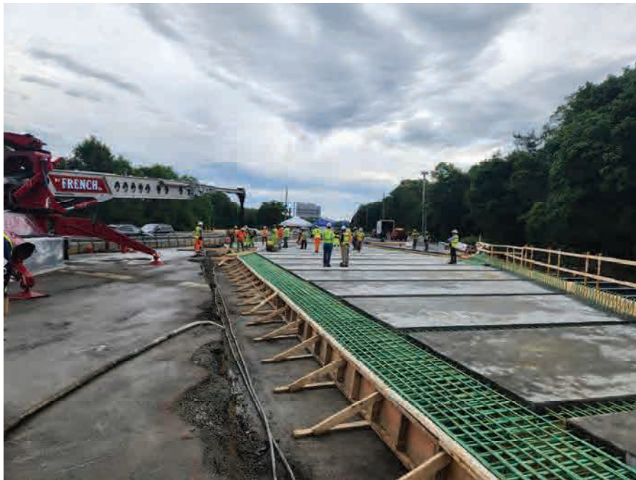
Weekend Two Precast Bridge Units (Bridge N-12-067)
