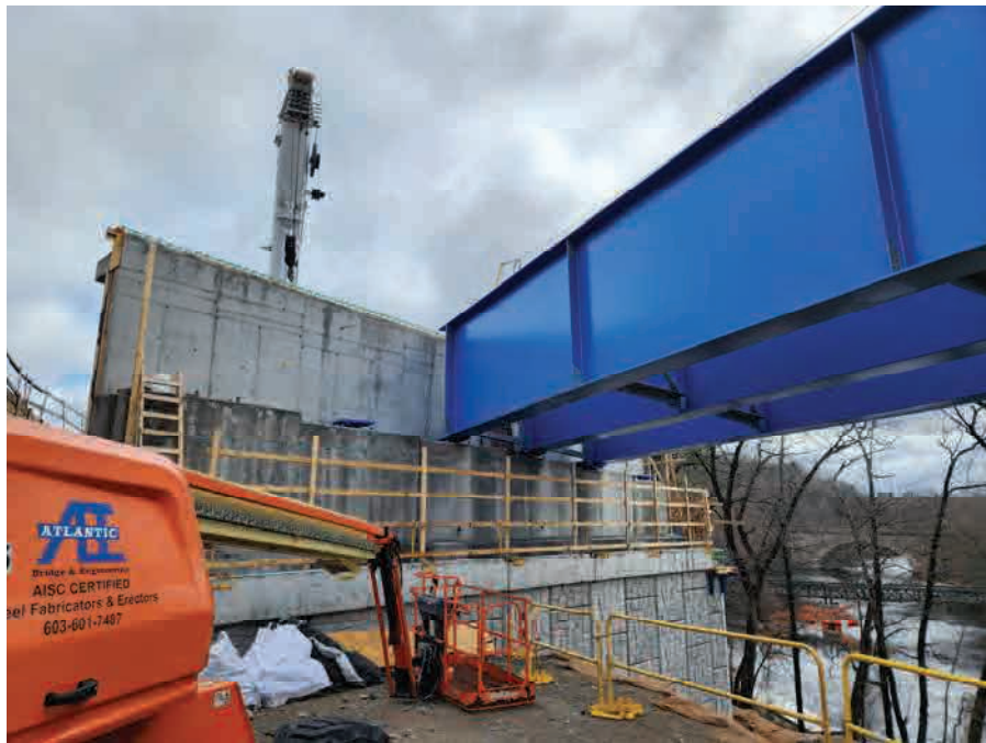
Girder Installation at East Abutment (Bridge N-12-066)
