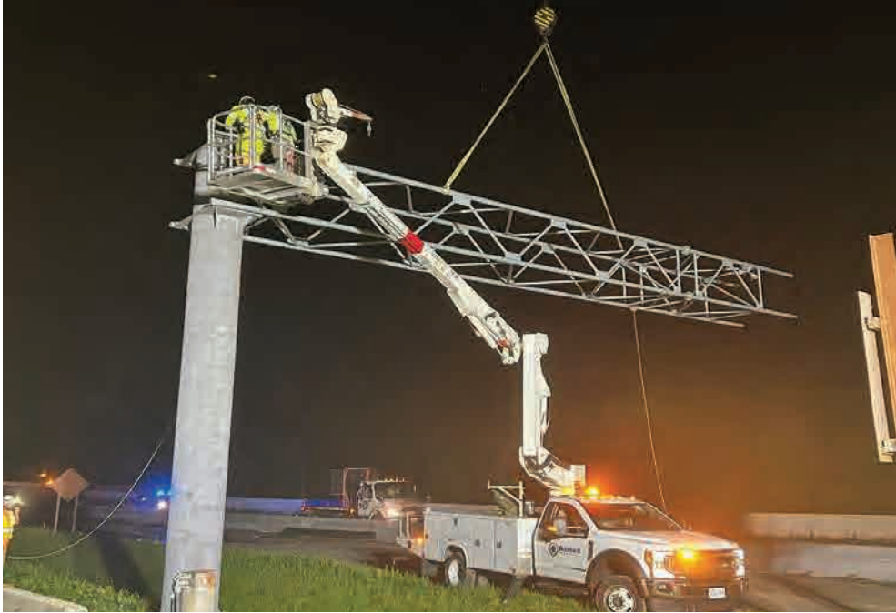
Overhead Sign Installation on Route 140
