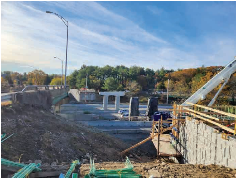
Bridge W-29-055 Abutment and Pier Construction
