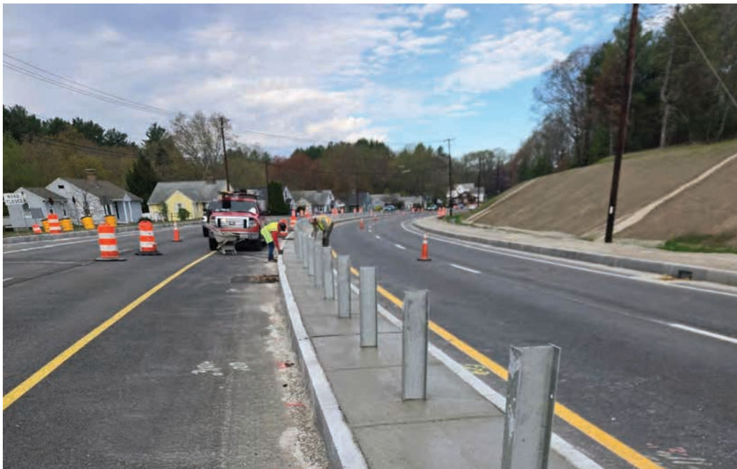
Raised Median Construction
