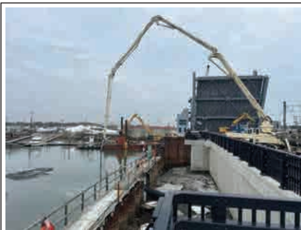
Placement of concrete ballast blocks on 20" MWRA water main January 2025
