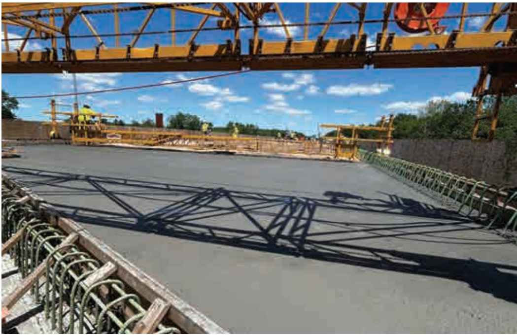
Bridge T-01-046 Concrete Deck Placement
