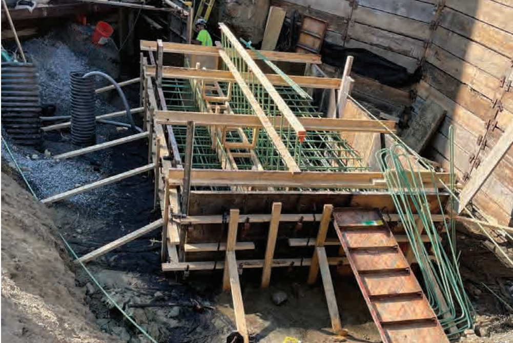
Bridge T-01-054 North Extension Wingwall Footing
