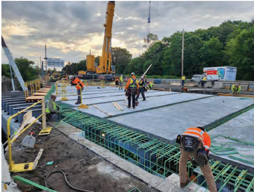
Weekend One Installation of Precast Bridge Units (N-12-067)
