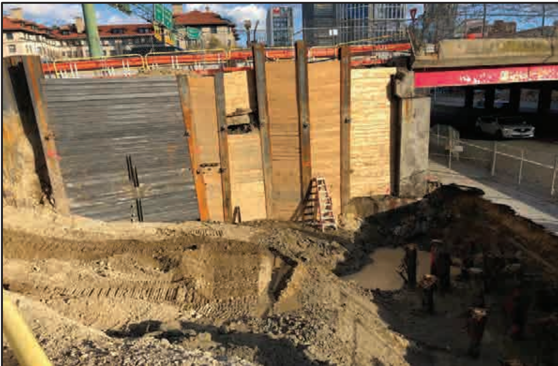
Charlesgate West North Support of Excavation and Timber Piles – November 24, 2025
