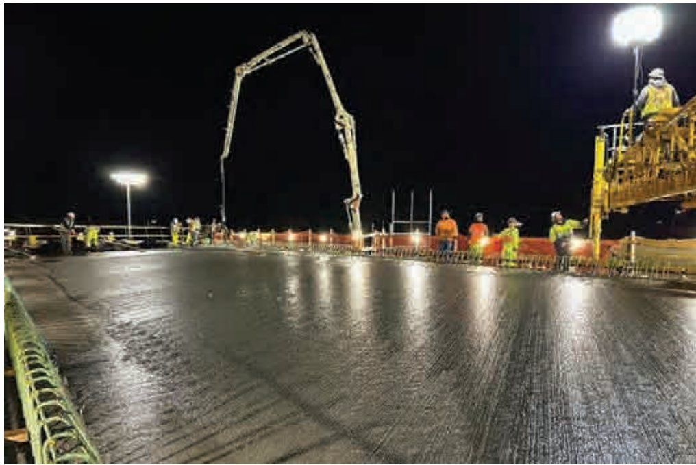
W-29-057 Deck Concrete Placement
