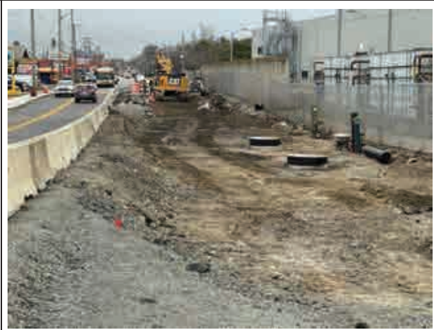
Looking north: full depth roadway reconstruction Rt. 107 northbound in Lynn December 2025
