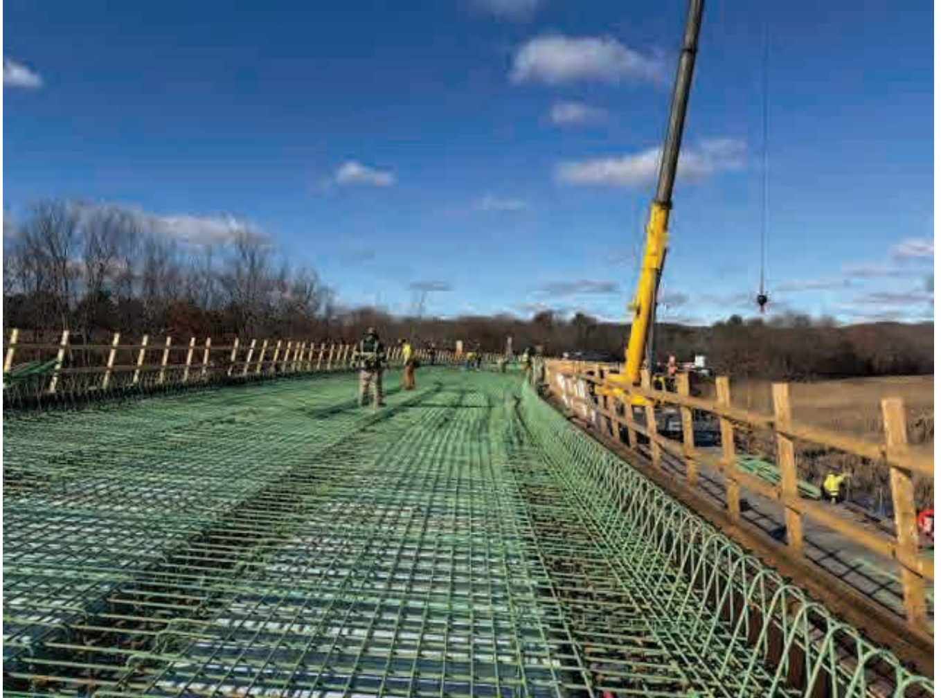
Ramp WN with deck pans and studs installed and now rebar being placed
