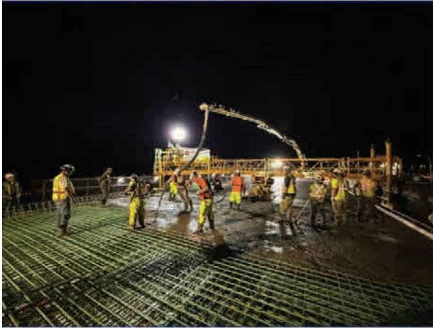
Deck Concrete Placement (N-12-066)
