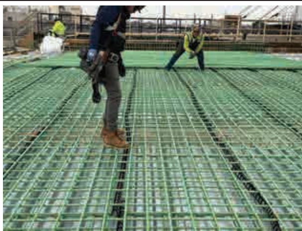
Span 3 reinforcing steel detail January 2025
