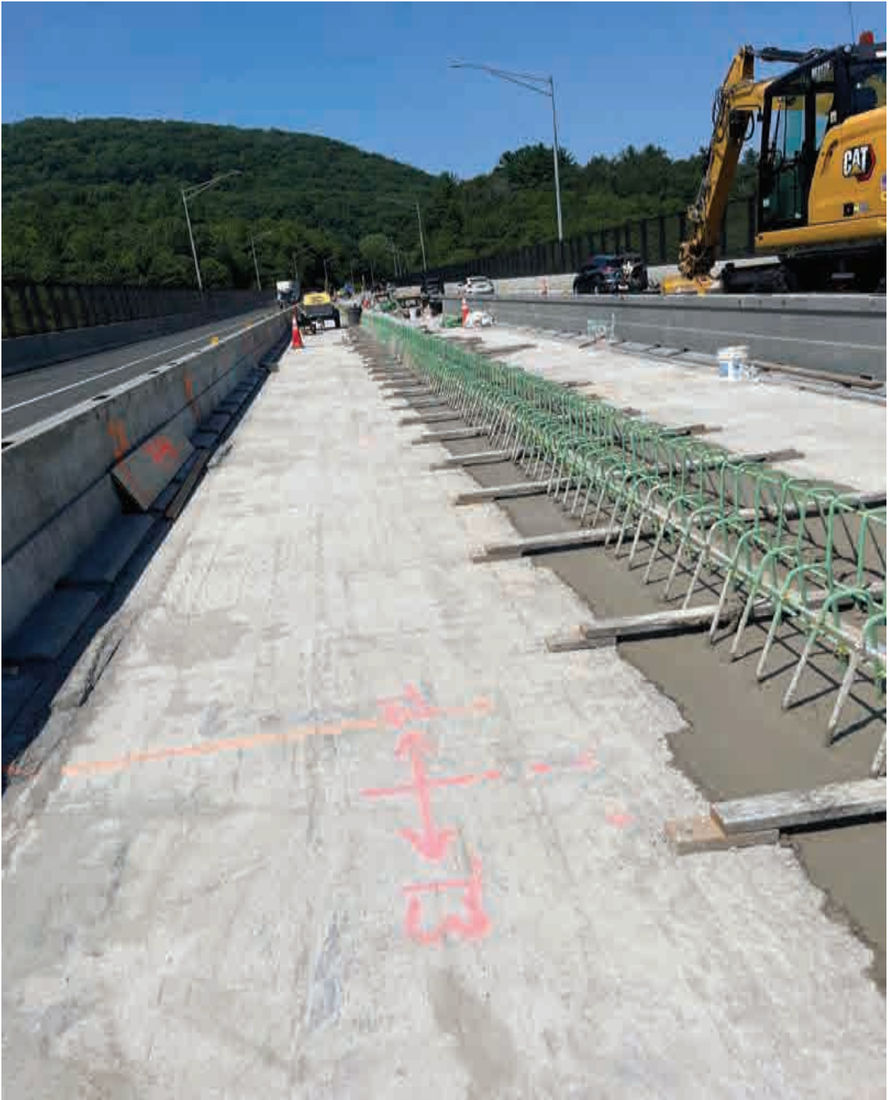
Placed Concrete at Center Median Barriers Stage VI
