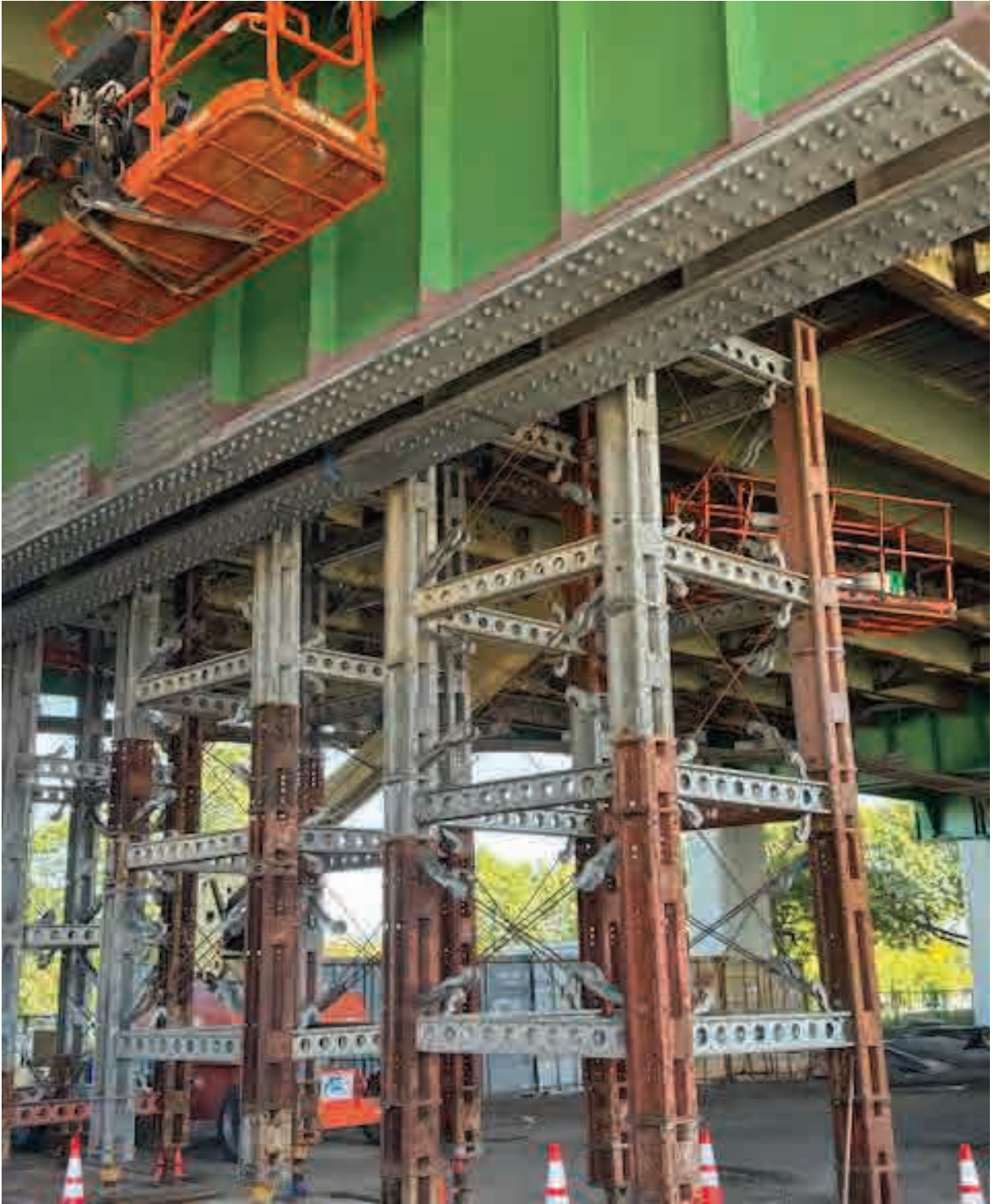
Major steel repairs to girders with temp shoring towers shown
