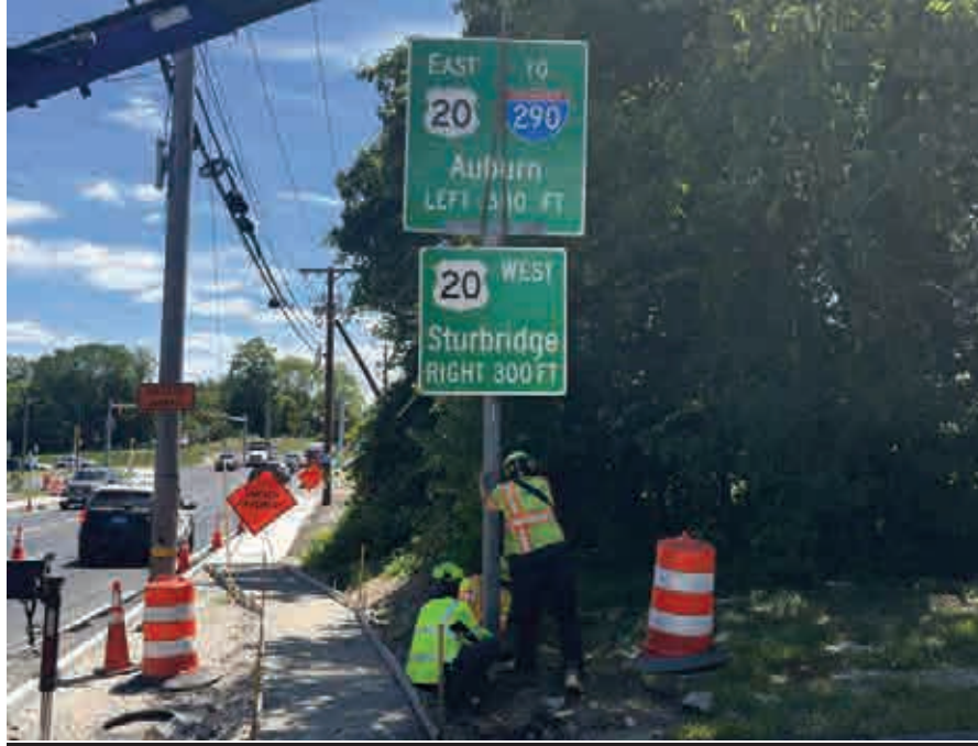
Guide Sign Installation
