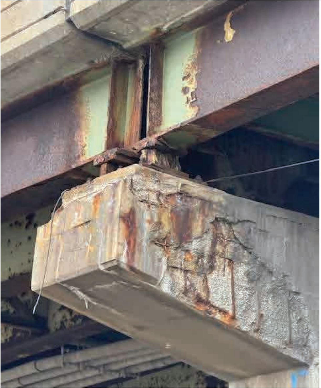
Typical conditions of concrete pier cap and steel beams prior to repairs (2023)
