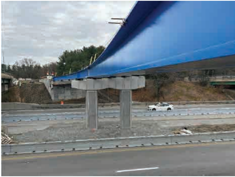
Girders Installed at Bridge W-29-055
