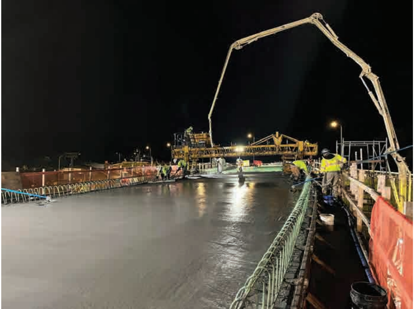
Ramp WS deck placement beginning at night
