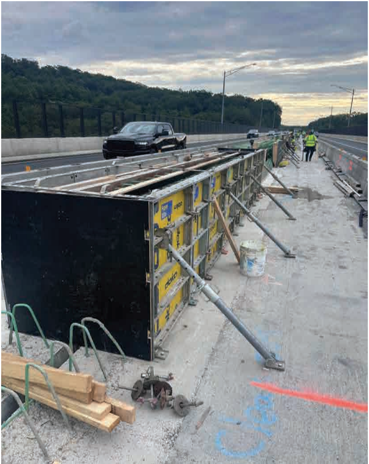
Form Work for Median Barrier Sections
