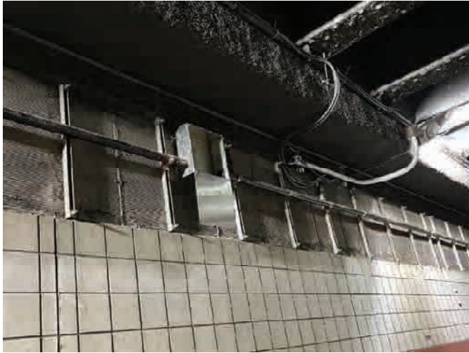
Figure 1 Showing installed lighting conduit and junction box
