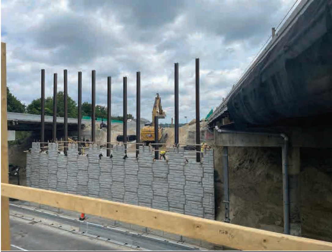
ME Wall Installation at Abutment
