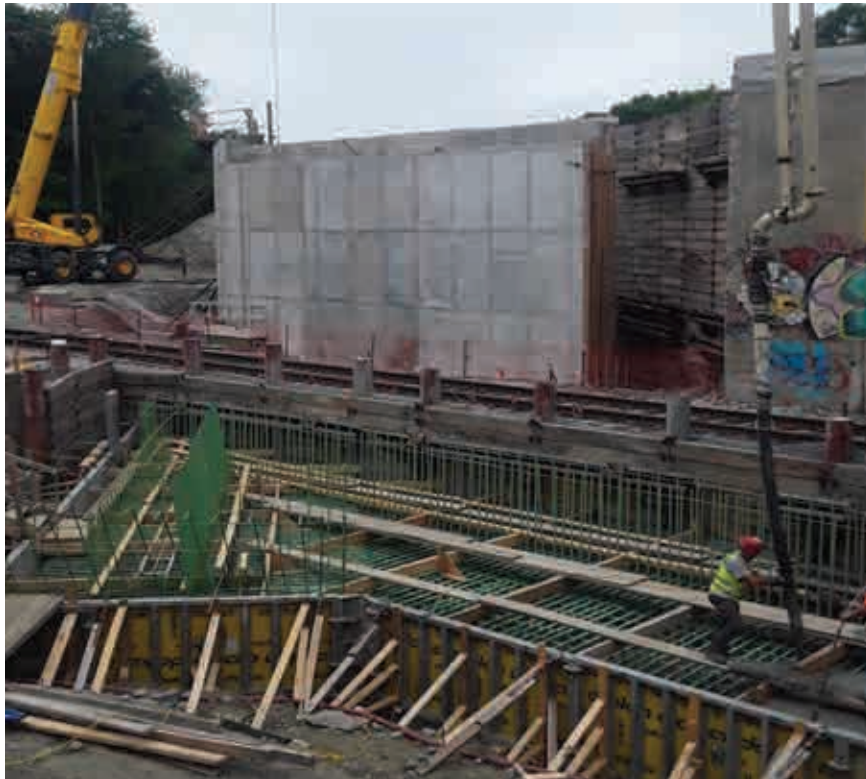
Concrete Placement at Bridge T-01-045 North Abutment Footing
