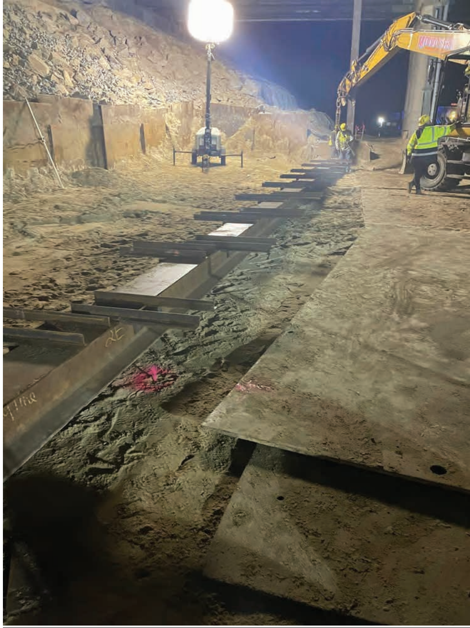
Pile Installation for Integral Abutment
