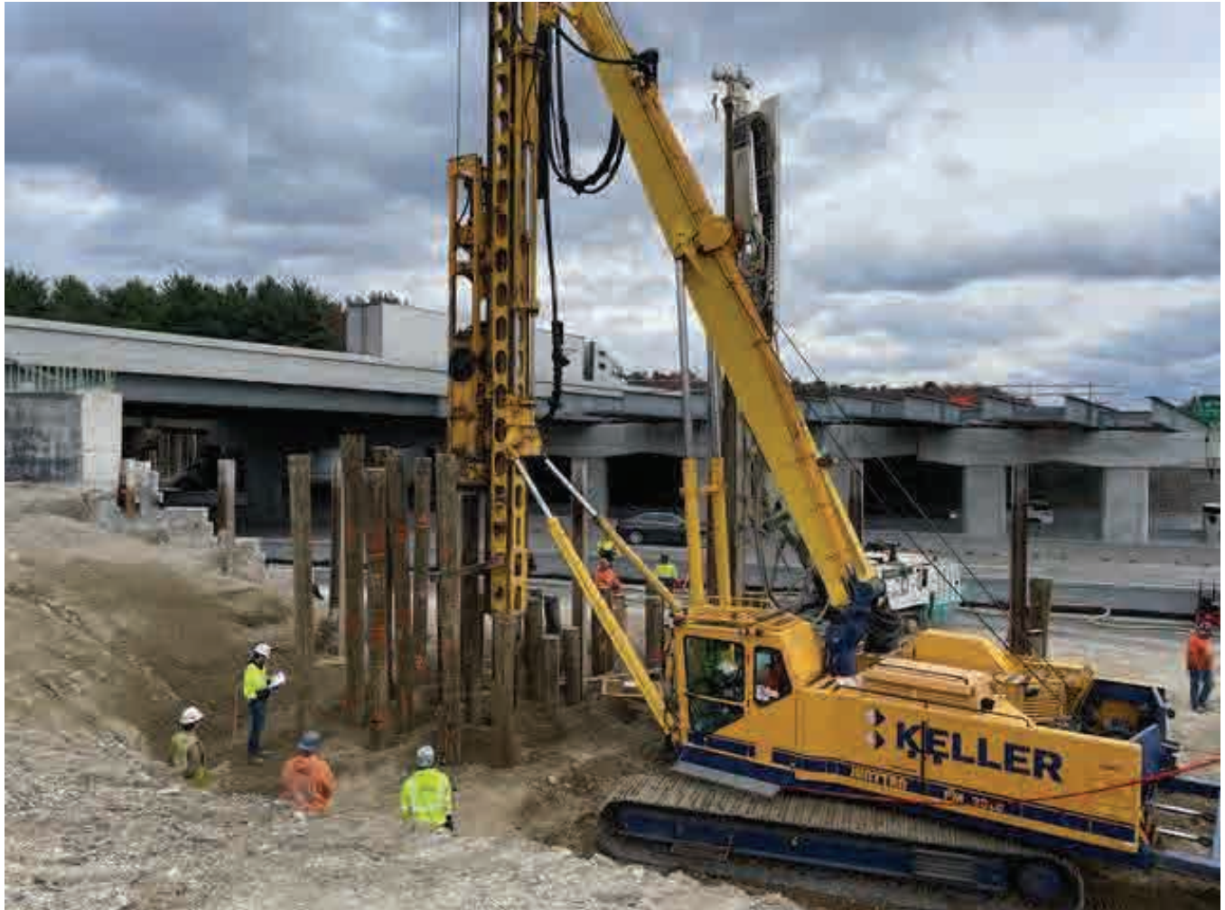
Timber piles being driven to improve ground at I-495 over I-90 north abutment
