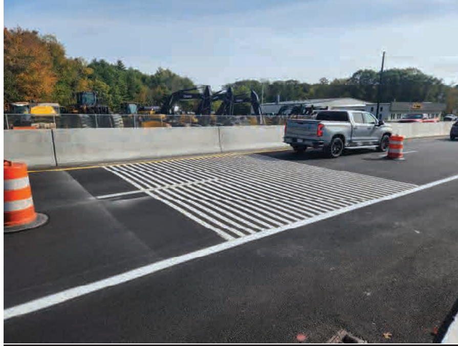
Placement of Approach Warning Strips to the Oxbow Roundabout
