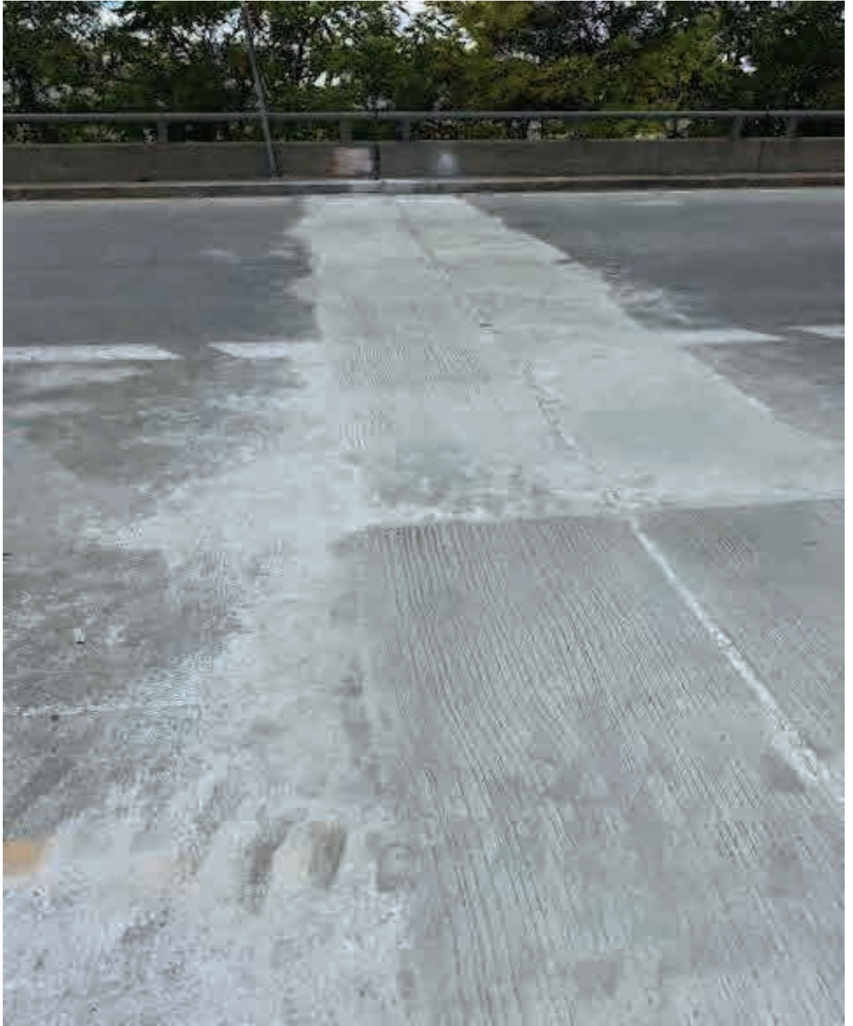
Roadway joint repair completed on Ramp D
