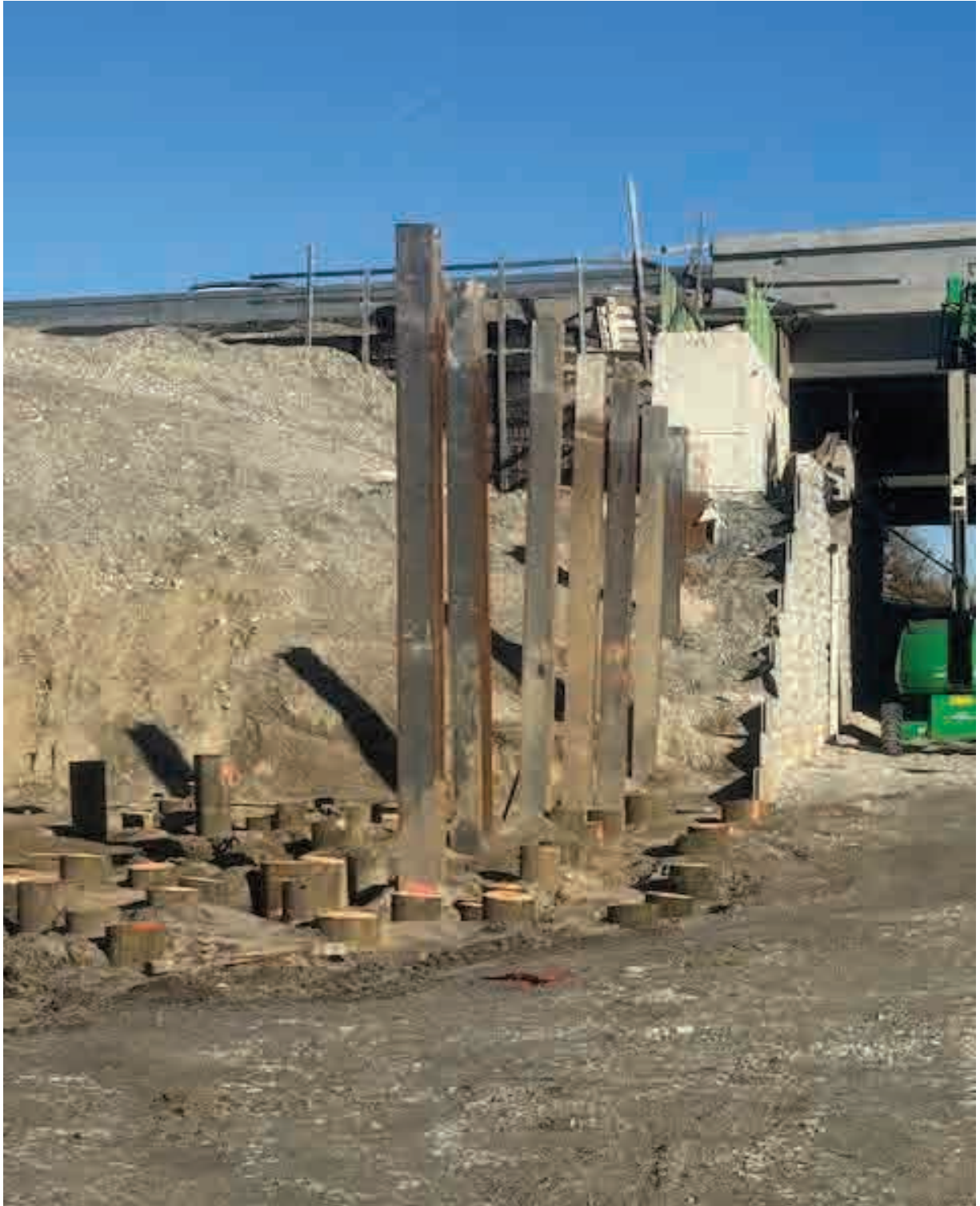
Timber piles completed and cut off at I-495 north abutment
