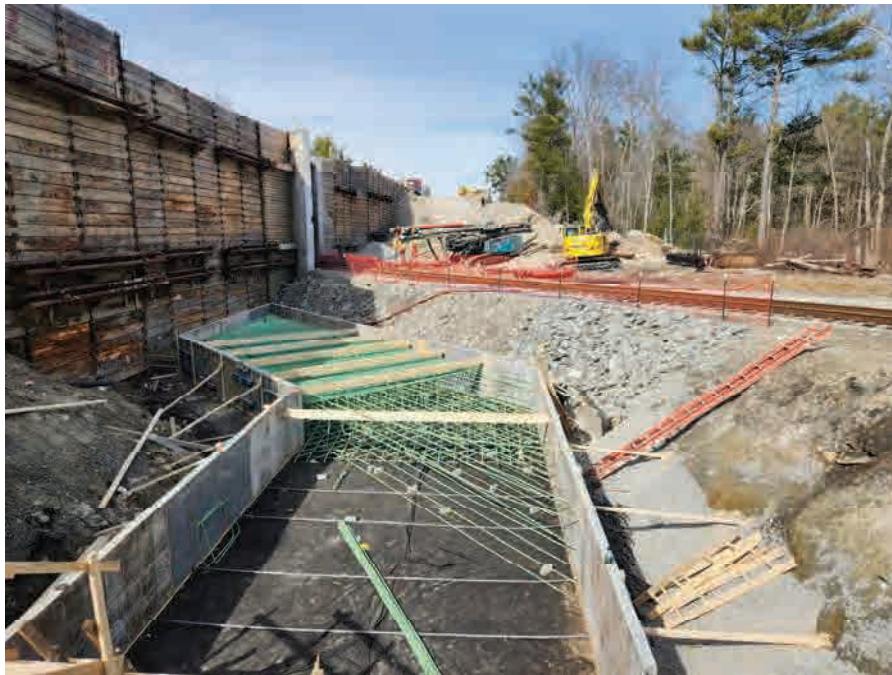
Bridge T-01-045 South Abutment Footing
