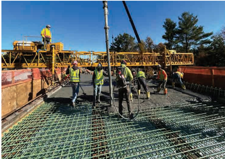
Bridge T-01-045 Concrete Deck Placement
