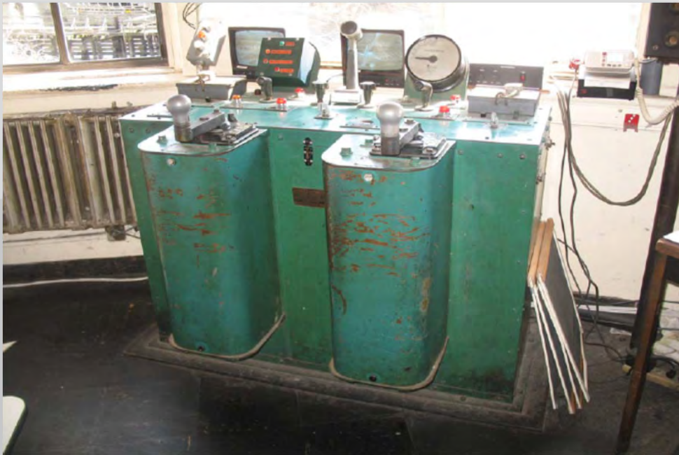
Switching machinery, second floor control room, since moved to current control tower. 2010
