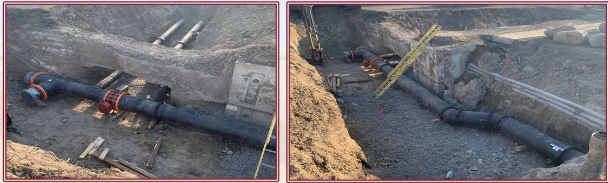
18" diameter HDPE Central Loop
