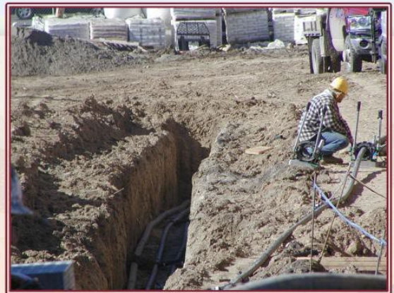
Pipes connecting bore holes
