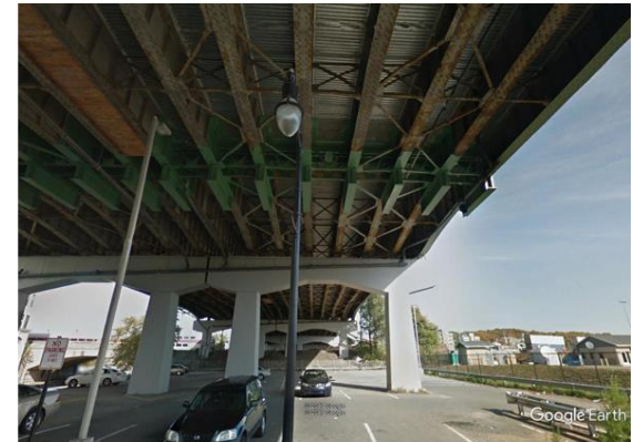
I-290 Viaduct, Worcester | 177ksf
